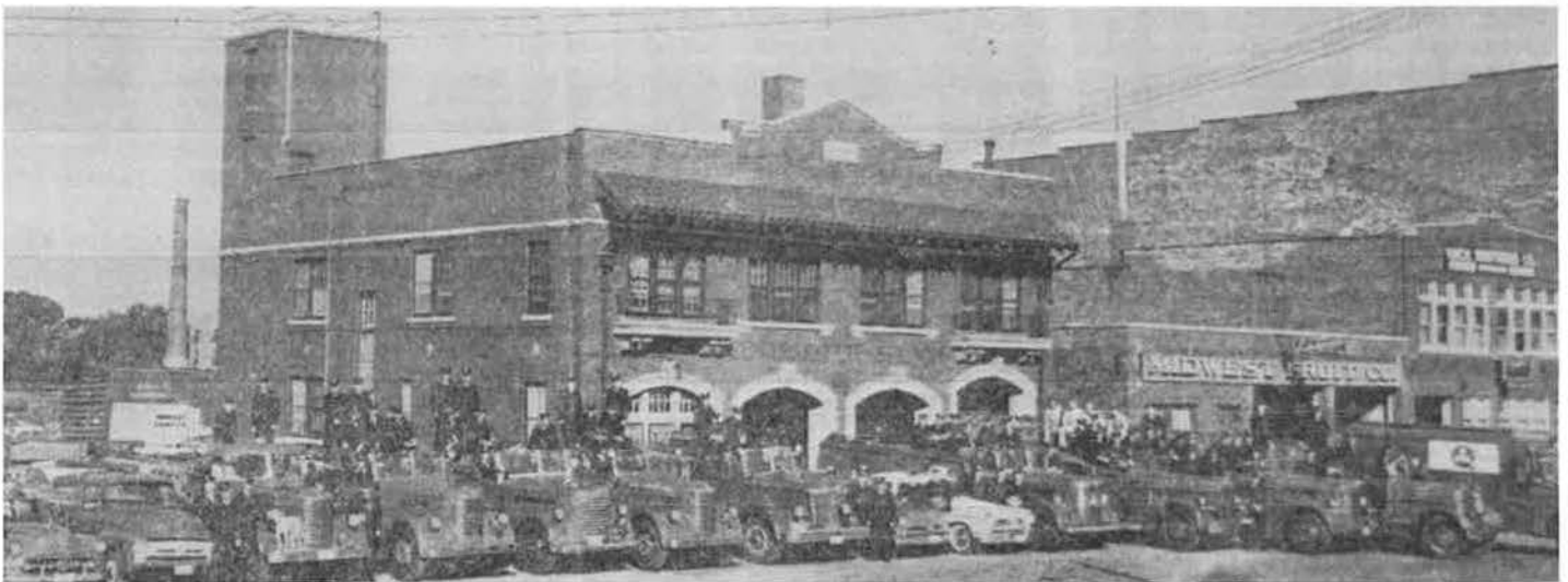
Figure 4 This 1956 photograph clearly shows the addition of a tall tower at the rear corner of the fire station. The projecting structure behind the roof's crown pediment is the station's chimney, which is extant. All of the warehouse buildings seen in this view are extant as well. The tallest stepped wall on the right is the southern wall of the Warfield-Pratt-Howell Company. (Carl & Mary Koehler History Center)
