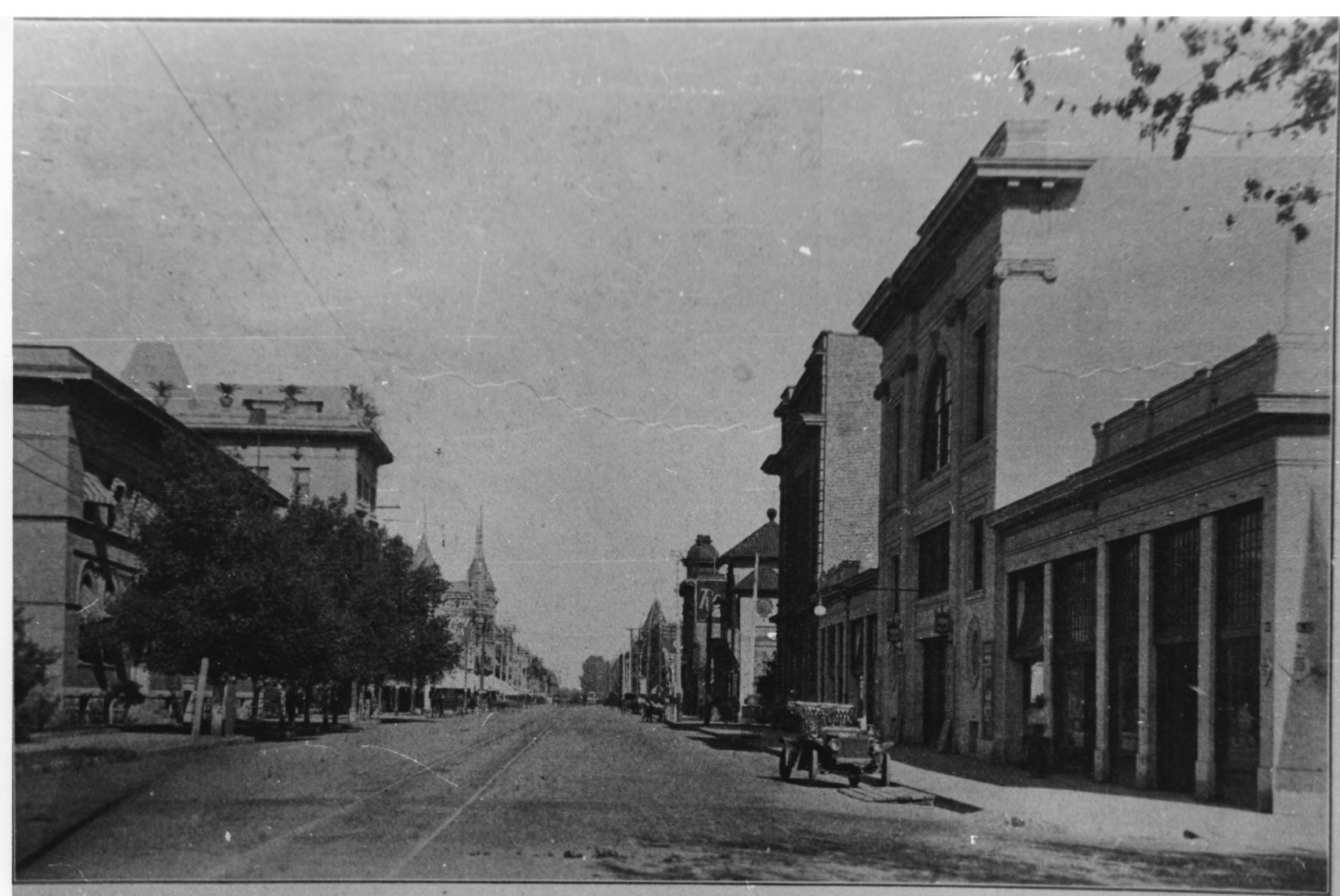
Nineteenth Street — Showing Bakersfield Opera House, the Kern County Land Company Building, the Oil Exchange, the Producers Bank Building
