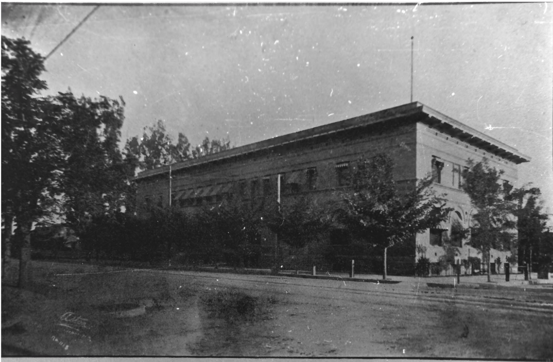
KERN COUNTY LAND CO. BUILDING COR. 19TH AND H STREETS Office Kern County Land Company and Kern County Canal and Water Company
