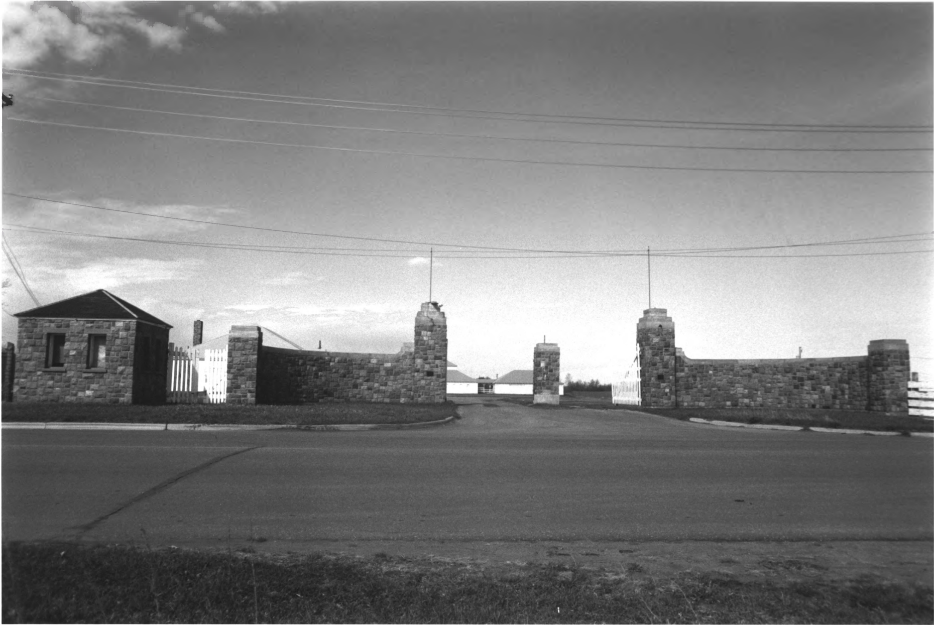
Entrance, Mahanomen County Fairgrounds Historic District Mahanomen, MN 09235/17
