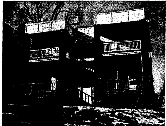
Significant Loss of Integrity, Missing Porch Entablature, Roof, Cornice, and Railings
