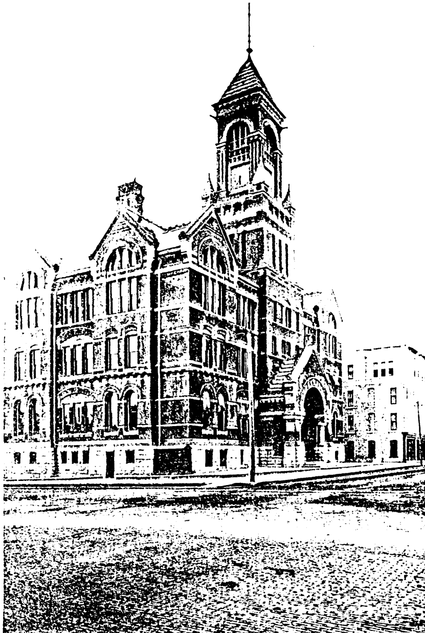
1903, Mahaska County Courthouse, view to southeast.
