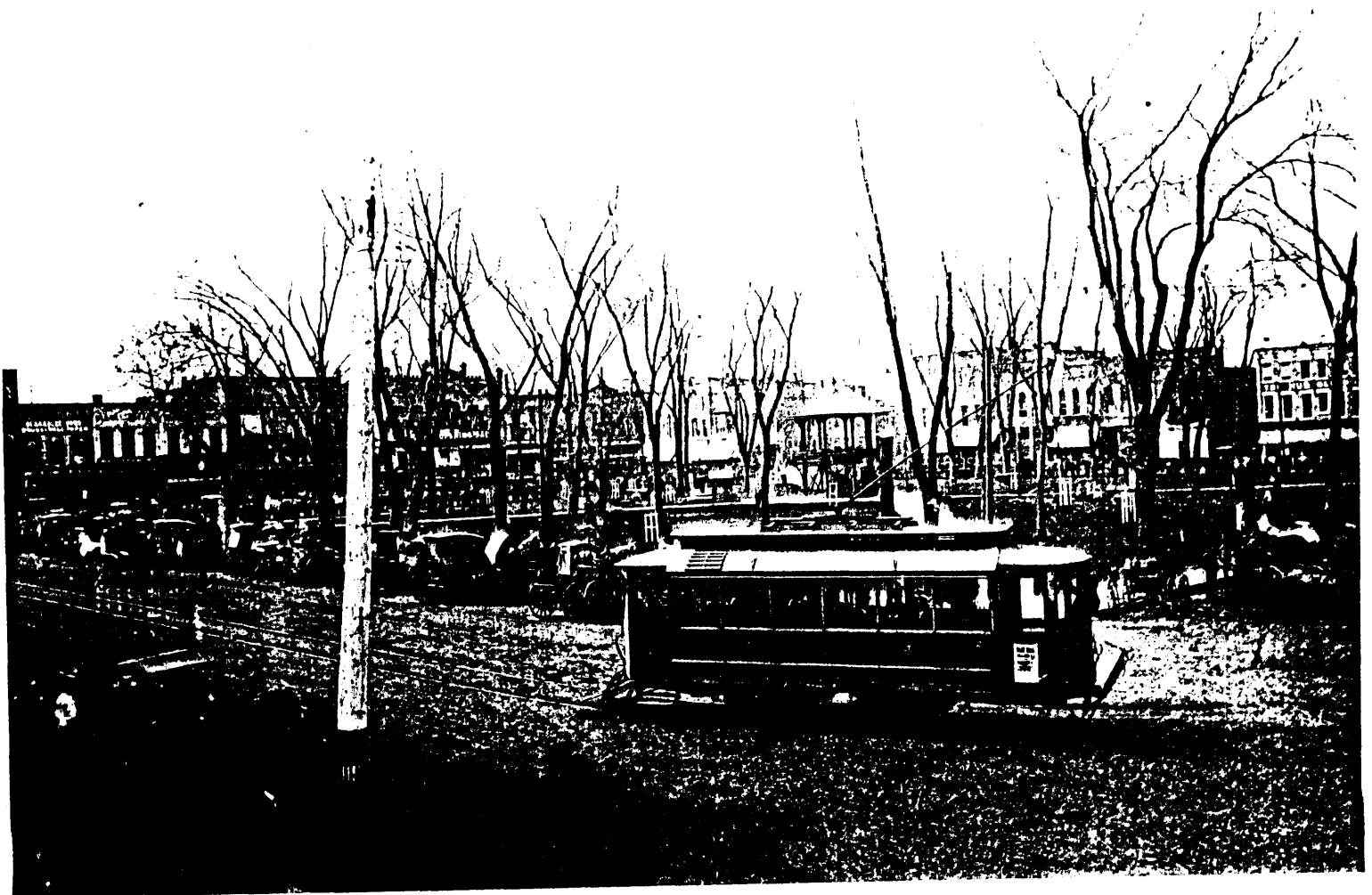
1902, Harry Nix photo, Southeast corner of square, view to northwest.
