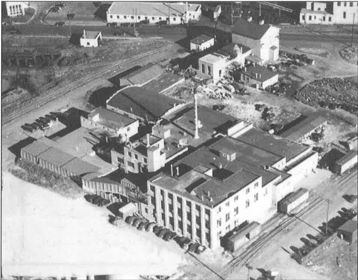
Figure 15. Superior Packing Company Plant, facing northeast, before cattle ramp and pens were built in brick, 1937. (MNHS)
