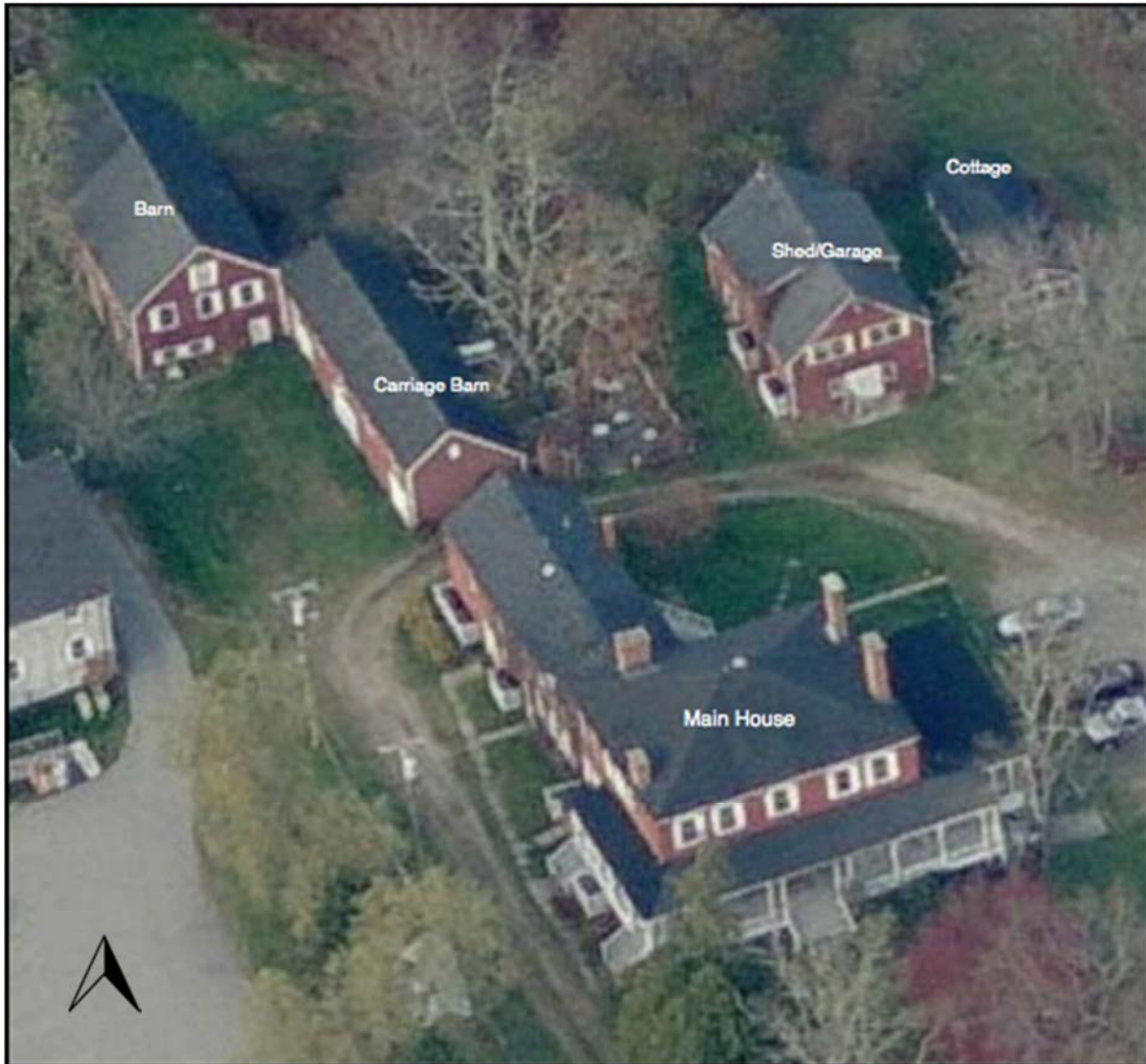
SOUTHGATE FARM SCARBOROUGH, MAINE BIRD'S EYE VIEW (2015 image)
