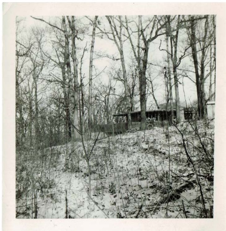
Figure C: Himmelfarb House nears completion (1942)
