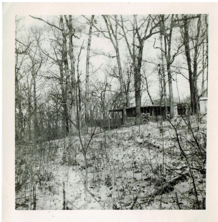
Figure C: Himmelfarb House nears completion (1942)
