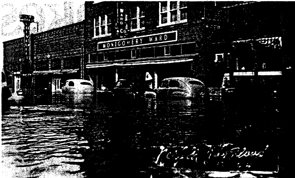
Norfolk's devastating flood of 1944 destroyed the WJAG basement offices in the Hotel Norfolk. This picture is of the first block of North 4th Street.
