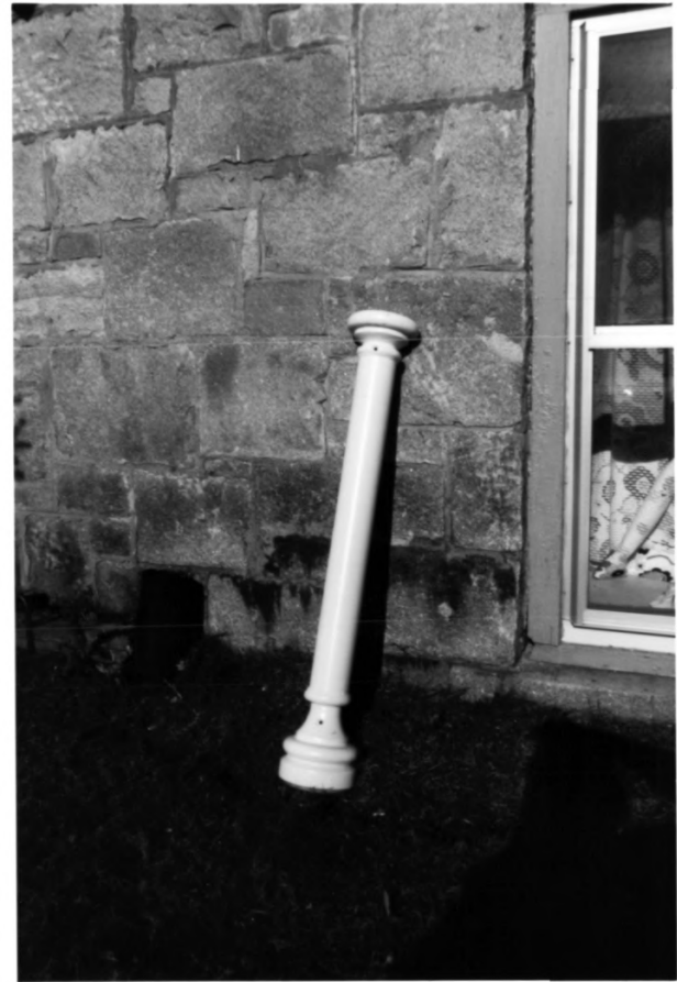
Photo 11. Belfry attached column, normal view.
