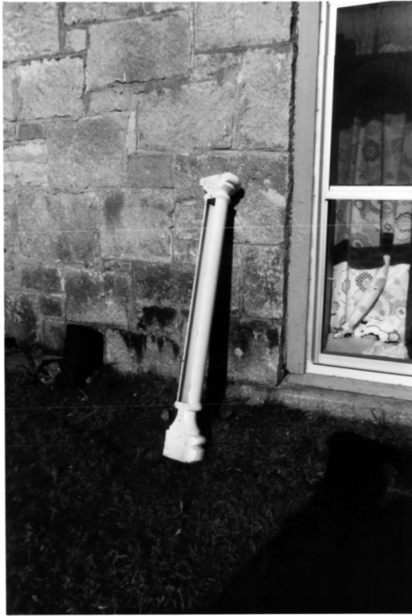
Photo 10. Belfry attached column, showing hollow constuction.
