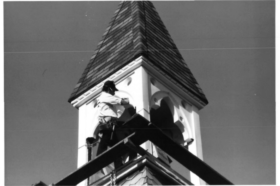
Photo 7. At work on the belfry. (See Photo 1.)
