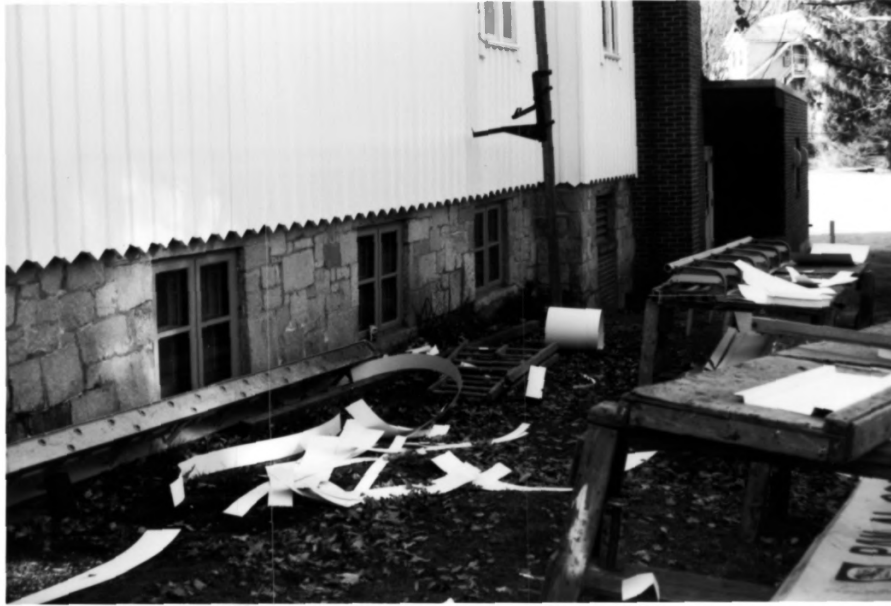
Photo 3. Work area north of church, view southwest.
