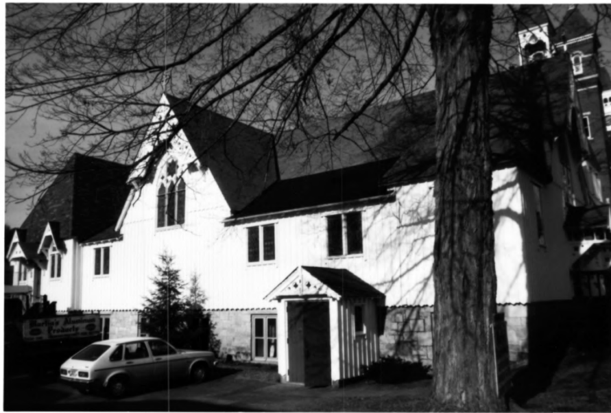
Photo 2. South elevation, view northwest.
