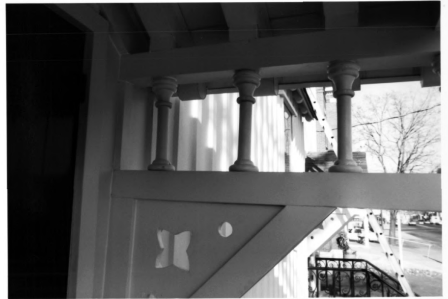
Photo 9. Obverse of Photo 8. Spindles also are cast.
