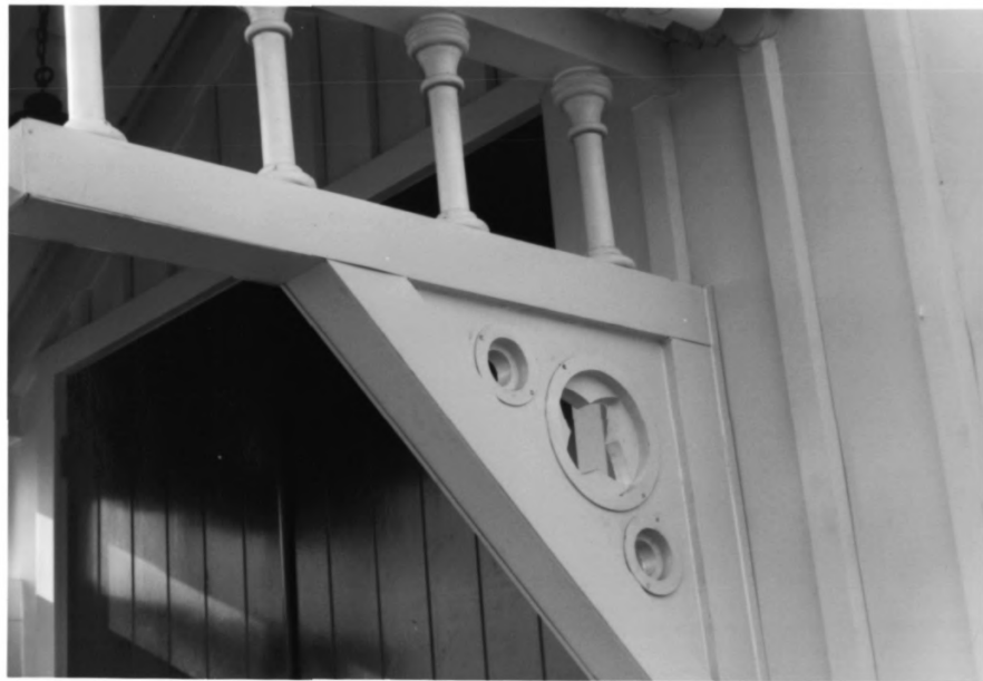
Photo 8. Star casting put into place with its flange overlapping the flat sheet.
