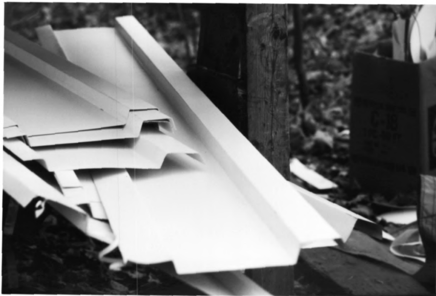
Photo 4. Sheet aluminum pieces shaped to fit over board and battens.
