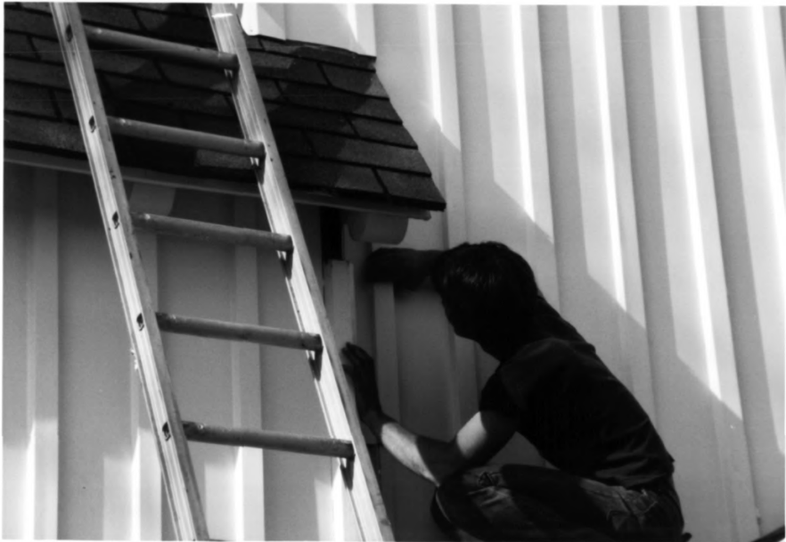
Photo 6. Fitting the piece into place.
