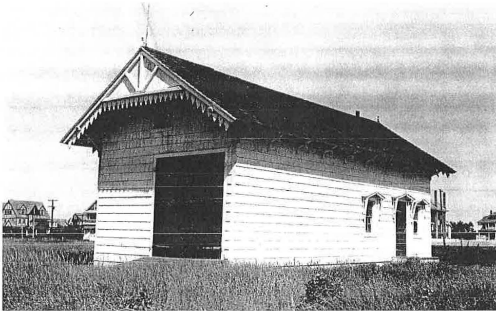
Figure 3: Cold Spring Life-Saving Station, Cape May, NJ Station is believed to have been similar to the 1853-1854 Ocean City boathouse U.S. Coast Guard
