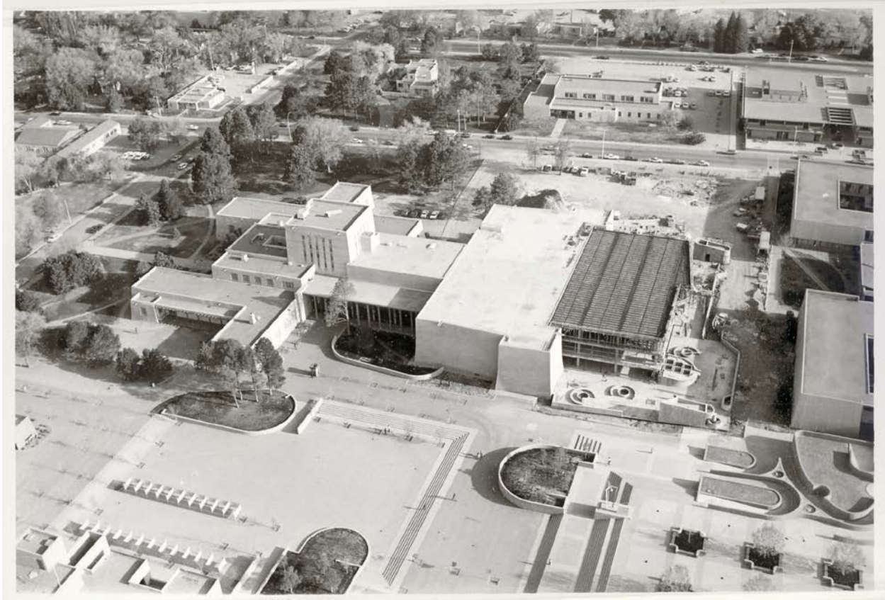
Zimmerman Library with 1974 addition under construction
