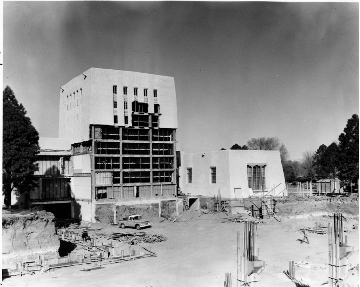
East façade of Meem library (1936) altered for construction of 1966 addition
