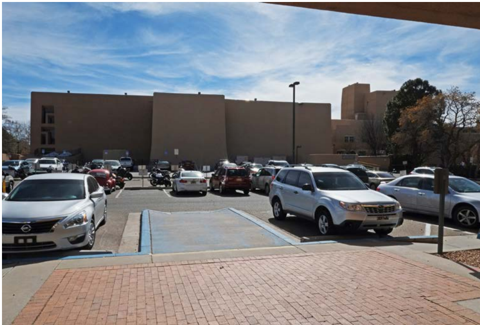
14 of 40. North elevation with 1966 and 1974 additions, photographer facing north.
