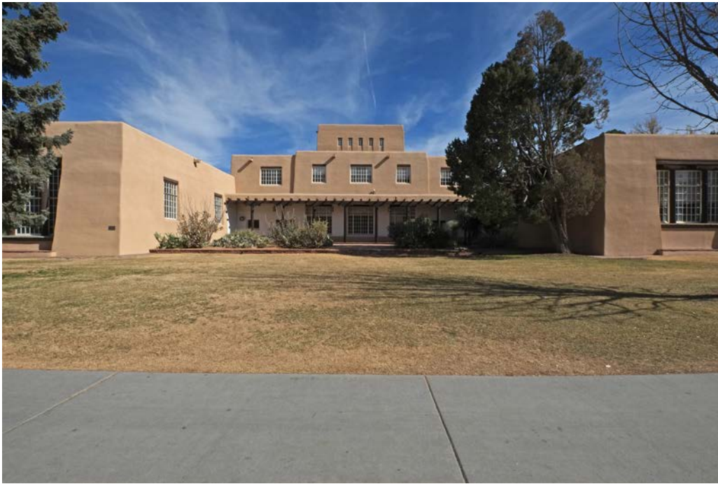
1 of 40. Main (west) facade, photographer facing east.
