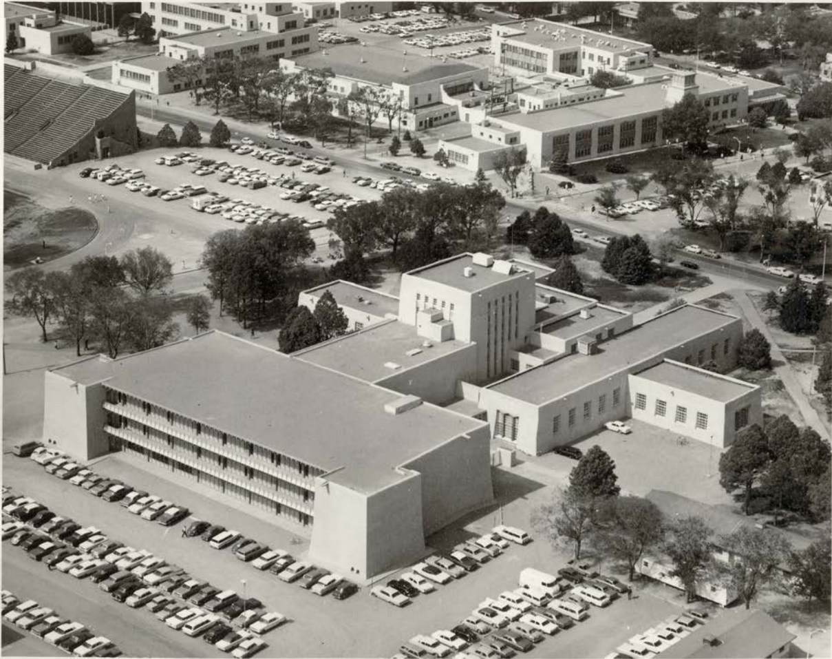
Zimmerman Library with 1966 addition
