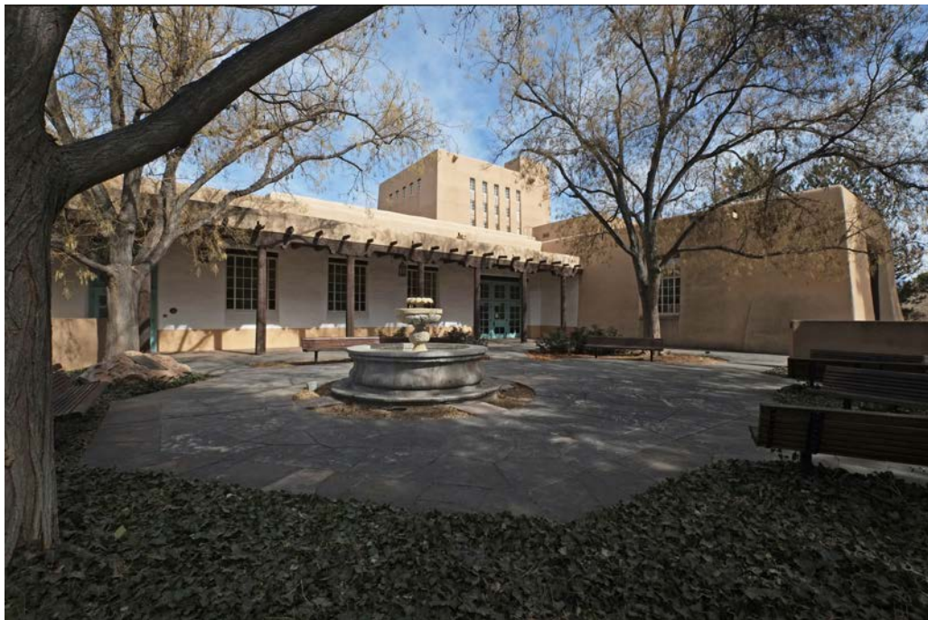
6 of 40. Portal and courtyard on south side, photographer facing northeast.
