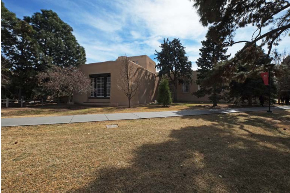
17 of 40. North (left) and west (right) reading rooms, photographer facing southeast.
