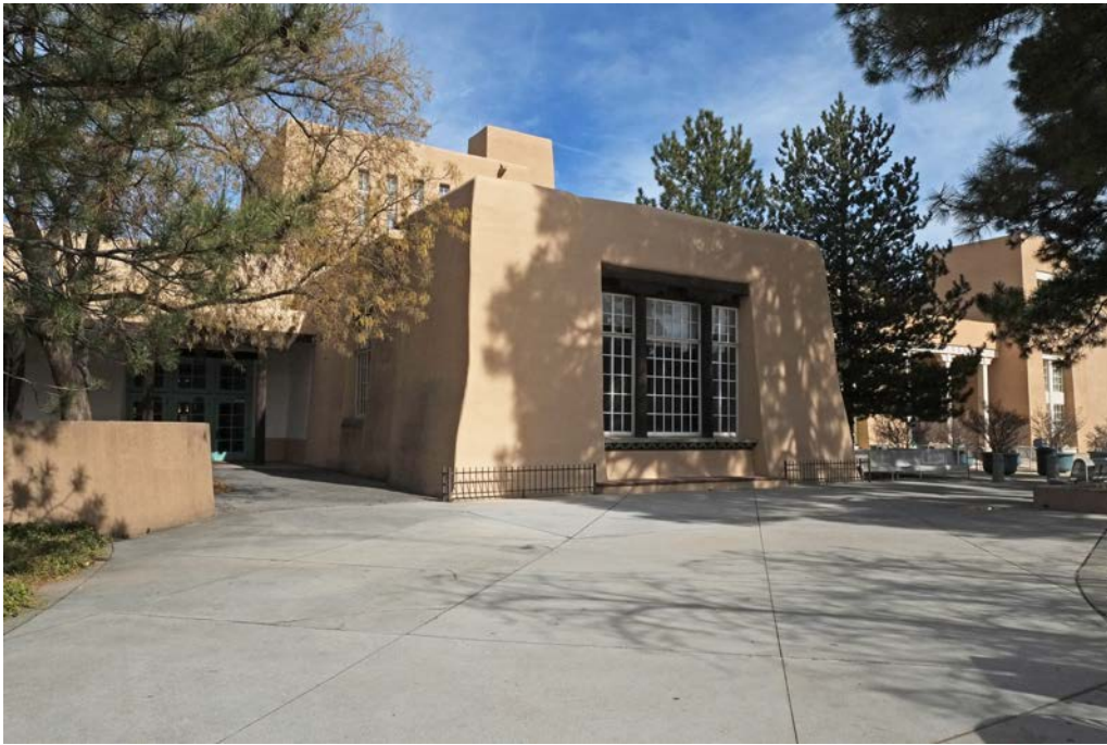
9 of 40. South reading room, photographer facing northeast.
