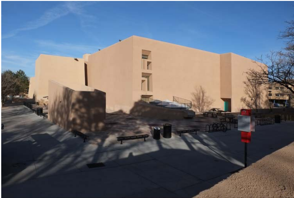
13 of 40. South and east (rear) sides of 1966 and 1974 additions, photographer facing northwest.
