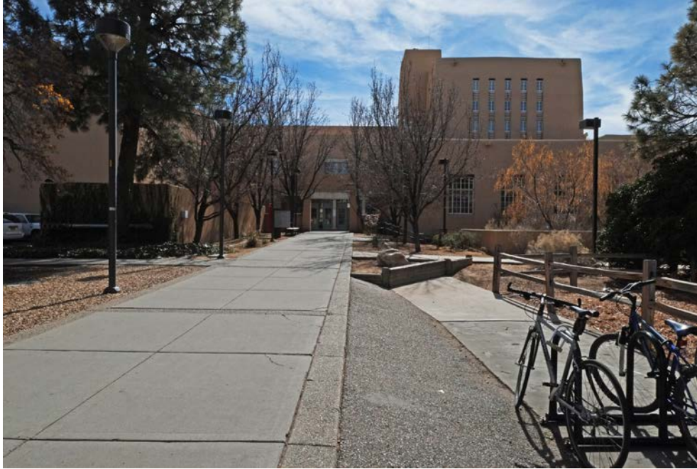
15 of 40. North elevation with stack tower, photographer facing north.
