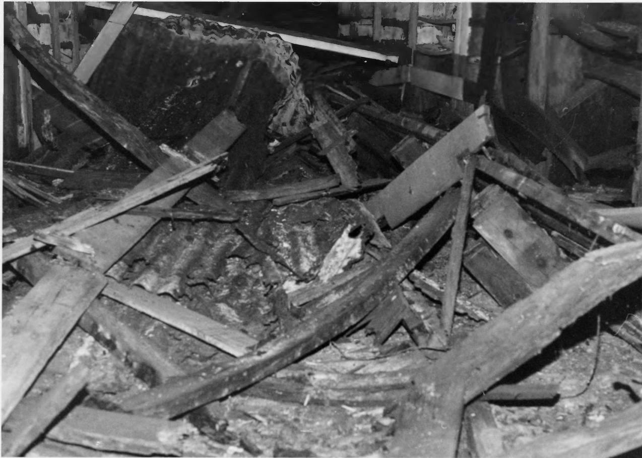
10. Inside a Japanese underground structure on Peale Island. Although it was stoutly constructed with heavy plank and steel beams, its interior lining is fast caving in.
