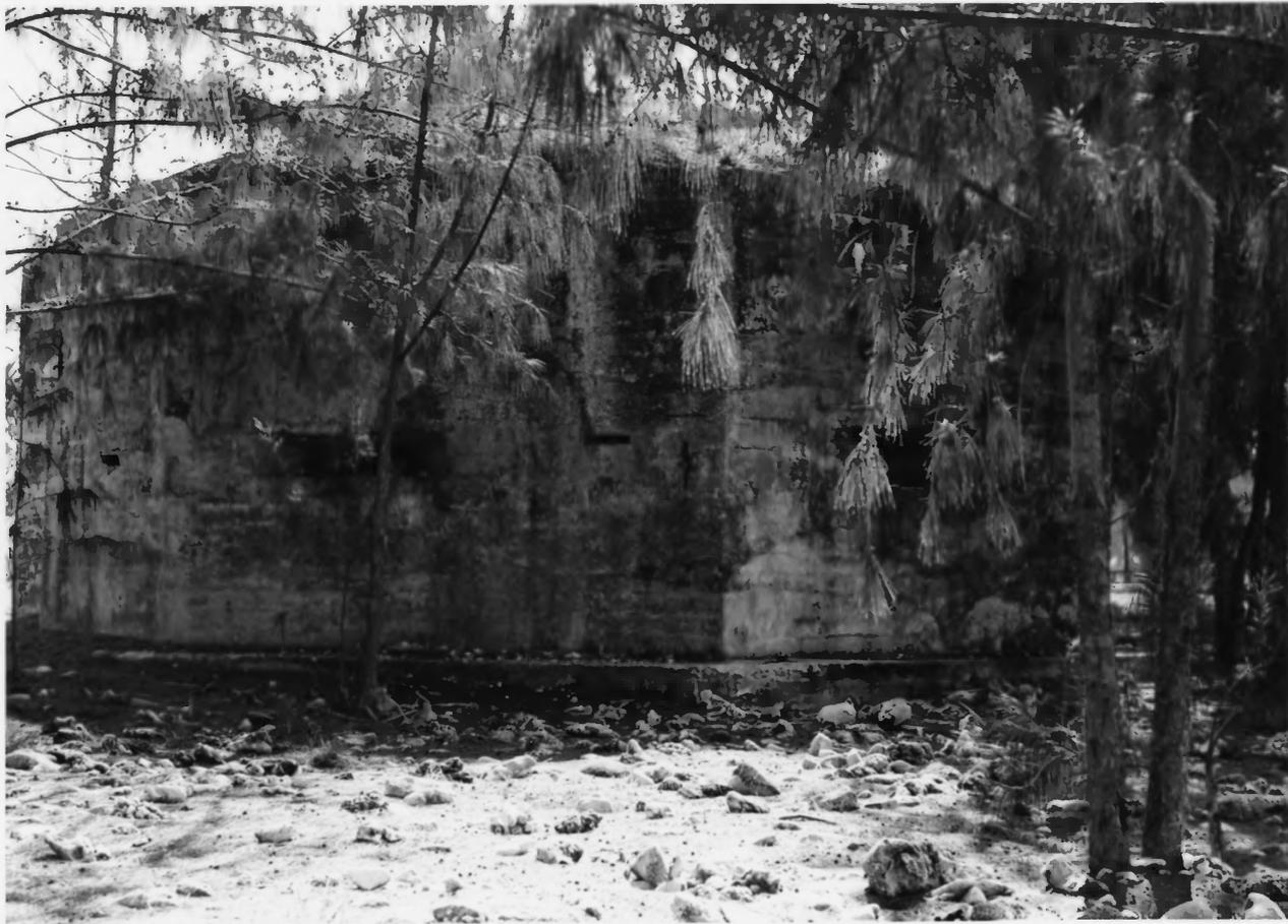
4. Largest Japanese blockhouse on Wake. This six-sided structure, containing both gun embrasures and rifle slits, stands between the admiral's command post and the ocean, northwest corner of Wake Island.
