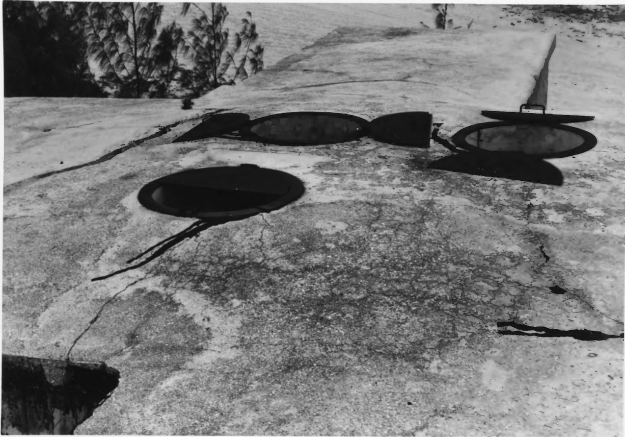
3. Steel-protected observation posts on the roof of Admiral Sakaibara's command post, Wake Island. This strong, three-level structure stands near the bridge to Peale. Only one level is accessible.
