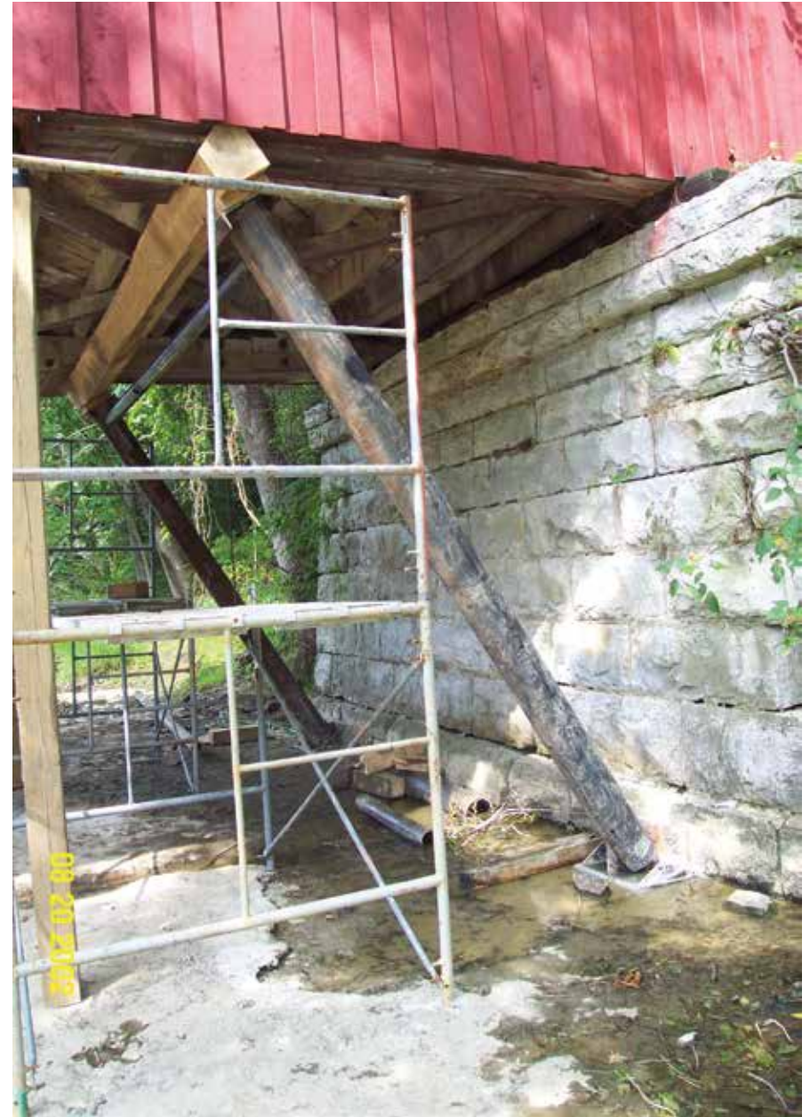
Figure C2.4 Temporary shoring installation. J. A. Barker Engineering, August 2002.
