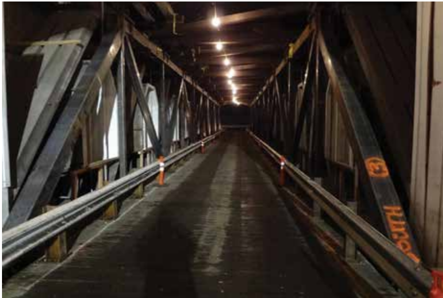
Figure C6.6 Both temporary steel trusses in place; bridge open to traffic, 2013.
