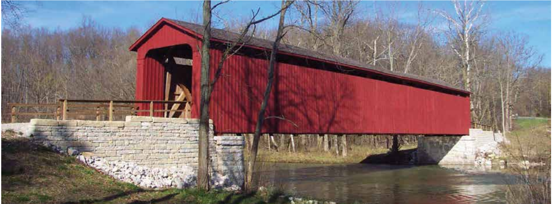
Figure C2.1 Cataract Falls Covered Bridge after rehabilitation. Matthew Reckard, 2006.
