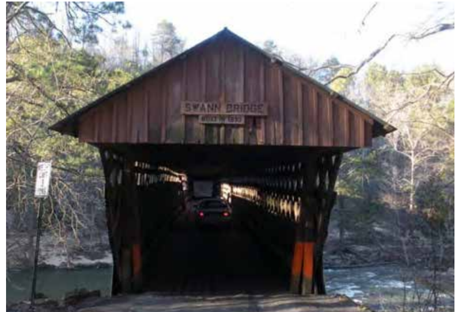
Figure C11.4 General view, looking west. TranSystems, 2009.
