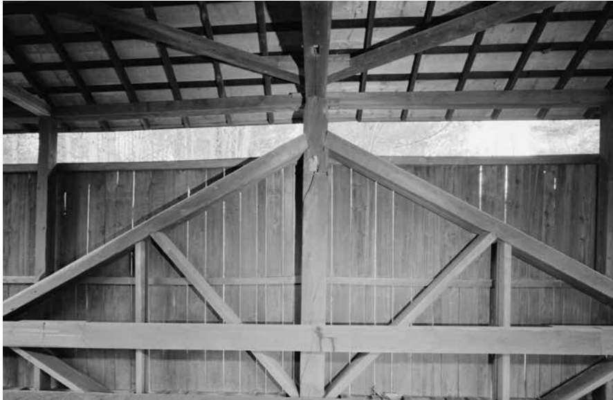
A single kingpost truss supports this short 48' long bridge.
