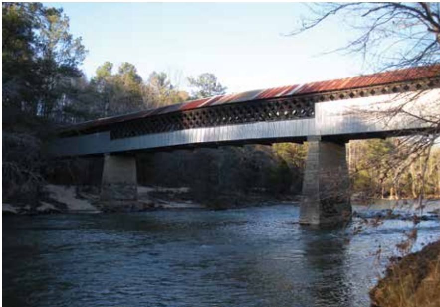
Figure C11.2 South elevation, looking northwest. TranSystems, 2009.
