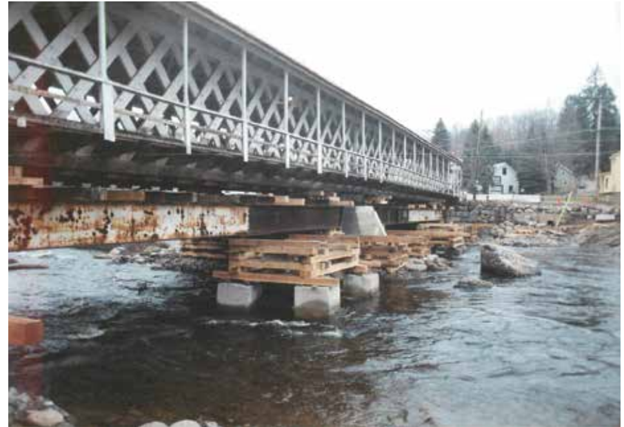
Figure C1.8 Shoring underneath bridge. Sean T. James, 1998.
