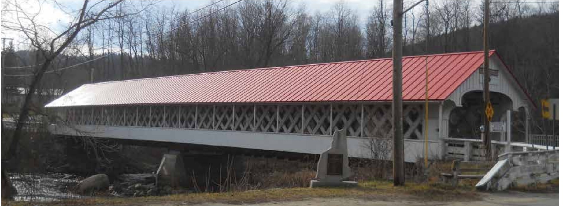
Figure C1.1 Upstream elevation of Ashuelot Covered Bridge. Sean T. James, 2012.
