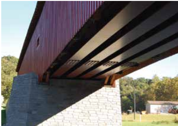
Figure 3.4a-b When repairing or replacing masonry elements, similar materials and construction techniques should be utilized. If possible, modern veneer panels should be avoided, such as at Pine Grove Bridge, PA, where the original floor system was replaced by steel I-beams.
