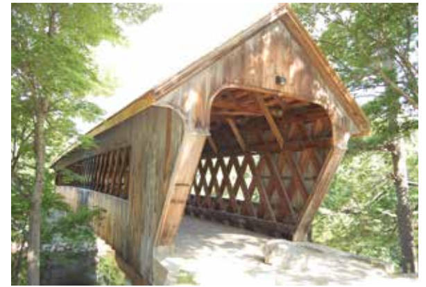
Figure 5.4e-f To provide accessibility to the Sachs Covered Bridge in Pennsylvania, Adams County employed matching stone for an ADA compliant ramp. A simple boulder is used as a bollard on the pedestrian-only Henniker Bridge, NH.
