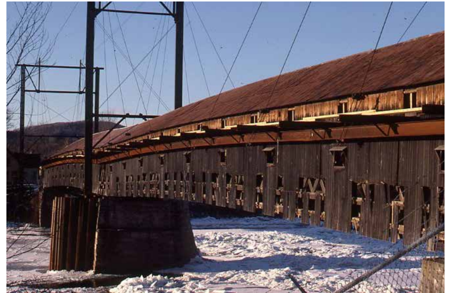
Figure C3.3 Tower system erected prior to rehabilitation work. James L. Garvin, December 1988.
