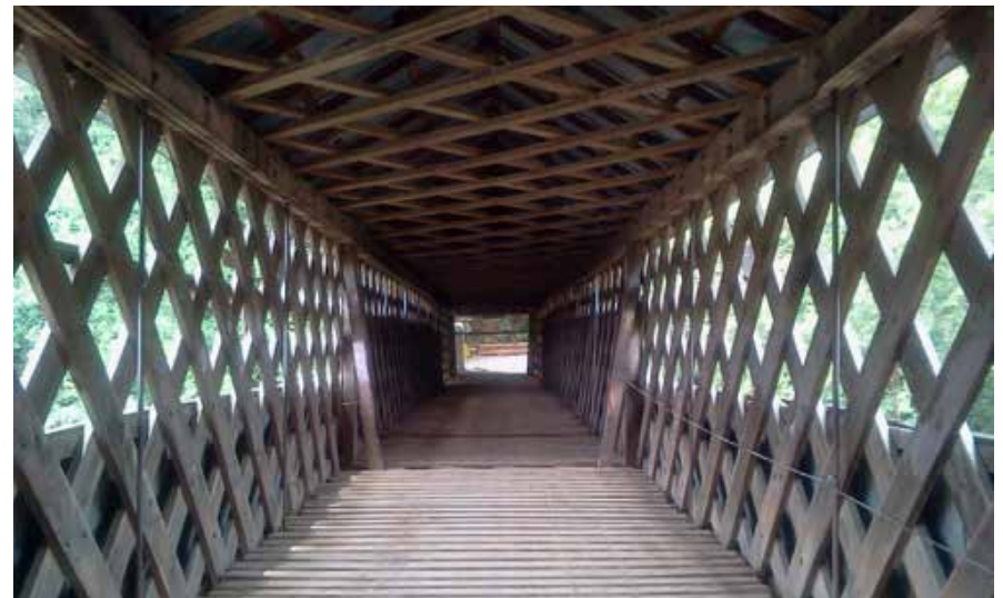
Figure C11.6 Floor, runners, and rail removed. TranSystems, 2012.
