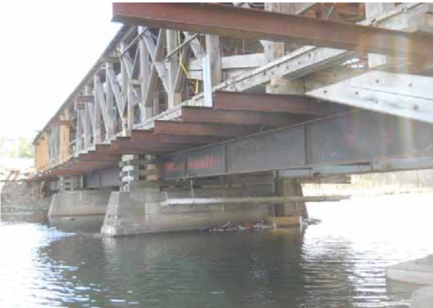
Figure C10.15 Temporary shoring system, looking south. Josif Bicja, April 2012.
