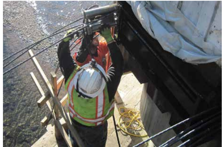
Figure C6.8 Jacking the PT strand, 2013.
