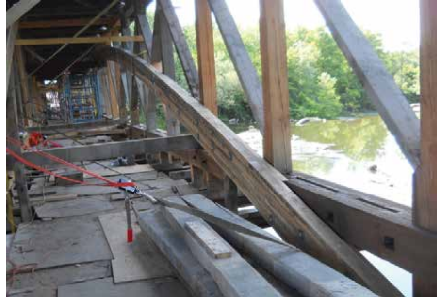
Figure C10.19 Replaced portion of north arch, east end. Josif Bicja, July 2012.
