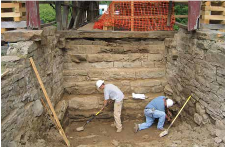
Figure C8.11 Excavated abutment before reinforcement. SCLA.
