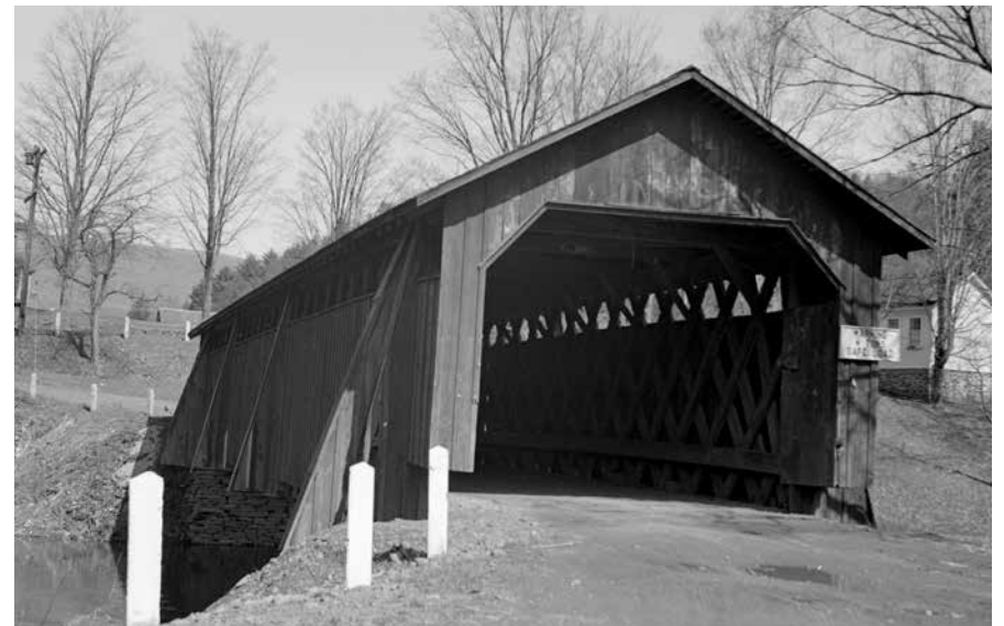
Figure C4.2 Historic view of Fitch's Covered Bridge, note outriggers. Richard Sanders Allen.
