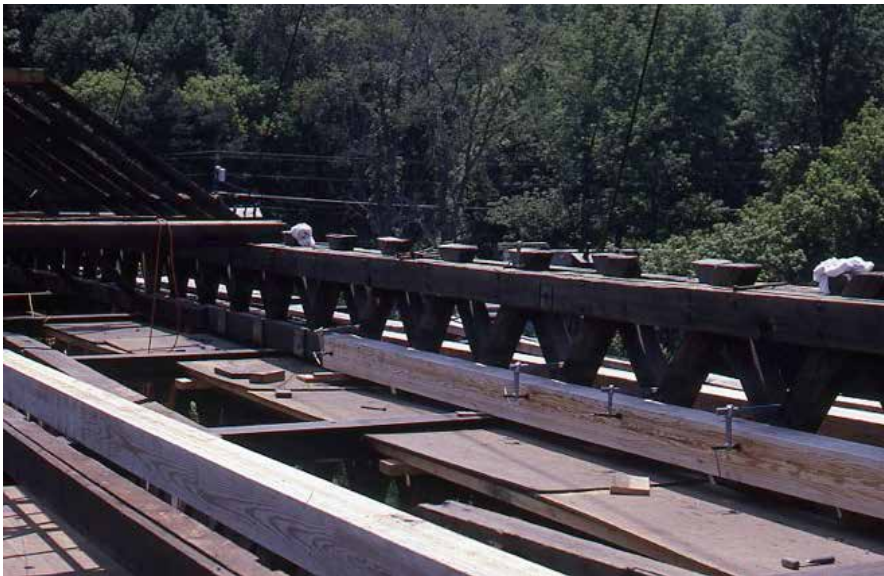
Figure C3.7 Original upper chords with glulam replacement chord. James L. Garvin, June 1989.
