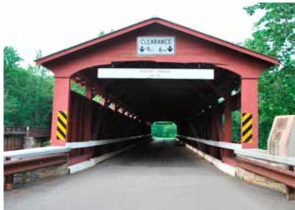
Figure 5.4c-d Strategies for limiting height include "headache" bars, which are a cost effective way to protect the portal and knee-braces of the bridge, and control entry of overweight vehicles.
