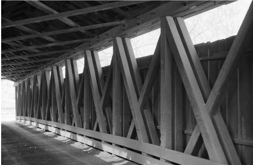
A long truss, with paired braces and single counterbraces.
