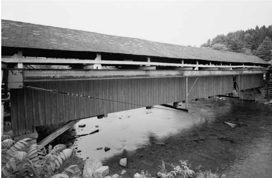
Figure C8.8 Stabilization of the bridge, showing tension cables tied to steel I-beams. HAER PA-638-3, Jet Lowe, 2005.
