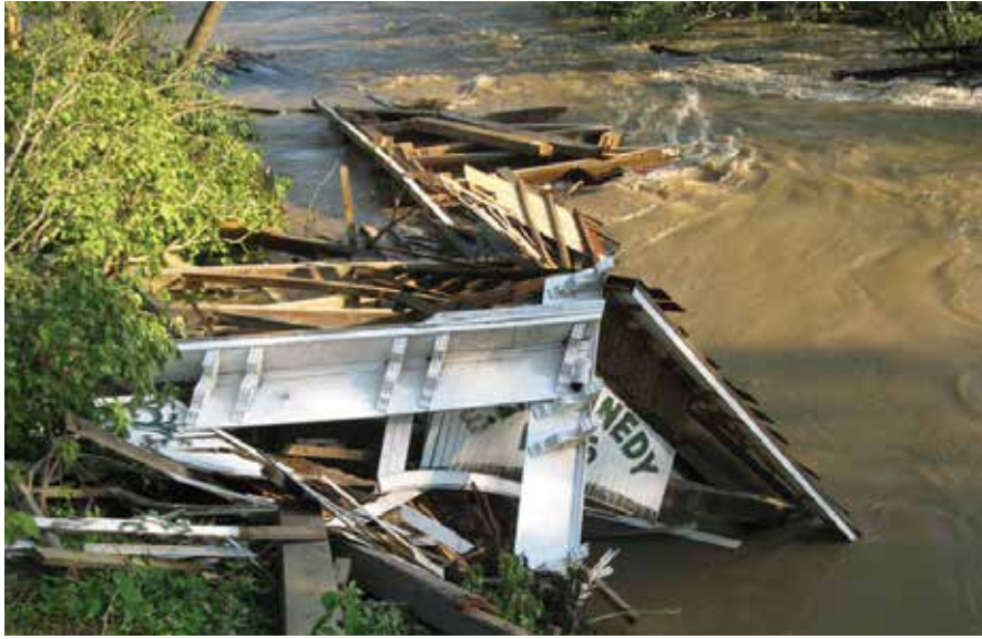
Figure C9.5 View of Moscow Bridge after the 2008 tornado. Part of the east portal remains, but the river washed away most of the span. Ed Derringer, 2008.
