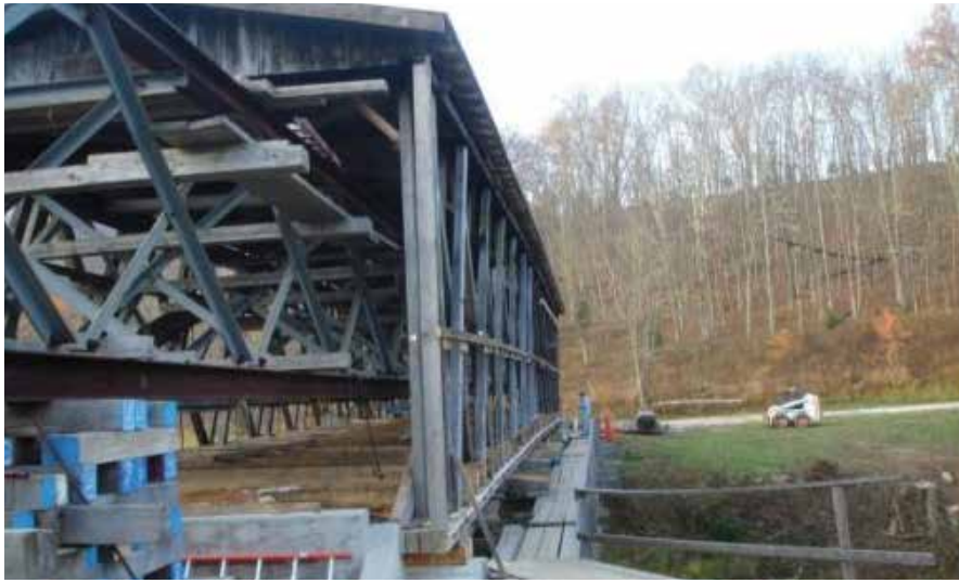
Figure C7.6 View of bridge after camber was restored to 9". William Caswell, 2008.
