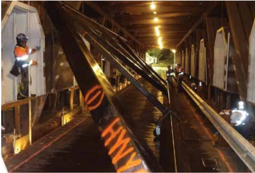
Figure C6.5 Installation of first temporary steel truss during night closure, 2013.
