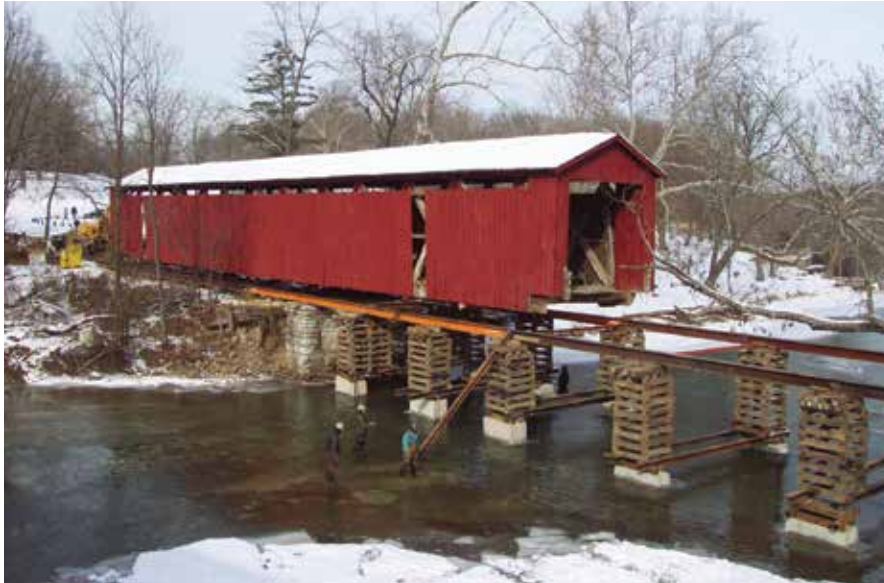
Figure C2.5 Moving bridge off the river. J. A. Barker Engineering, January 2003.
