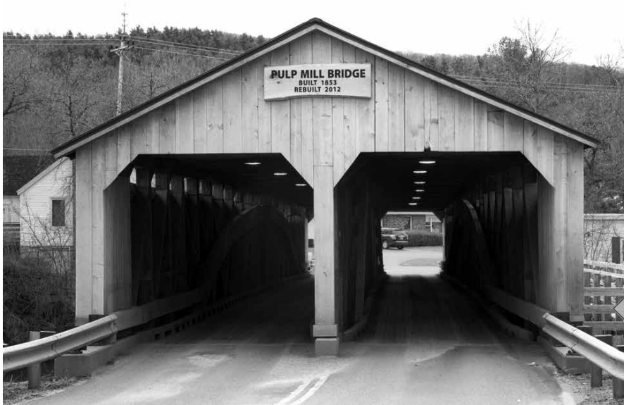
The double-barrel Pulp Mill Covered Bridge, VT, accommodates two lanes of traffic.
