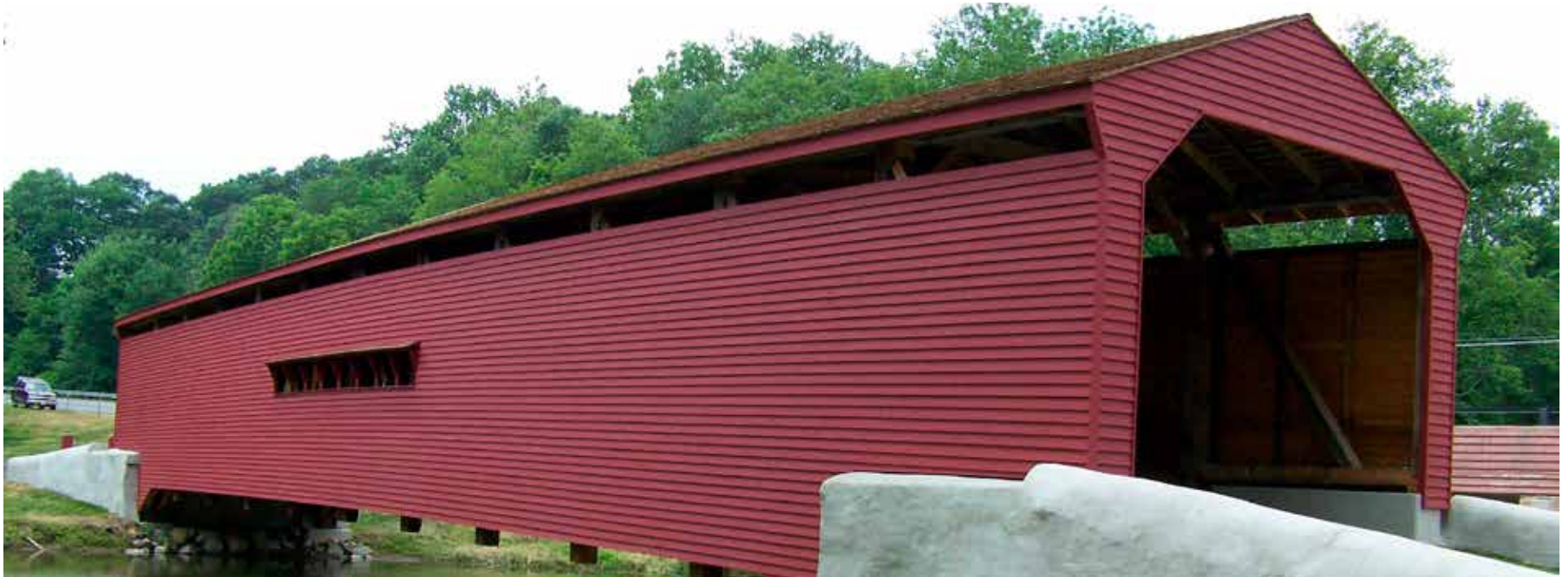
Figure C5.1 Completed rehabilitation of Gilpin's Falls Covered Bridge. W. Earl Simmers, 2010.
