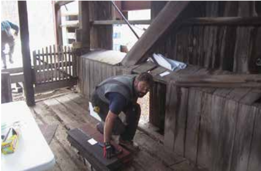
Figure C8.5 Human and livestock gates at east portal. Note the diagonal repair rods through the truss braces, which were installed early in the twentieth century. SCLA.
