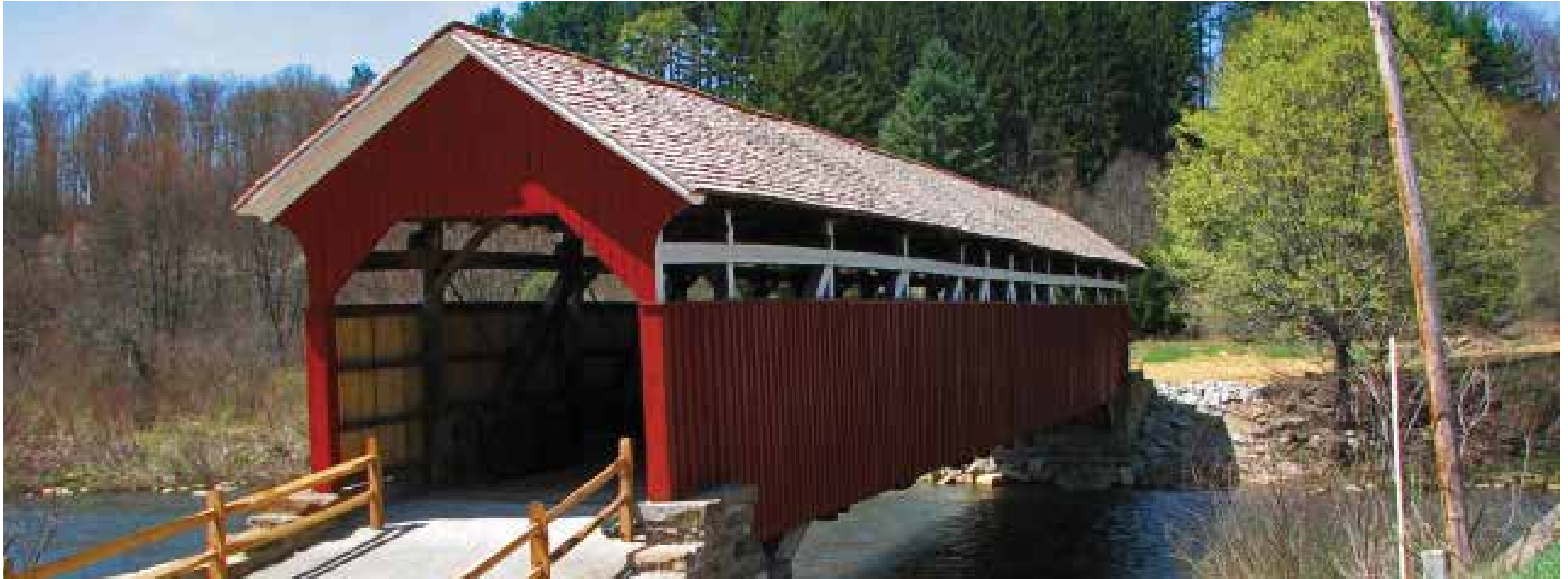
Figure C8.1 Completed rehabilitation of King's Covered Bridge. Simone Collins Landscape Architecture (SCLA), 2008.
