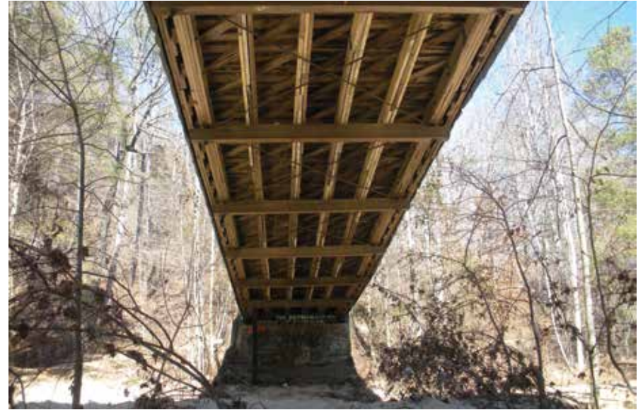
Figure C11.3 General underside view, looking west. TranSystems, 2009.
