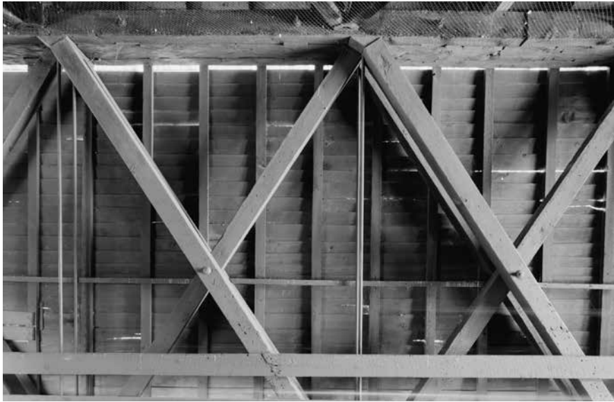
Paired, vertical iron tension rods in a Howe truss.
