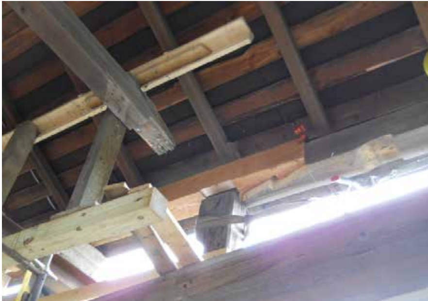
Figure C10.20 Typical top chord scarfed joint. Josif Bicja, July 2012.
