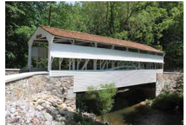
Figure 3.5e-f Before/after abutment at Knox Bridge, PA. The arch, chord, and post were all encapsulated in concrete, leading to heavy decay. The reconstructed abutment was designed to allow ease of cleaning and maintenance. Note the use of rot-resistant black locust bearing blocks and copper naphthanate to protect and defend the arch ends, end post, and end brace against decay.
