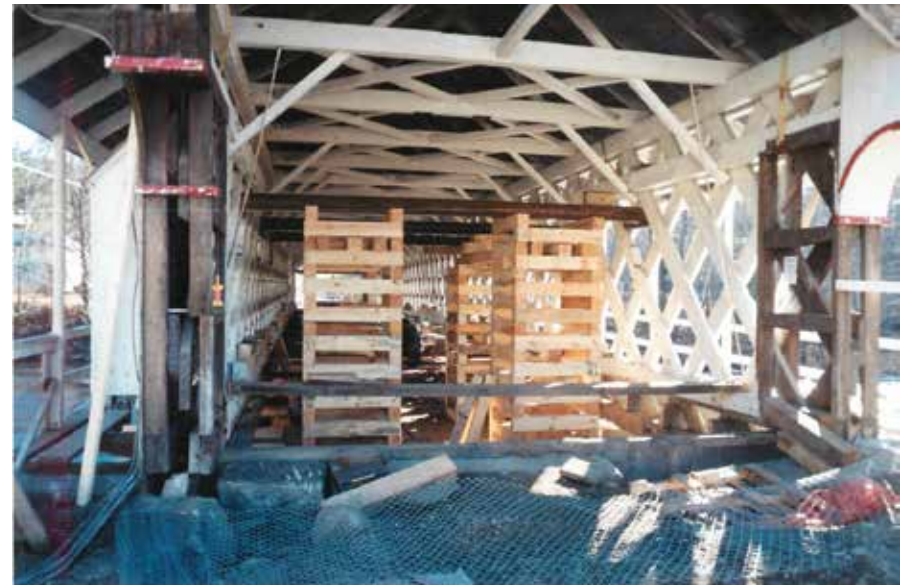
Figure C1.9 Interior shoring. Sean T. James, 1998.
