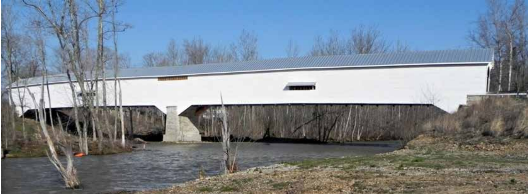
Figure C9.1 The rebuilt Moscow Covered Bridge. Arthur Gatewood, 2010.
