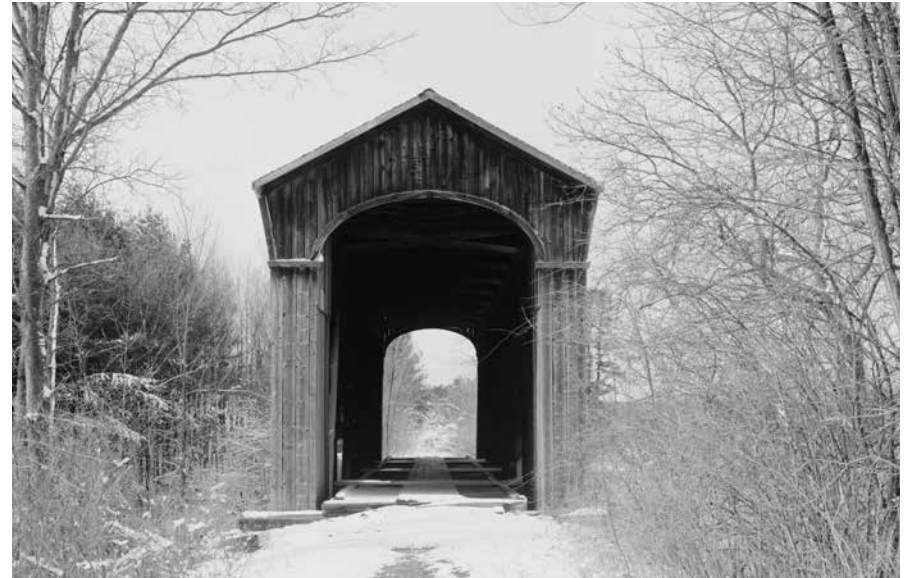
Portal of Shoreham Railroad Bridge, VT.
