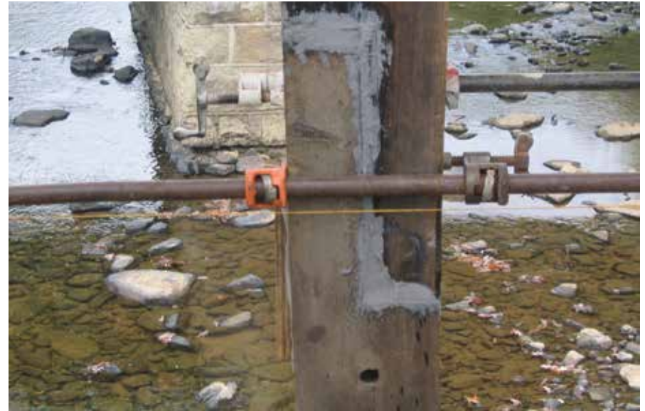
Figure C8.12 GFRP post repair. SCLA.
