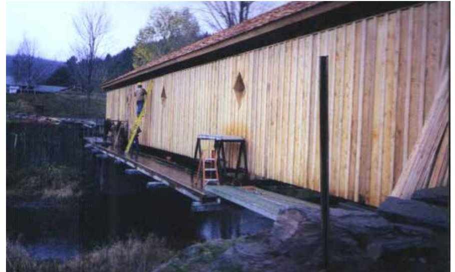
Figure C4.9 Siding being replaced with rough-cut 1" x 12" hemlock with battens. DCDPW.
