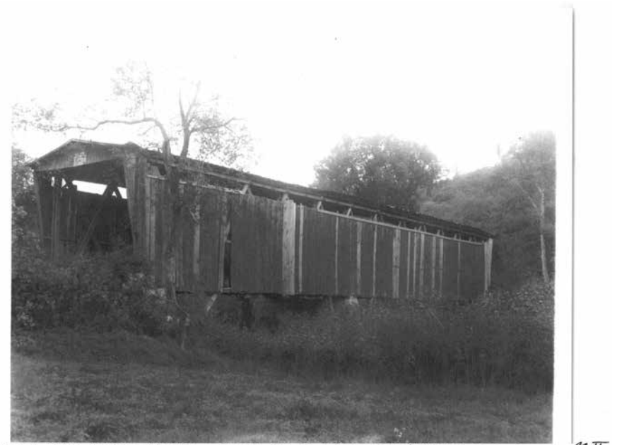
Figure C7.2 Johnson Creek Bridge in September 1951. Courtesy of John E. Thierman Photographic Collection, 1944-1970, PA 2, Special Collections, Transylvania University, Lexington, Kentucky.
