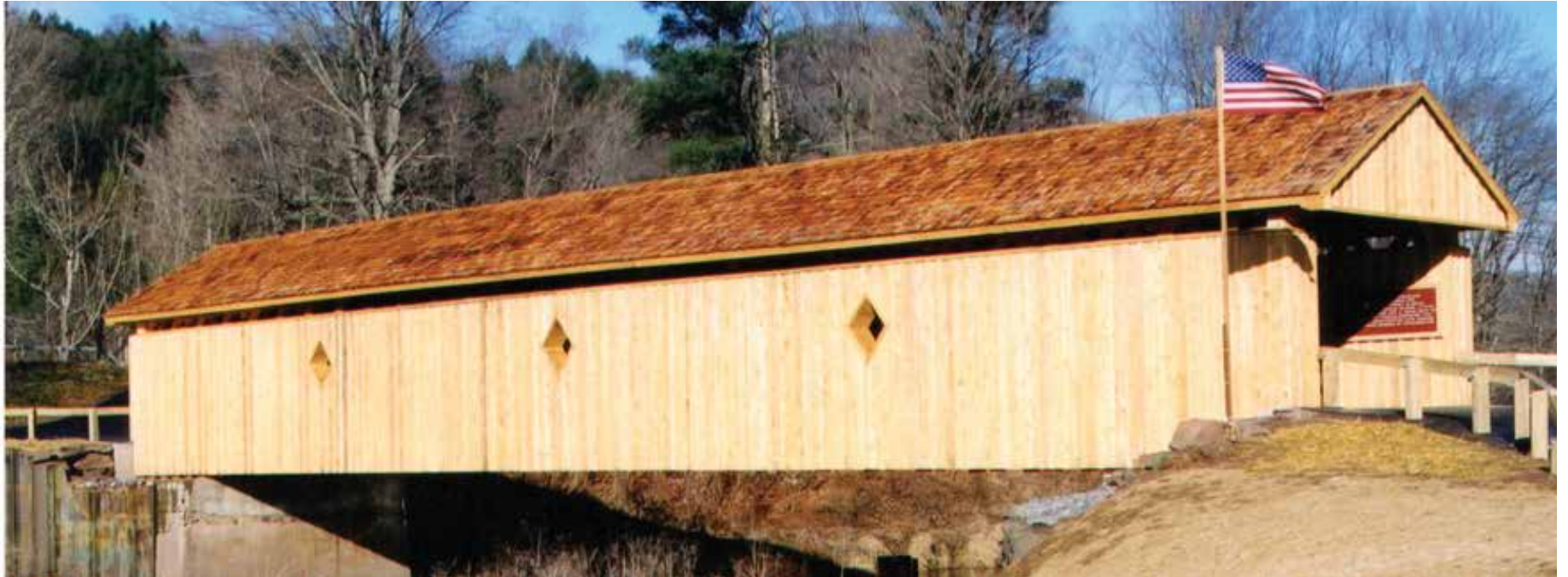
Figure C4.1 Fitch's Covered Bridge after completion with new diamond openings. Note timber railing system at left at north approach. Phillip C. Pierce, 2002.
