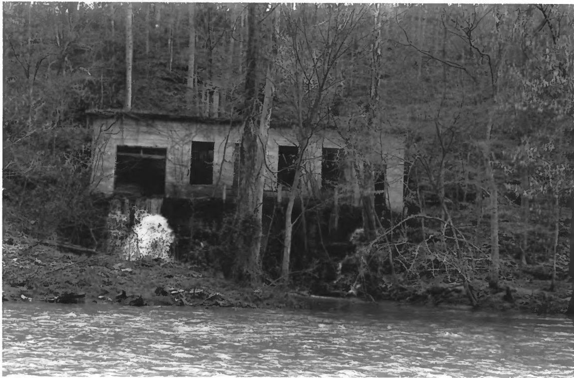
Lawrenceburg No. 1 Hydroelectric Station Lawrenceburg vicinity, Lawrence County, TN
