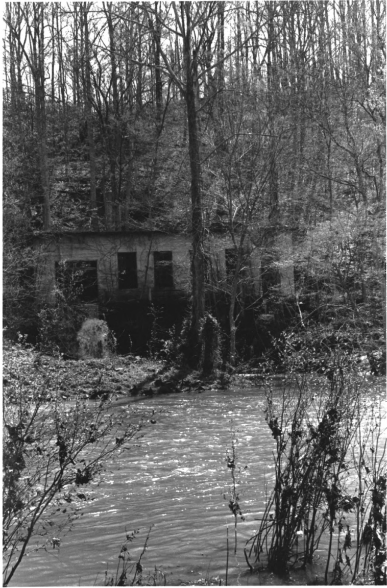
Lawrenceburg No. 1 Hydroelectric Station Lawrenceburg vicinity, Lawrence County, TN #3 of 4
