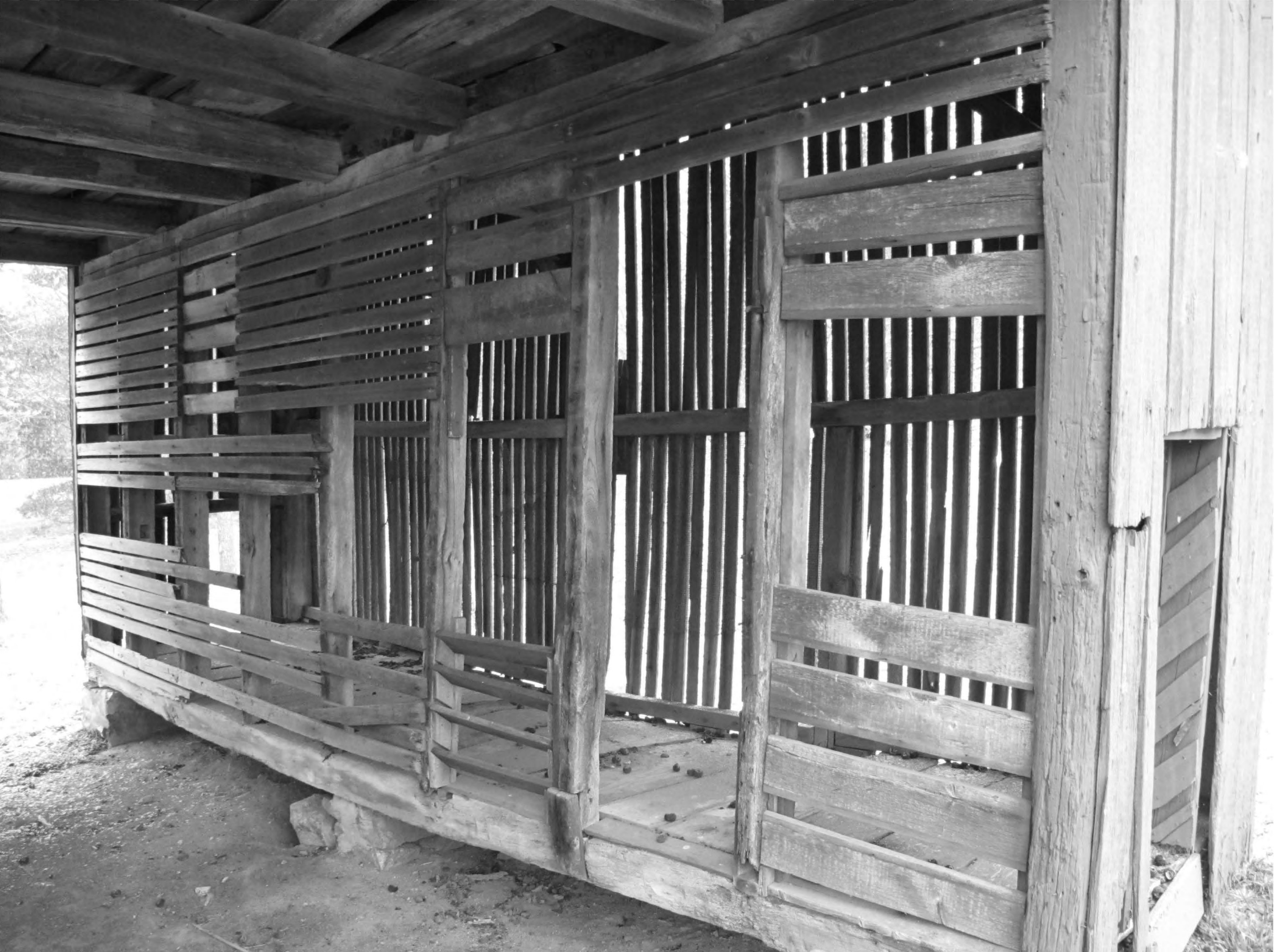
Cox-Phillips-Mitchell Agricultural Complex_New Castle County_DE Corncrib looking north
