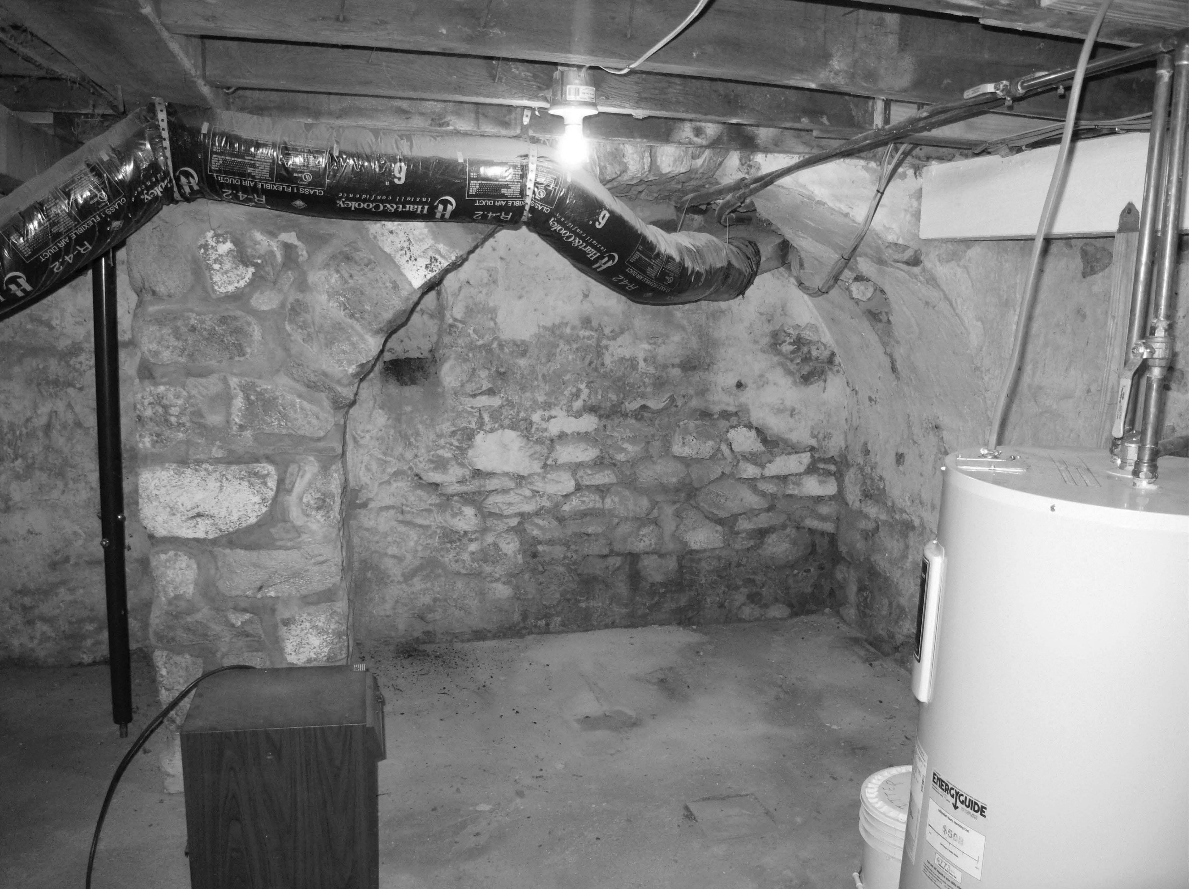
Cox-Phillips-Mitchell Agricultural Complex_New Castle County_DE Basement interior showing relieving arch on northeast wall looking northeast
