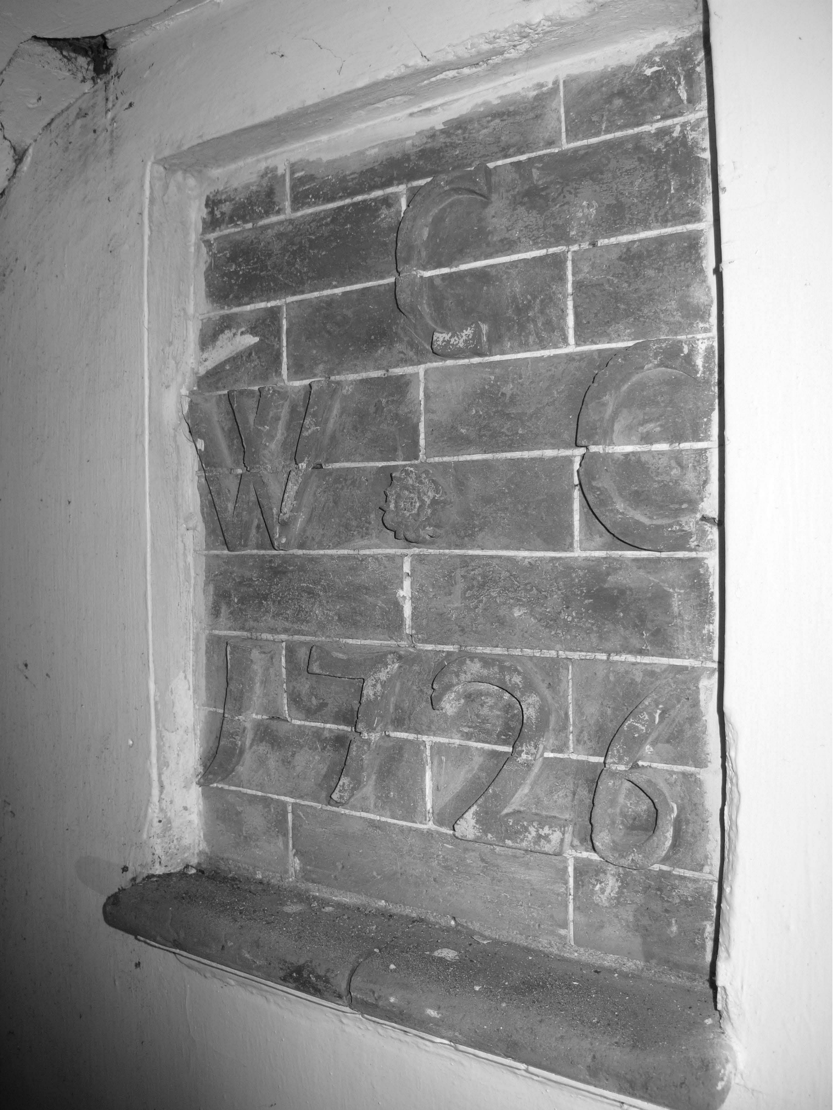
Cox-Phillips-Mitchell Agricultural Complex_New Castle County_DE Attic interior showing the now-enclosed Period I date stone dated 1726 looking south
