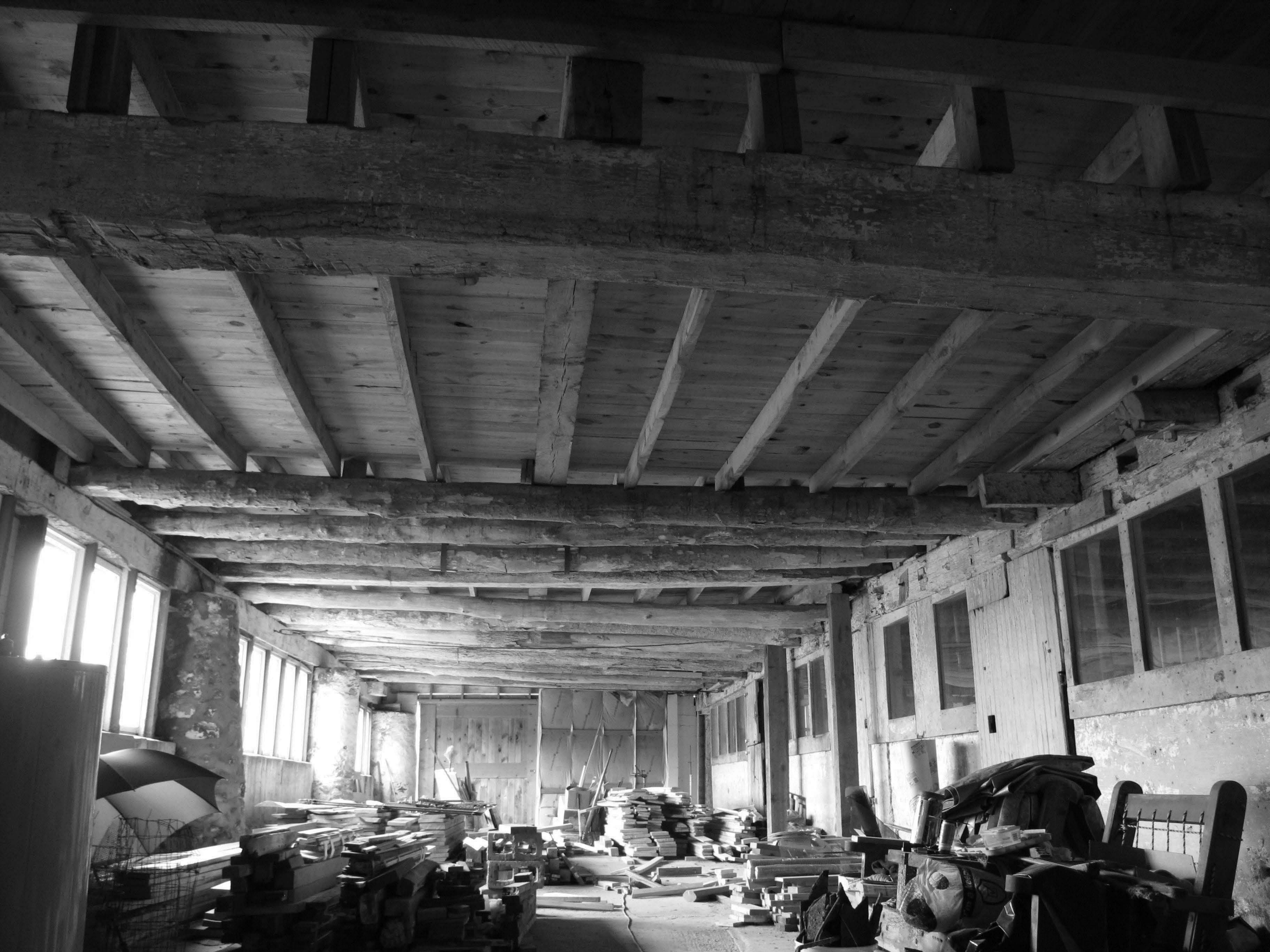
Cox-Phillips-Mitchell Agricultural Complex_New Castle County_DE Dairy barn interior, lower level, southeast room showing log joists looking southwest
