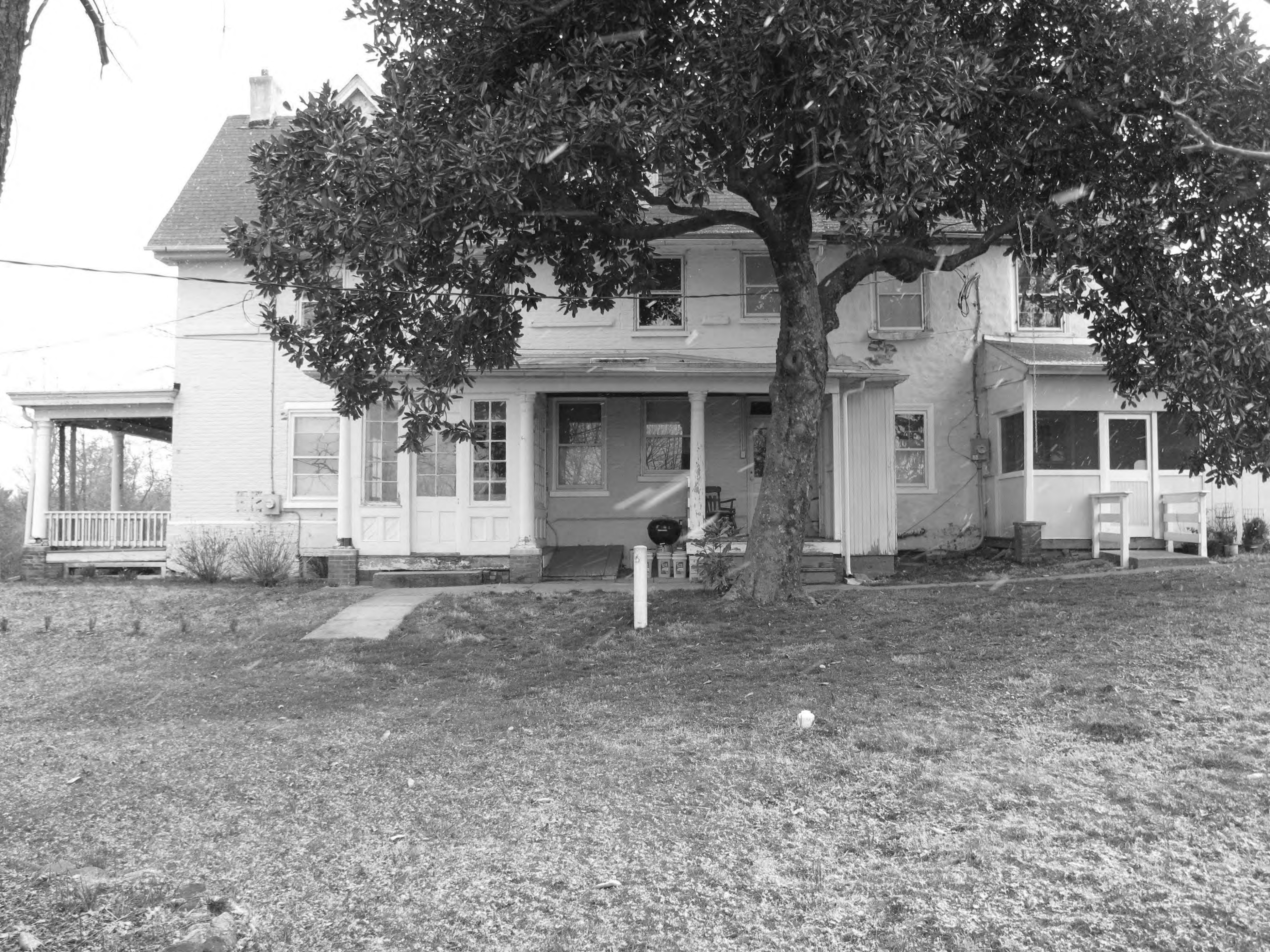
Cox-Phillips-Mitchell Agricultural Complex_New Castle County_DE View of southeast elevation of house looking northwest
