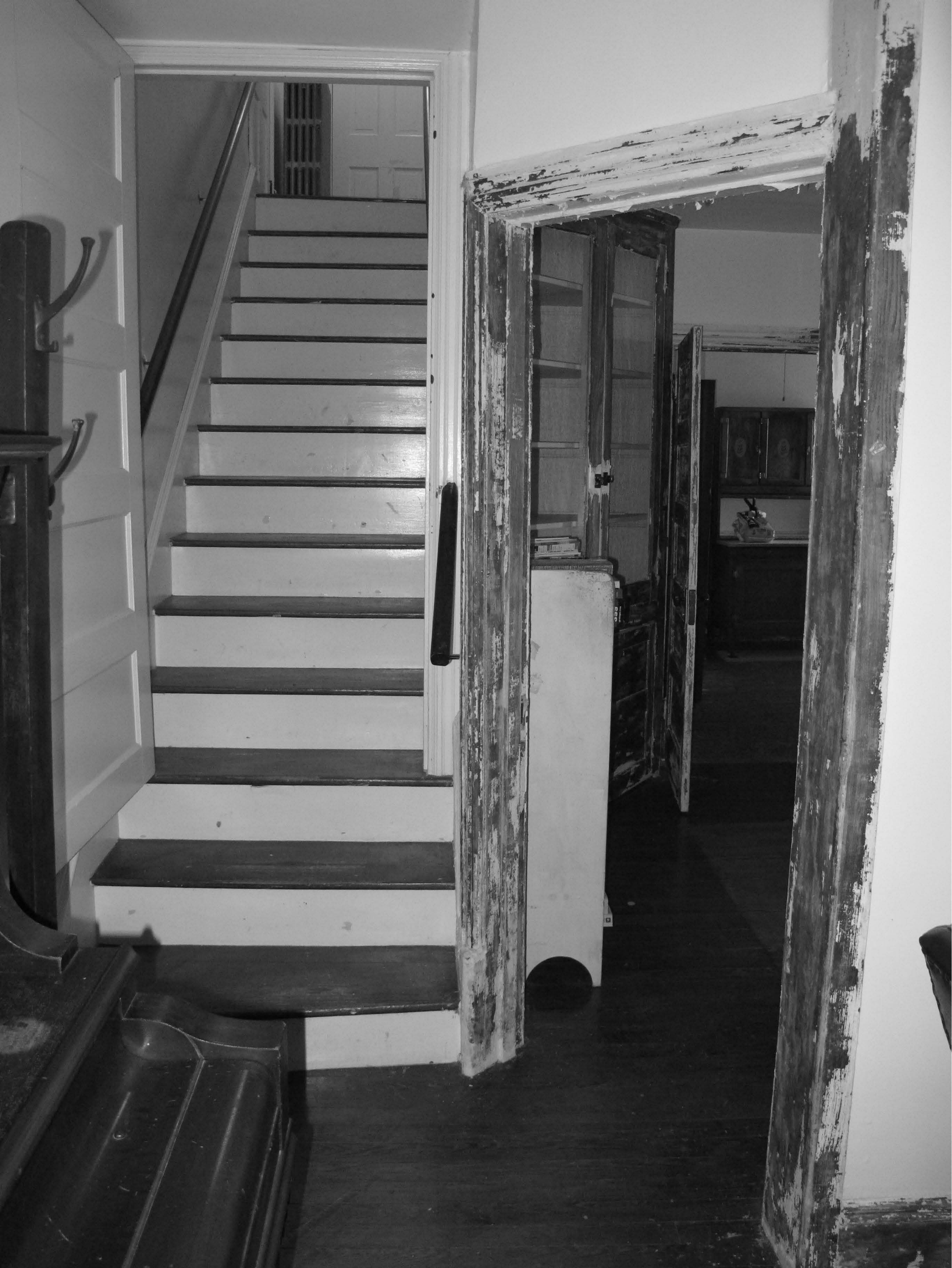
Cox-Phillips-Mitchell Agricultural Complex, New Castle County, DE Interior, first floor, Period I, view of room with staircase to second floor hallway, looking northeast
