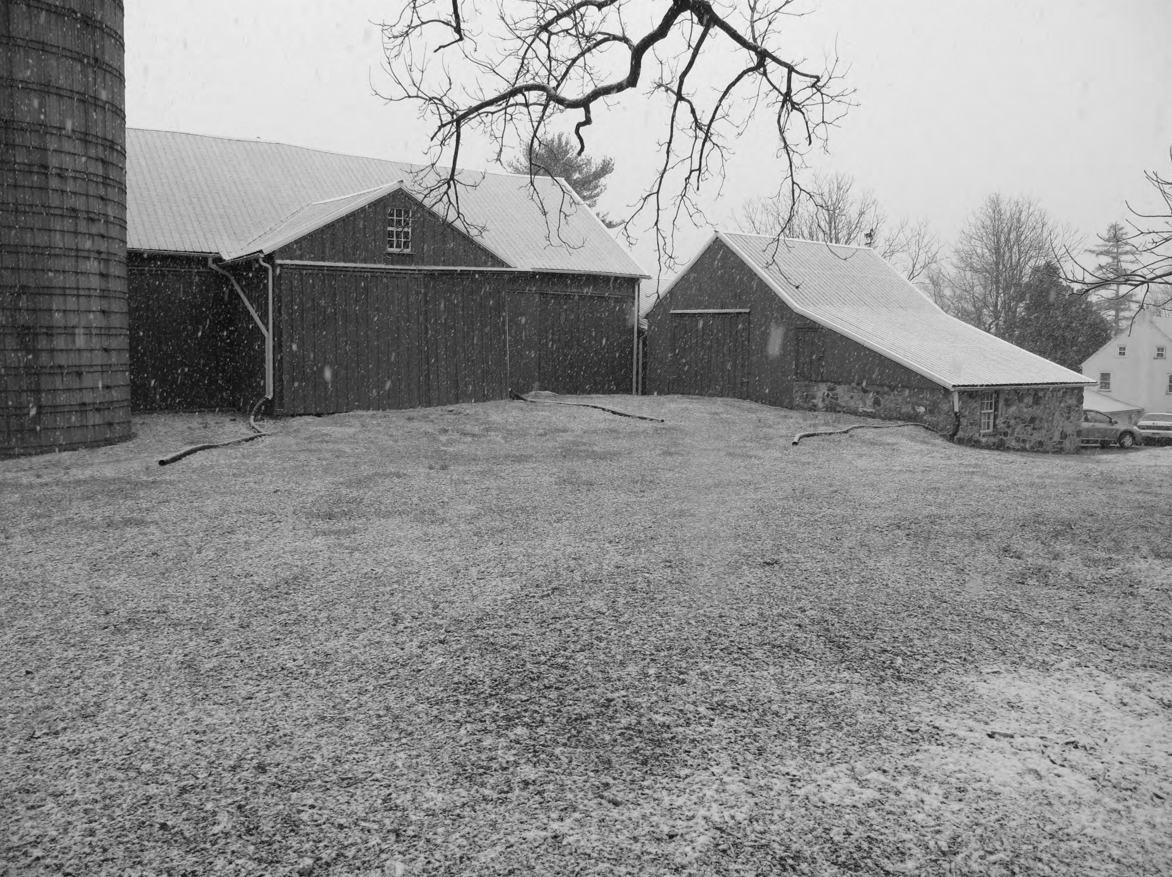
Cox-Phillips-Mitchell Agricultural Complex_New Castle County_DE Perspective view showing dairy barn, stable, and house looking southwest
