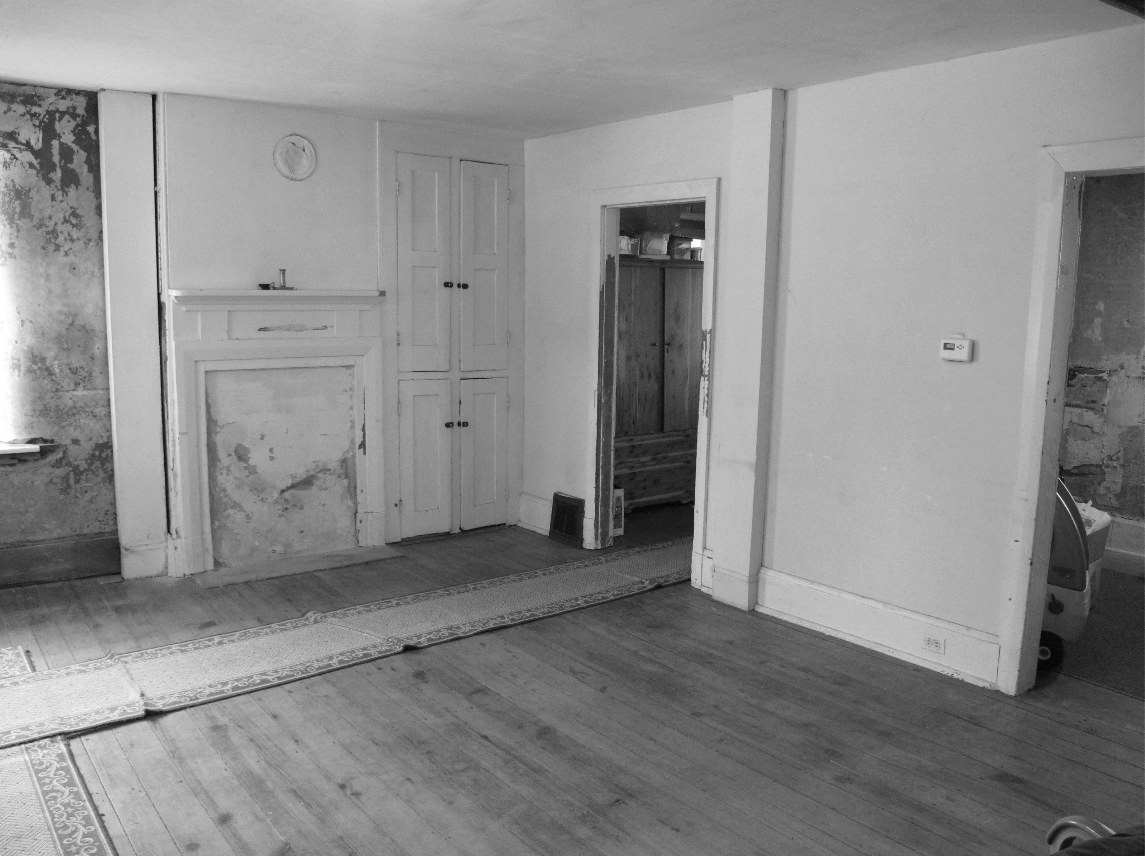
Cox-Phillips-Mitchell Agricultural Complex_New Castle County_DE interior, first floor, Period IV, view of southwest and southeast walls showing Greek Revival trim
