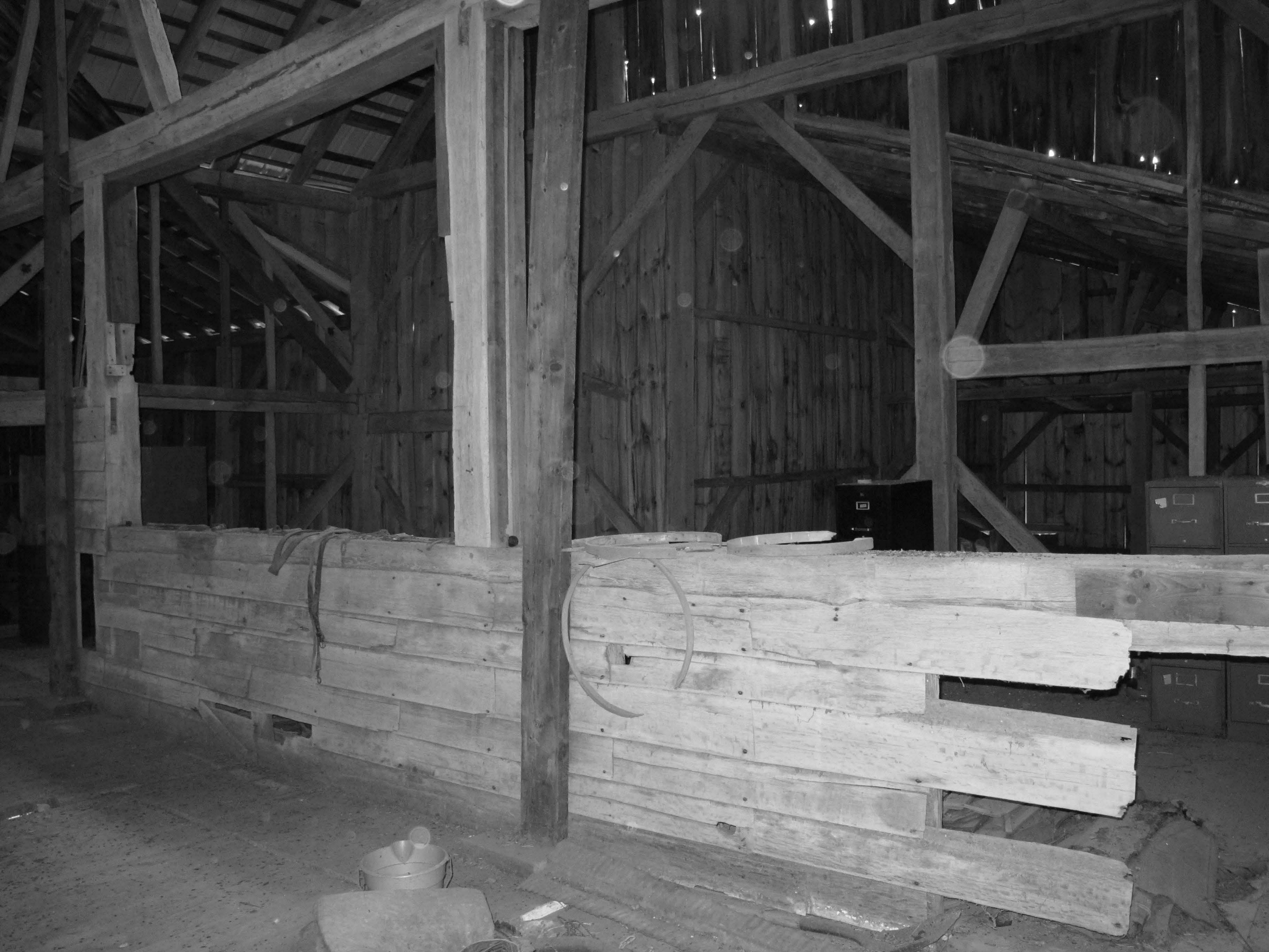
Cox-Phillips-Mitchell Agricultural Complex_New Castle County_DE Dairy barn interior upper level-threshing floor, riven clapboards looking south
