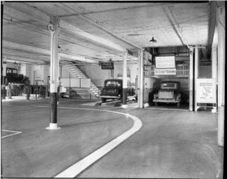
First Floor interior garage space at north end of first floor in 1933. Photo courtesy Bostwick-Frohardt Collection at Durham Museum
