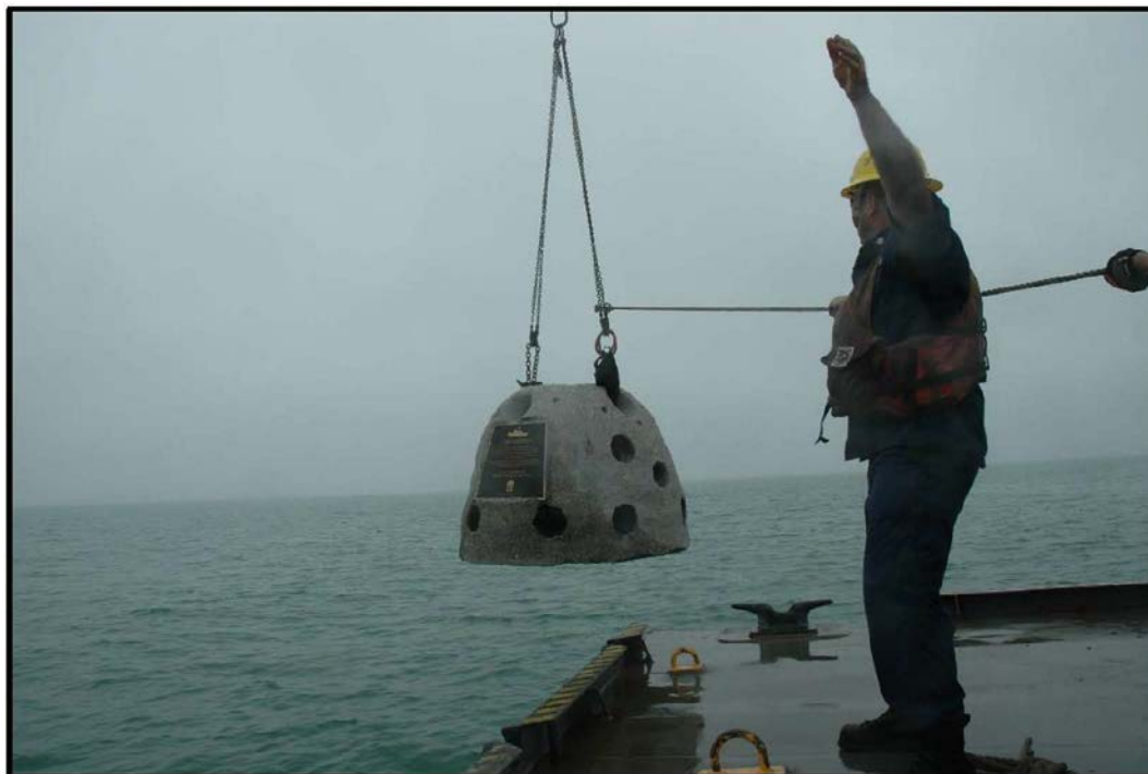
Figure 6. Concrete monument being deployed at the site (Florida Aquarium photo).
