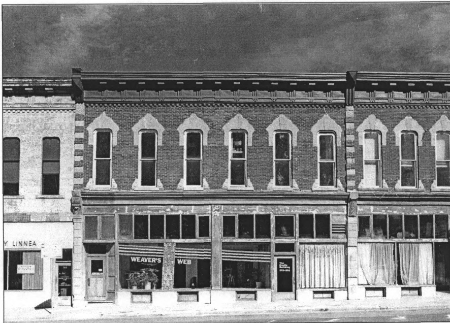
Figure 1: 1976 photo showing 516-518 and 520 East Grand, view north. Note the surviving basement windows, set into the bases of the ground floor display areas and storefront base plates. Note the Society Linnea sign on 518 East Grand, at the far left (courtesy of Tim Rypma)
