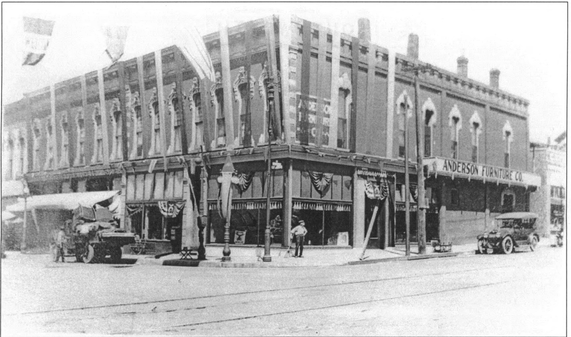
Figure 37: Anderson Furniture Company. Shriners' Convention Decorations, c.1920-21 (Courtesy Jim Boyt) Note also that the rearmost five stone hoods above the East Sixth Street have all been cut back to the wall plane, in preparation for the scored stucco covering that was to follow
