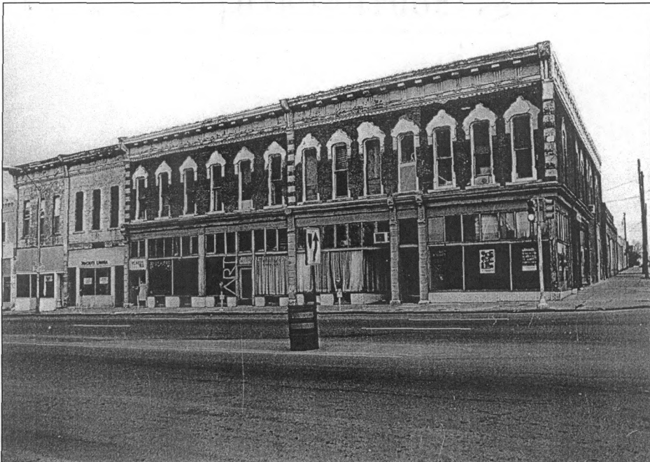
Figure 24: Buildings' appearance following stucco removal, c.1977, view northwest (Courtesy James Boyt)
