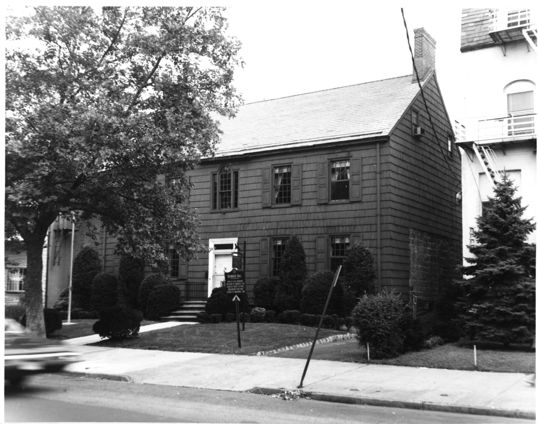
Elias Boudinot House, "Boxwood Hall," Elizabeth, New Jersey
