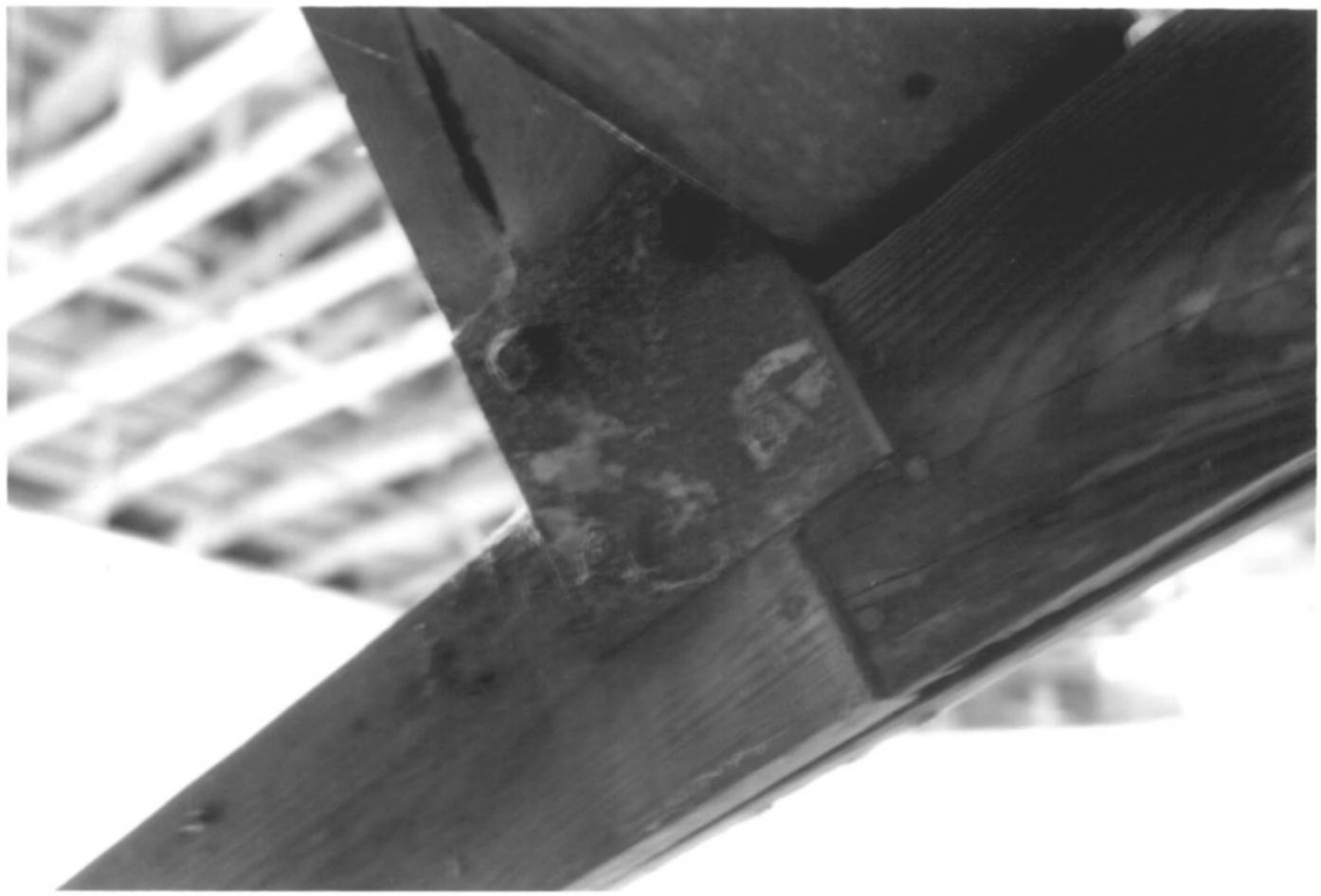
6. Interior of gym, detail + truss plates
