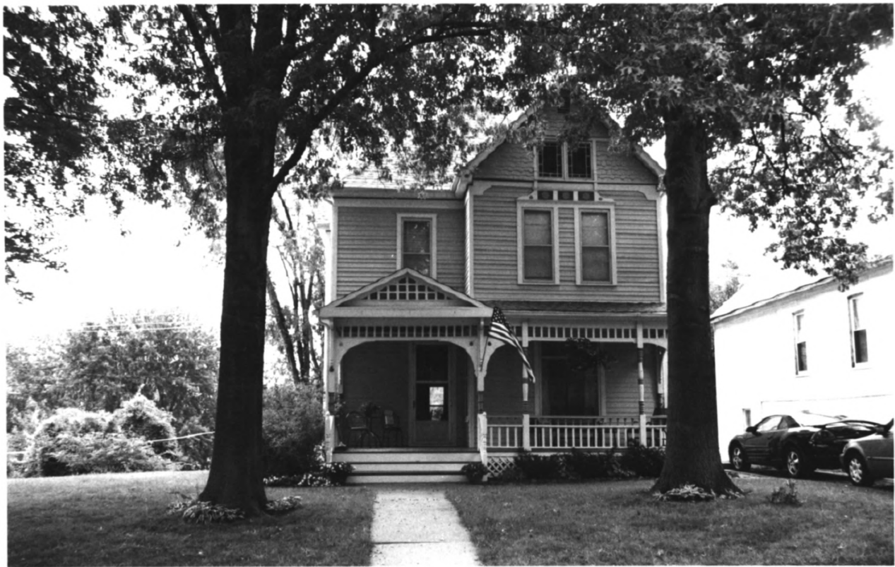
Janson House Atchison Co., Kansas
