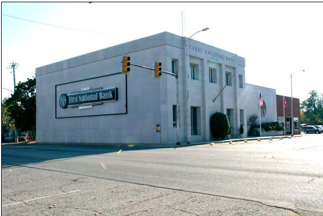
Photo 12. 300 Block (West), Public Square from Main Street; facing southwest.
