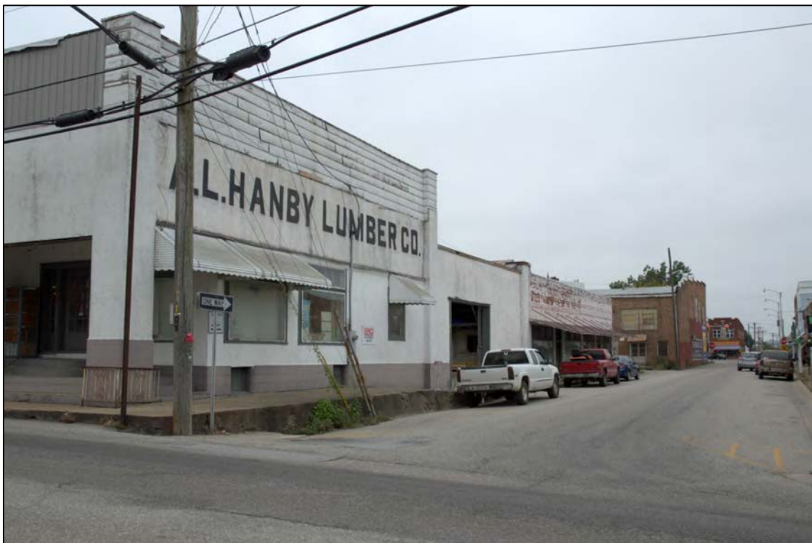
Photo 28. Southern side of East Church Street from North Springfield Street; facing southwest.
