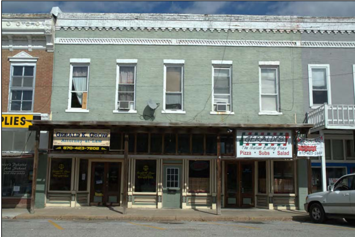
Photo 46. Perkins Dry Goods at 203/204 Public Square; facing east.
