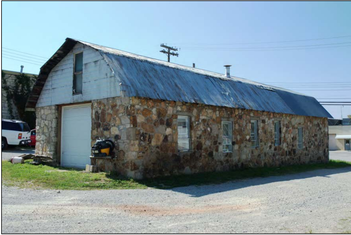
Photo 52. Former Blacksmith Shop at 111 Spring Street; facing southwest.
