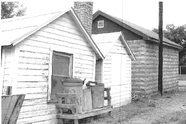
East elevations of garage (noncontributing), coal shed (contributing) and laundry (contributing) Photo taken June 2003 by Steve Allison.
