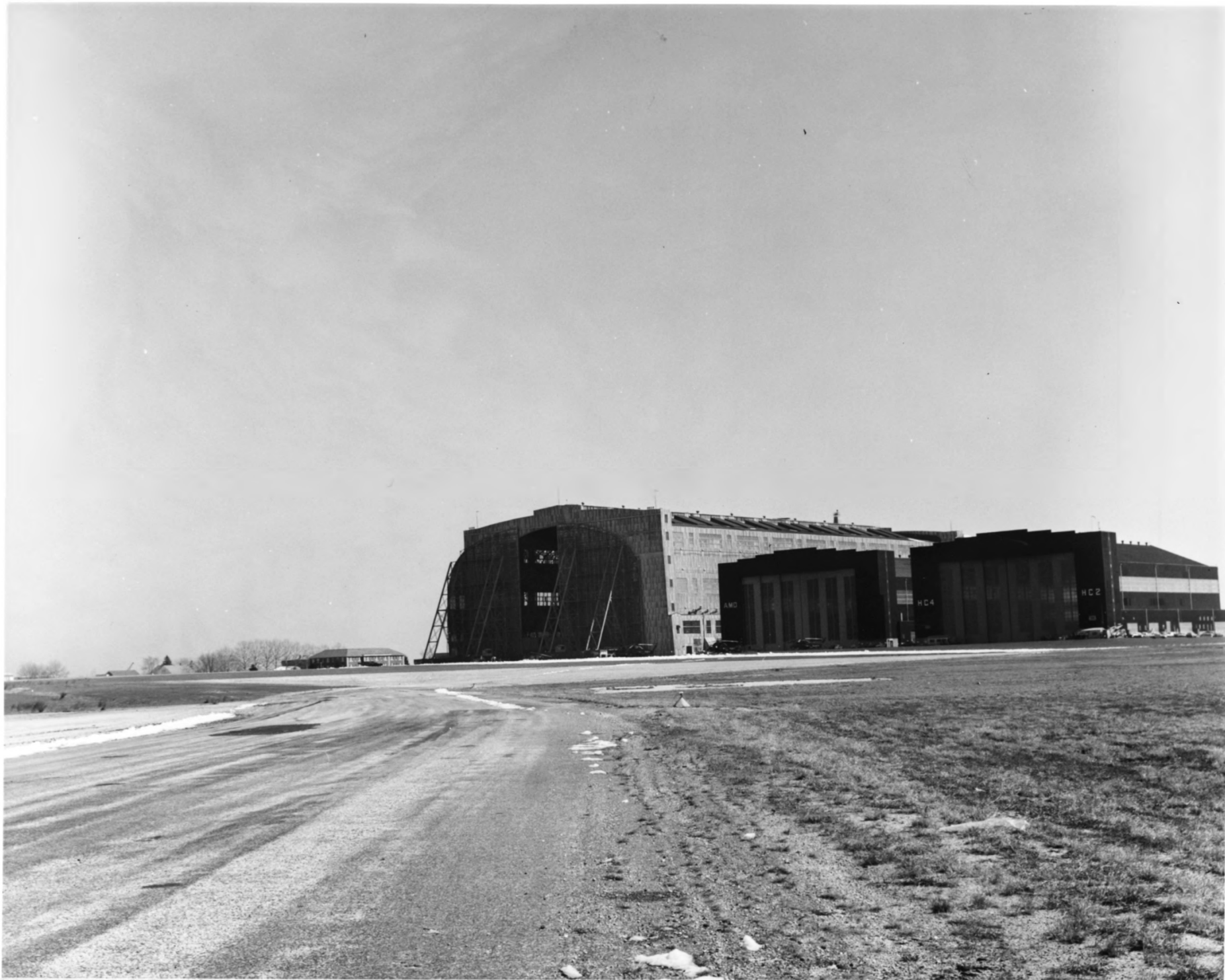
Hangar No. 1, Lakehurst Naval Air Station, New Jersey
