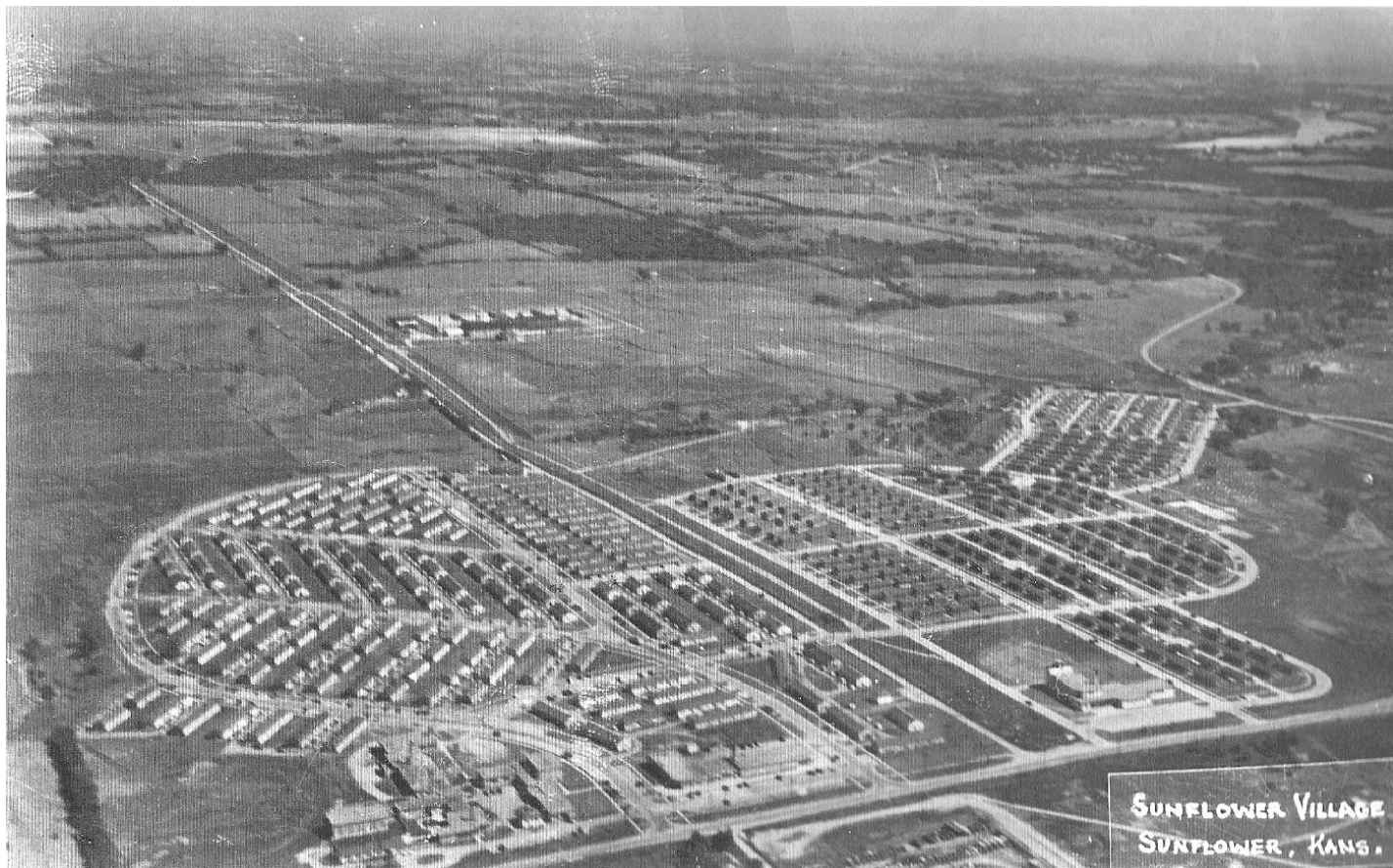
Figure 11 at right – Aerial view of Sunflower Village with 2 nd and 3 rd additions in place c.1945 (courtesy of David Rhodes, Clearview Village, Inc.)
