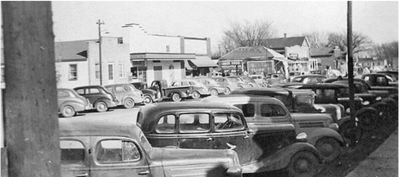
Figure 22 – 1942 Street Scene in the town of DeSoto whose population doubled in one year. (“Sunflower Ammunition Factory Caused Population Explosion in De Soto,” Lawrence Journal World , January 4, 2010). When plant construction began the government focused on transportation both for workers and the eventual product that would require rail and road improvements. A rail spur in DeSoto was completed in mid-July 1942 allowing construction to speed up with the faster transit of materials. 81 Bus companies added routes synced to Sunflower shifts to link Eudora and De Soto with Lawrence and Kansas City. 82
