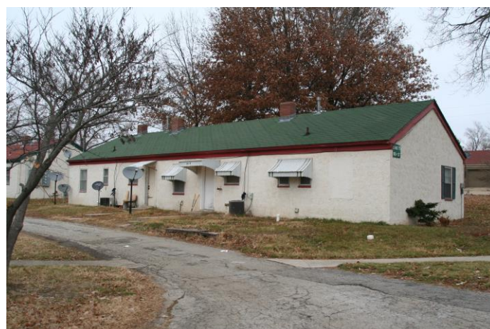
Figure 13 – Current views of residential buildings with exteriors dating to early 1970s remodeling by Hansen including: stucco finish on concrete block walls, porch added at front entry and shutters installed at windows. Some homes retain the metal slat awnings also installed in the early 1970s. (Spencer December 2013 and March 2014)
