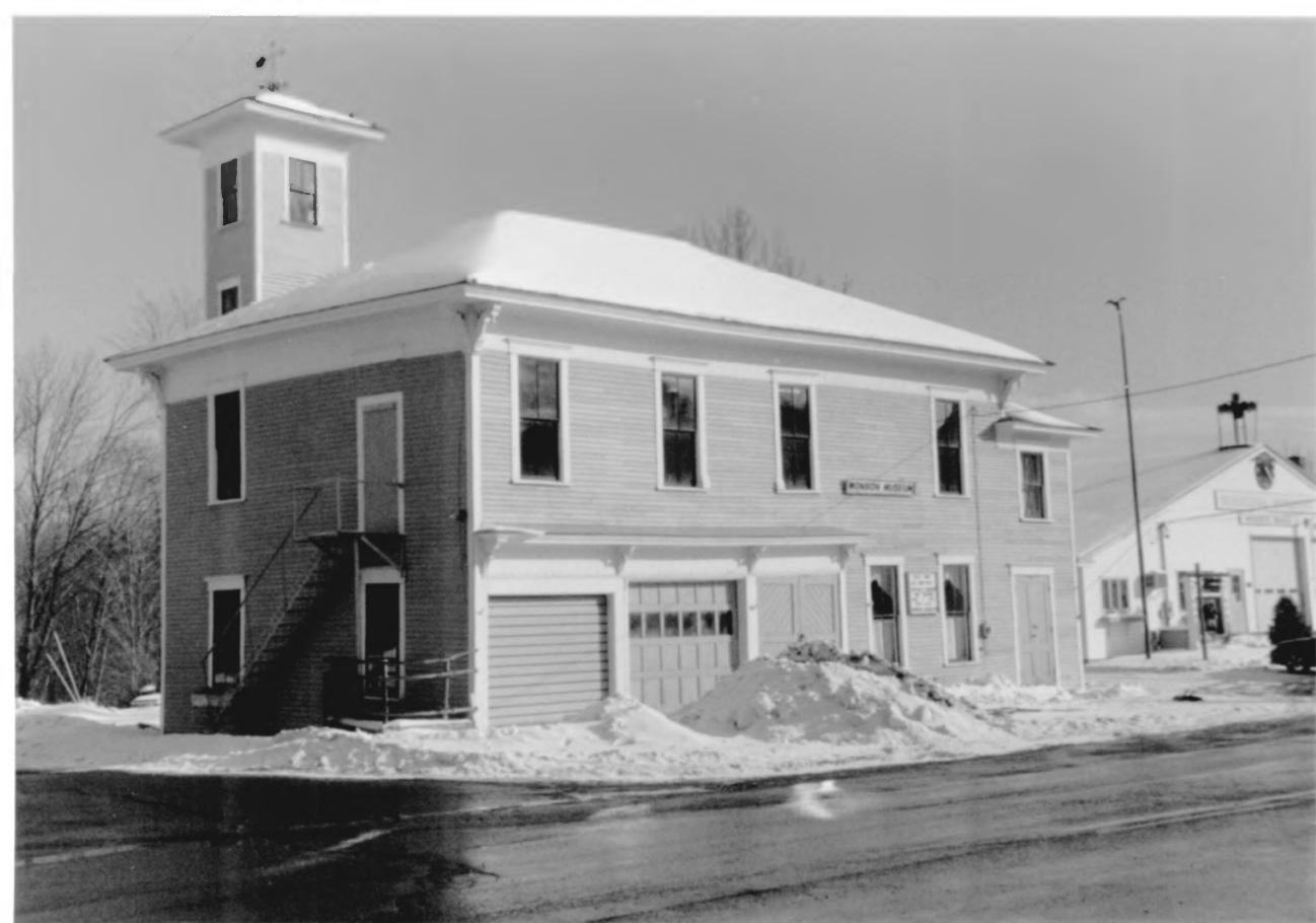
MONSON ENGINE HOUSE (FORMER); PISCATAQUIS CO., ME
