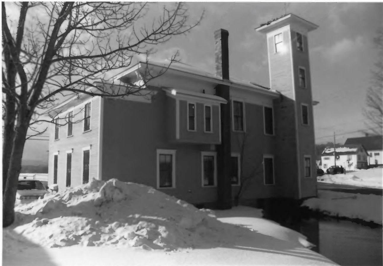
MONSON ENGINE HOUSE (FORMER); PISCATAQUIS CO., ME
