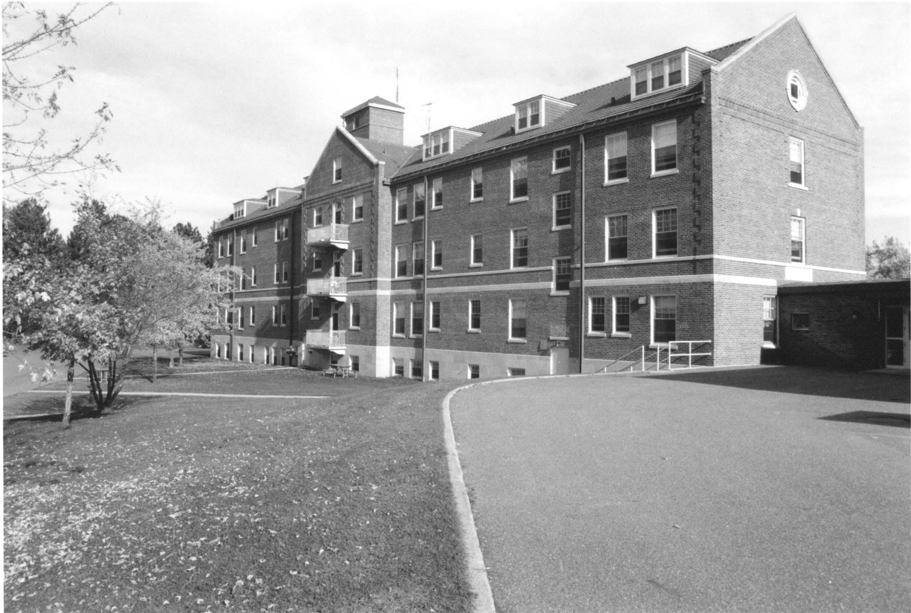
MINNESOTA STATE SANATORIUM FOR CONSUMPTIVES # 3 INDIAN BUILDING (REAR FACADE)
