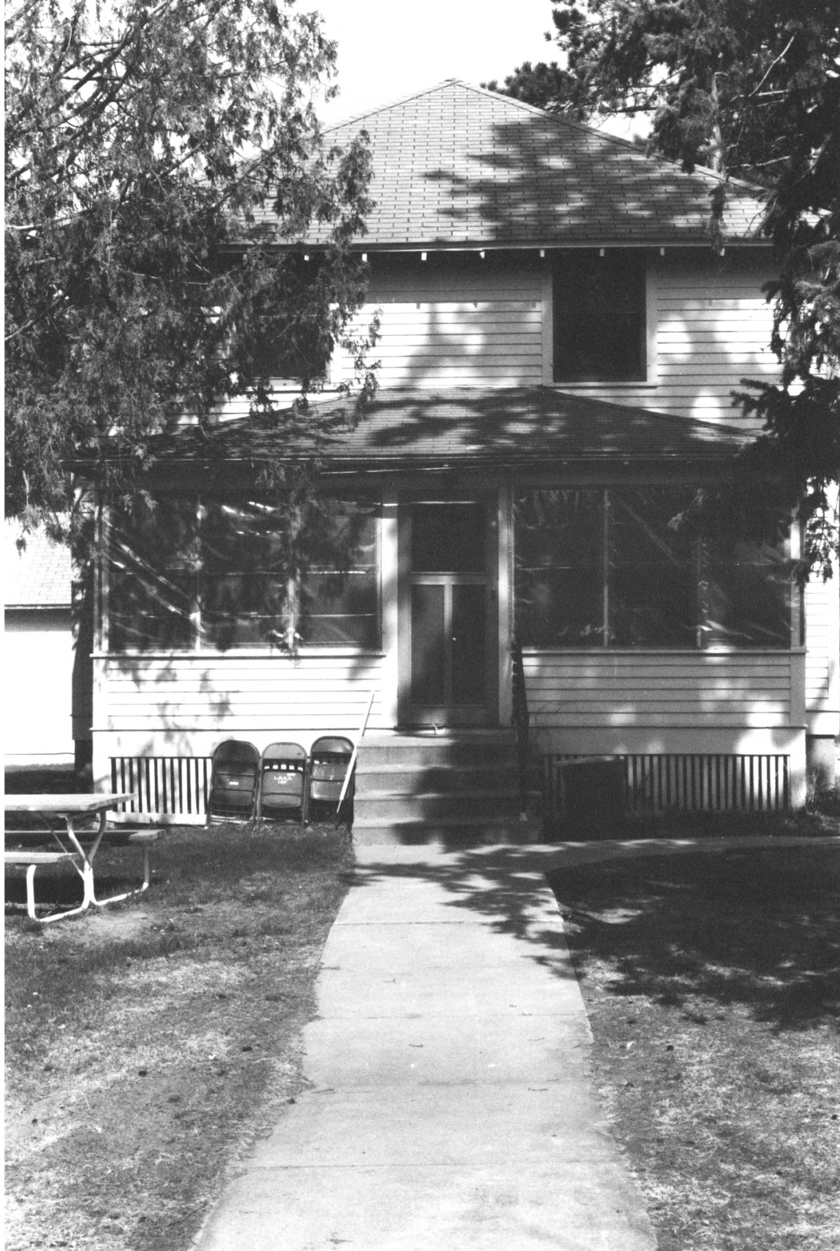
MINNESOTA STATE SANATORIUM FOR CONSUMPTIVES #10 ENGINEER'S COFFAGE 013032-0
