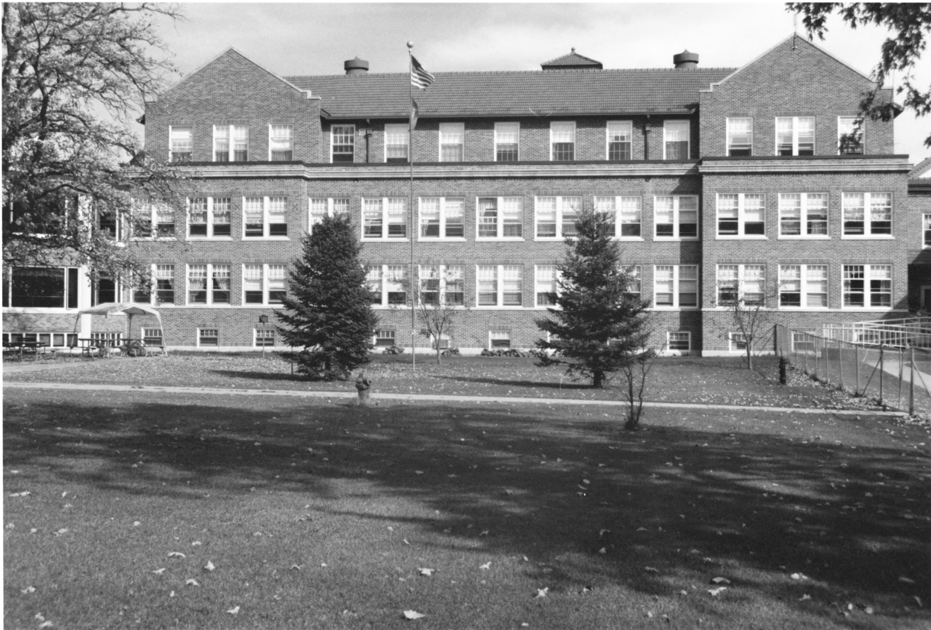
MINNESOTA STATE SANATORIUM FOR CONSUMPTIVES # 7 INFIRMARY II CASS CO., MN 012665-17
