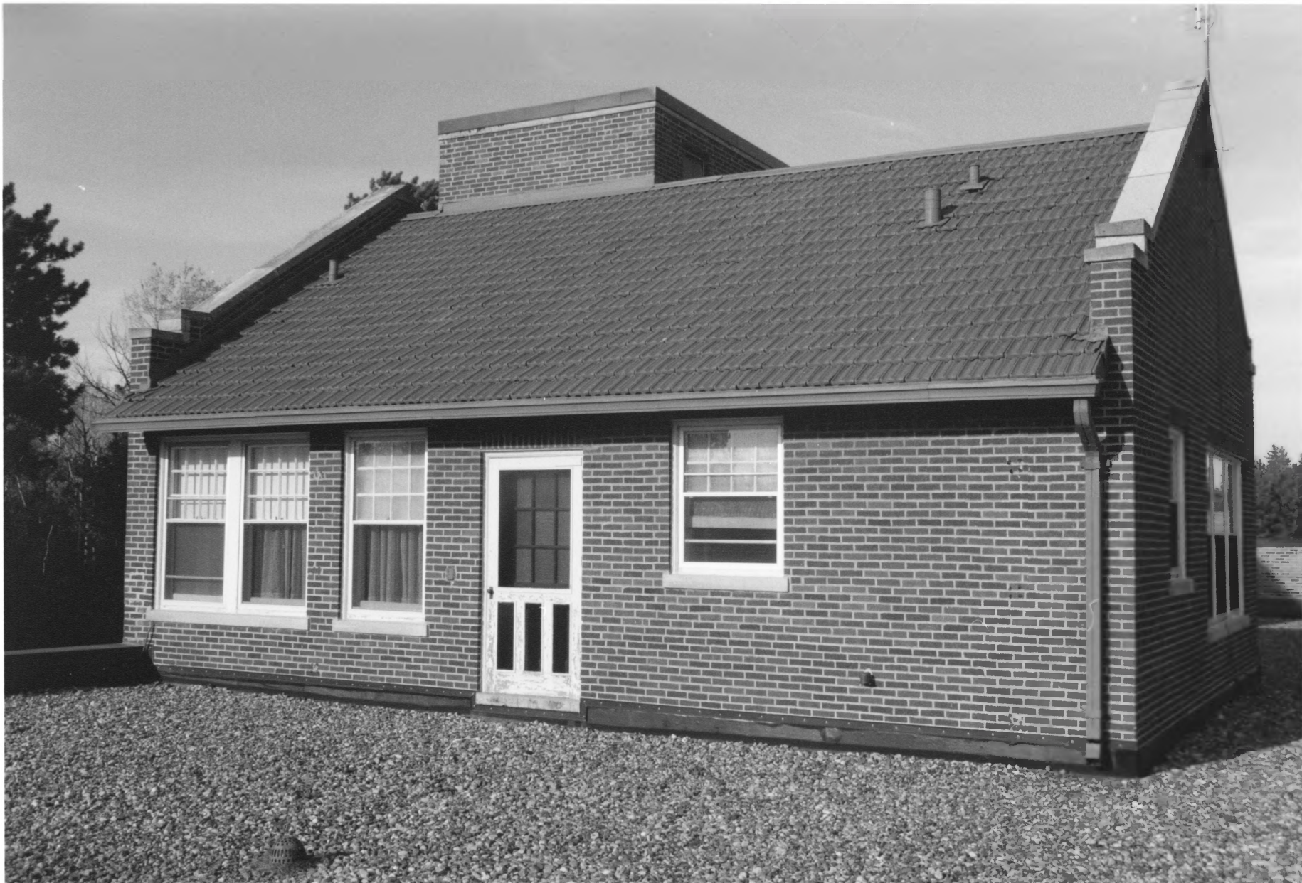
MINNESOTA STATE SANATORIUM FOR CONSUMPTIVES #6 "ROOF HOUSE" ON 3 rd STORY OF INFIRMARY I CASS CO., MN 012758-7
