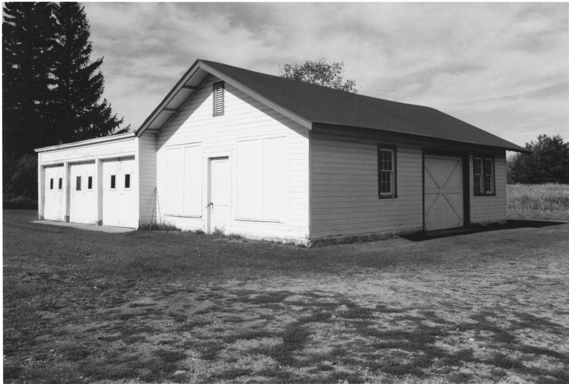
MINNESOTA STATE SANATORIUM FOR CONSUMPTIVES #25 GARAGE/SHOP CASS CO., MN 012666-9
