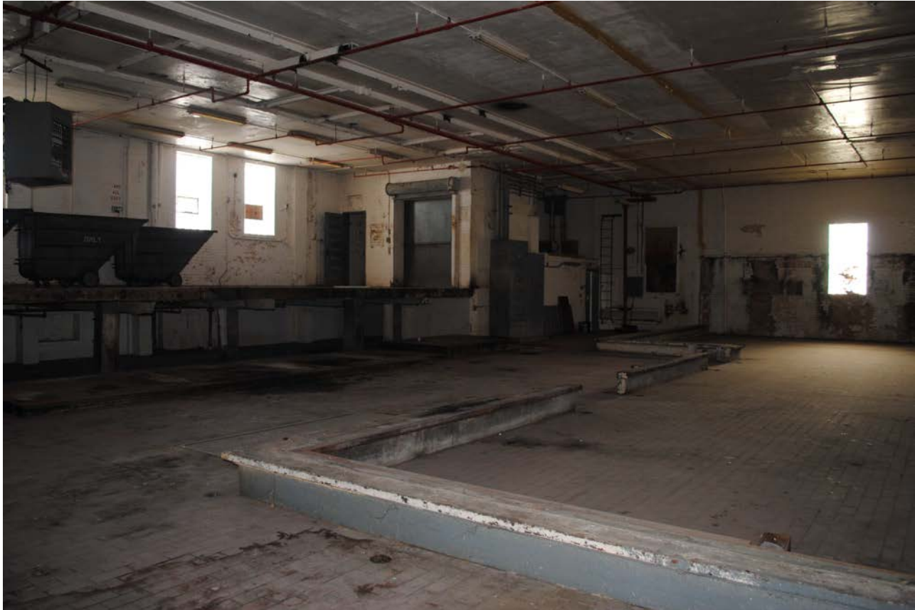
Figure 14: Third Floor, Block C, historic mixing room; note freight elevator and raised platform with flour bins. Source: Lauren Rieke, 2015.
