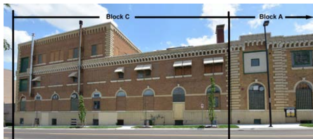
Figure 7: West Elevation, Block C and part of Block A. View east.
