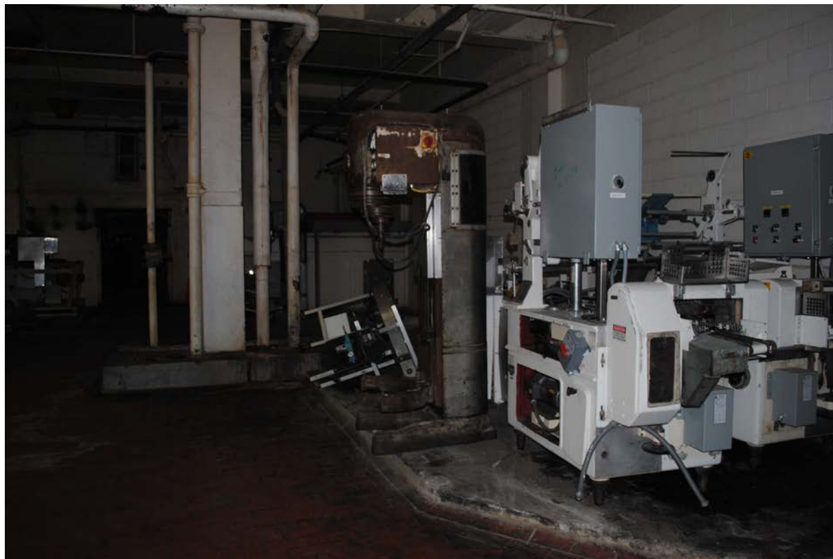
Figure 12: First Floor, Block A, historic oven room; note slightly raised concrete platforms and extant machinery. Source: Lauren Rieke, 2015.
