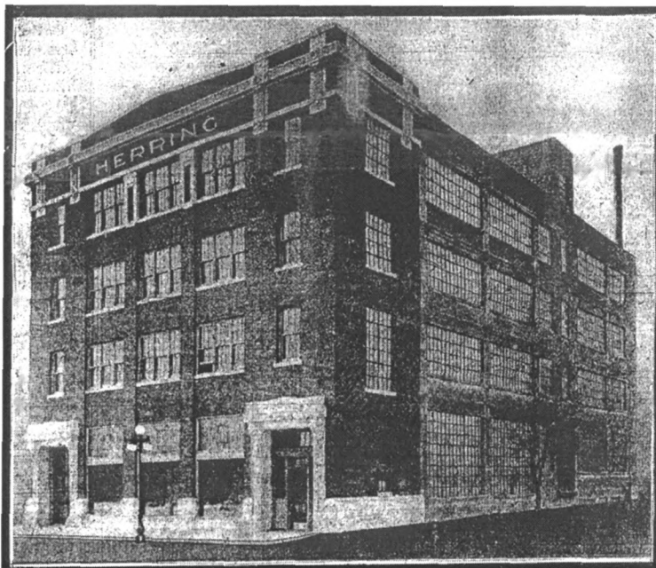
Finished building ( Register & Leader , March 2, 1913)
