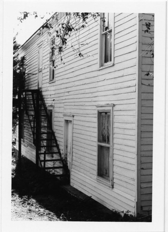
View of N Exposure Lecompton Constitution Hall
