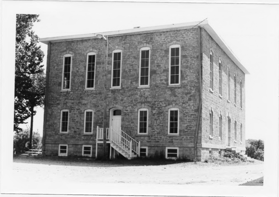
Lane University building - S & W exposures - built on foundation of unfinished capitol
