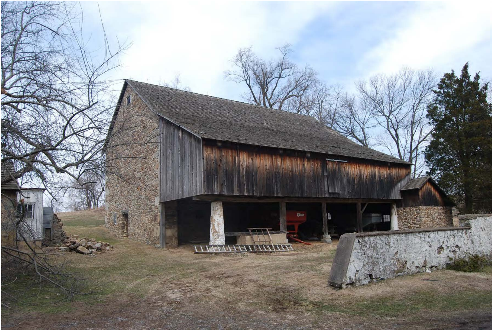
Photo 15 of 20. Levi Murray Barn [27], facing northeast from Nantmeal Road. The cylindrical piers under the forebay were a common feature in this region.
