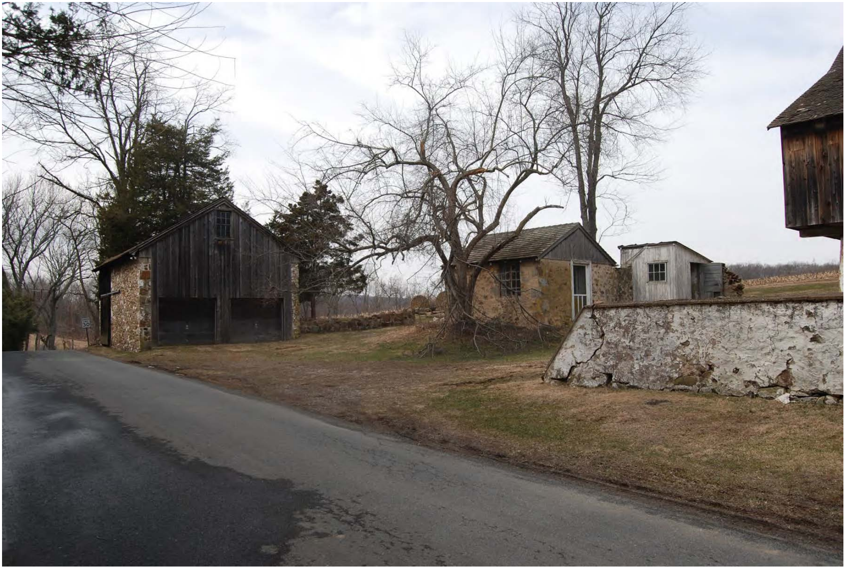
Photo 20 of 20. Outbuildings associated with the Levi Murray Barn [27], facing northwest from Nantmeal Road.
