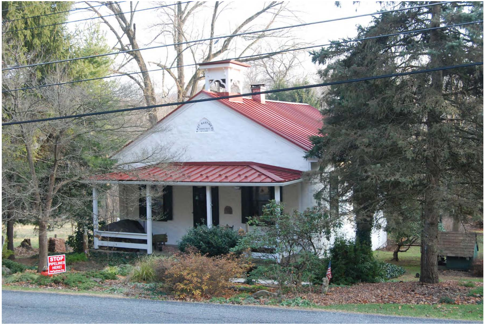
Photo 14 of 20. Nantmeal Village Schoolhouse [78], facing south from the Friends Burial Ground on the north side of Fairview Road.
