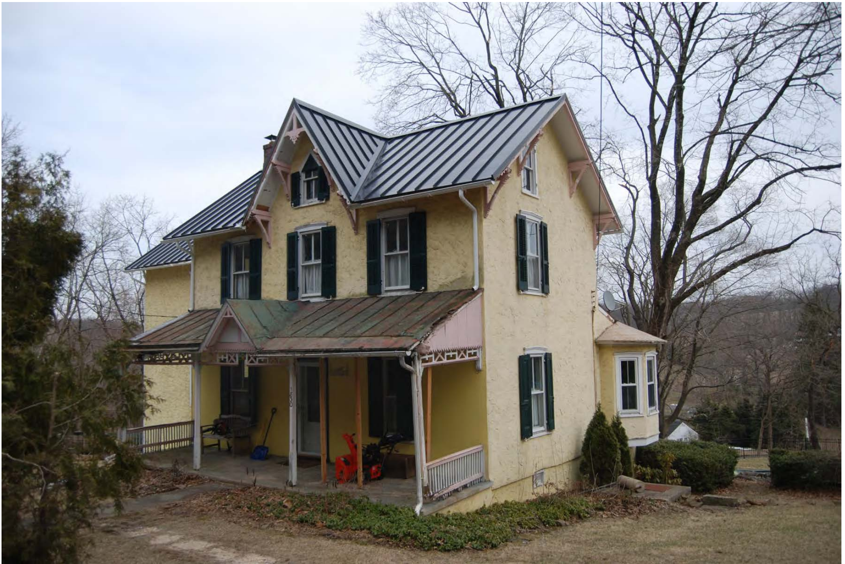
Photo 10 of 20. William Evans House [77], facing south from Fairview Road.
