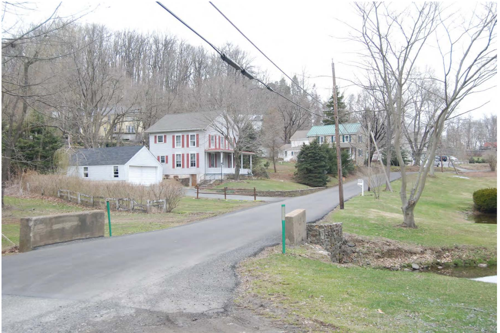
Photo 4 of 20. View of the south central portion of the district, facing north up Nantmeal Road. Resources on the left are the John Loomis House (frame, 80) and the Ann Hall House (stone, 79), right.
