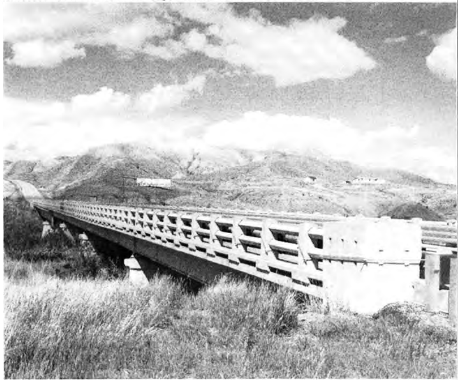
Photo 0002. Marias River Bridge. west elevation. View to the northeast
