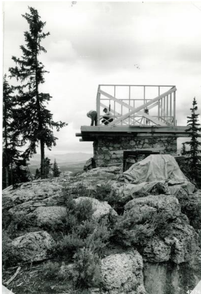
Lookout under construction in 1942 (USFS).
