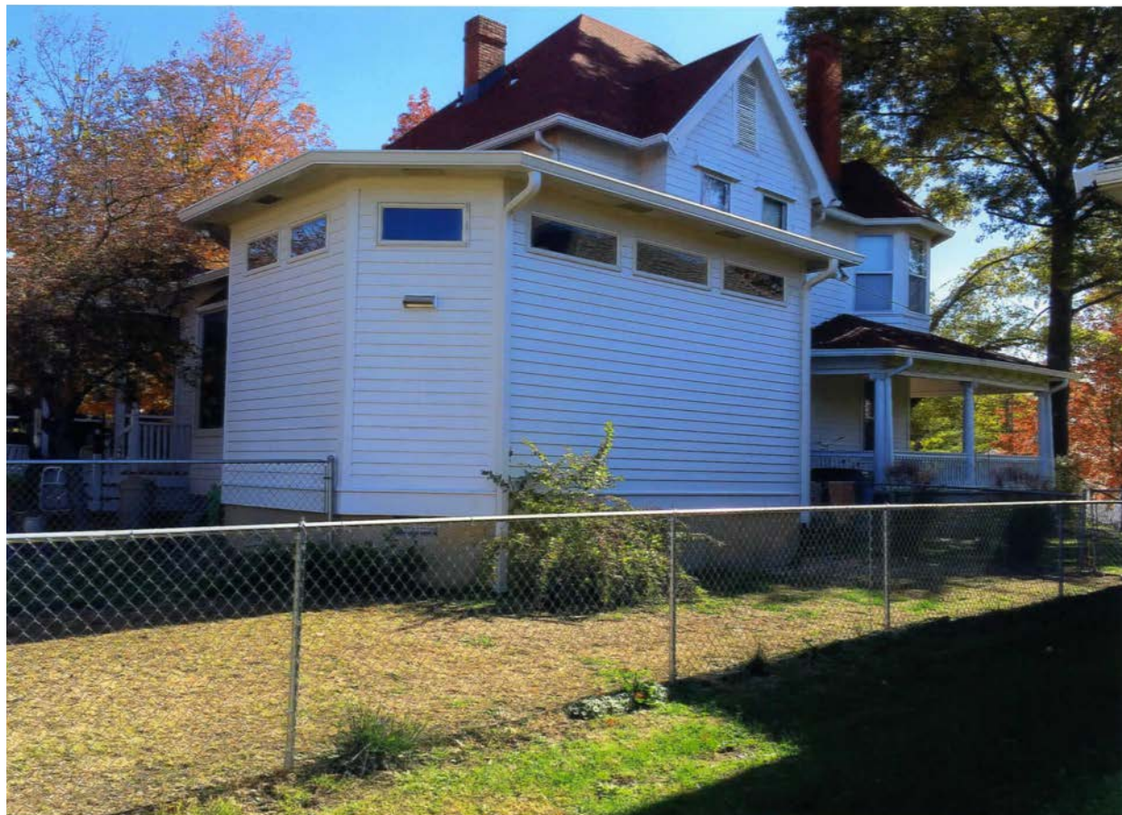
Figure 4. Image of the west elevation, shows the 2007 kitchen addition, c. 2014. Source: “George Wolz Residence Eligibility Assessment Form,” EAGY005.
