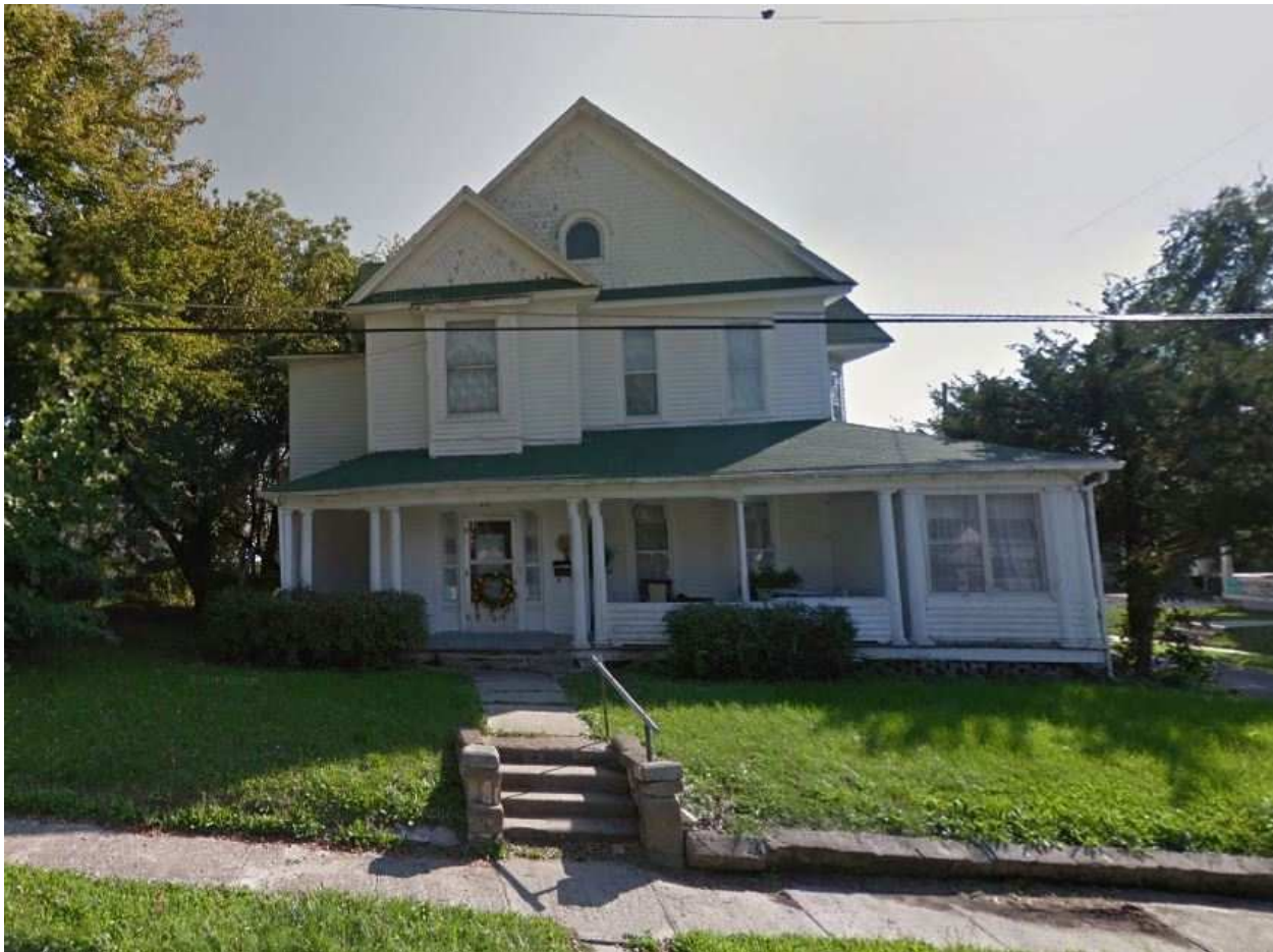
Figure 14: House at 312 West 12 th , Trenton. (Source Google, accessed 2/15/2018)
