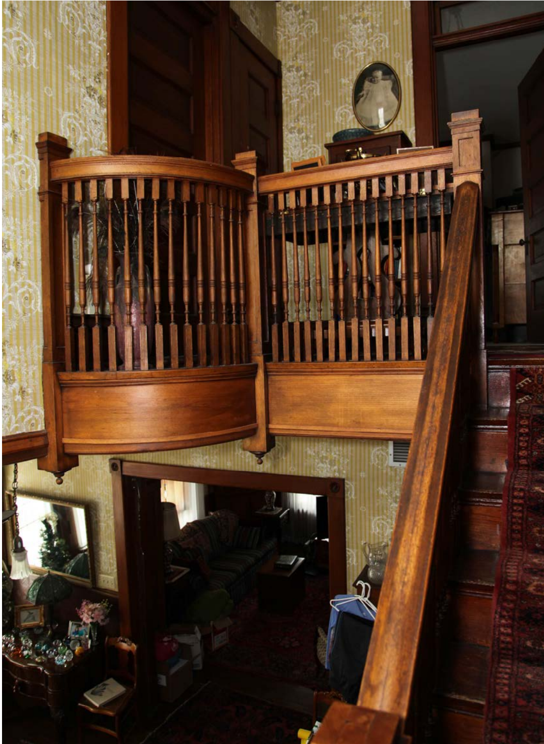
Figure 9. Stairs, c. 2015 Source: SHPO Staff Photos, taken April 2015.
