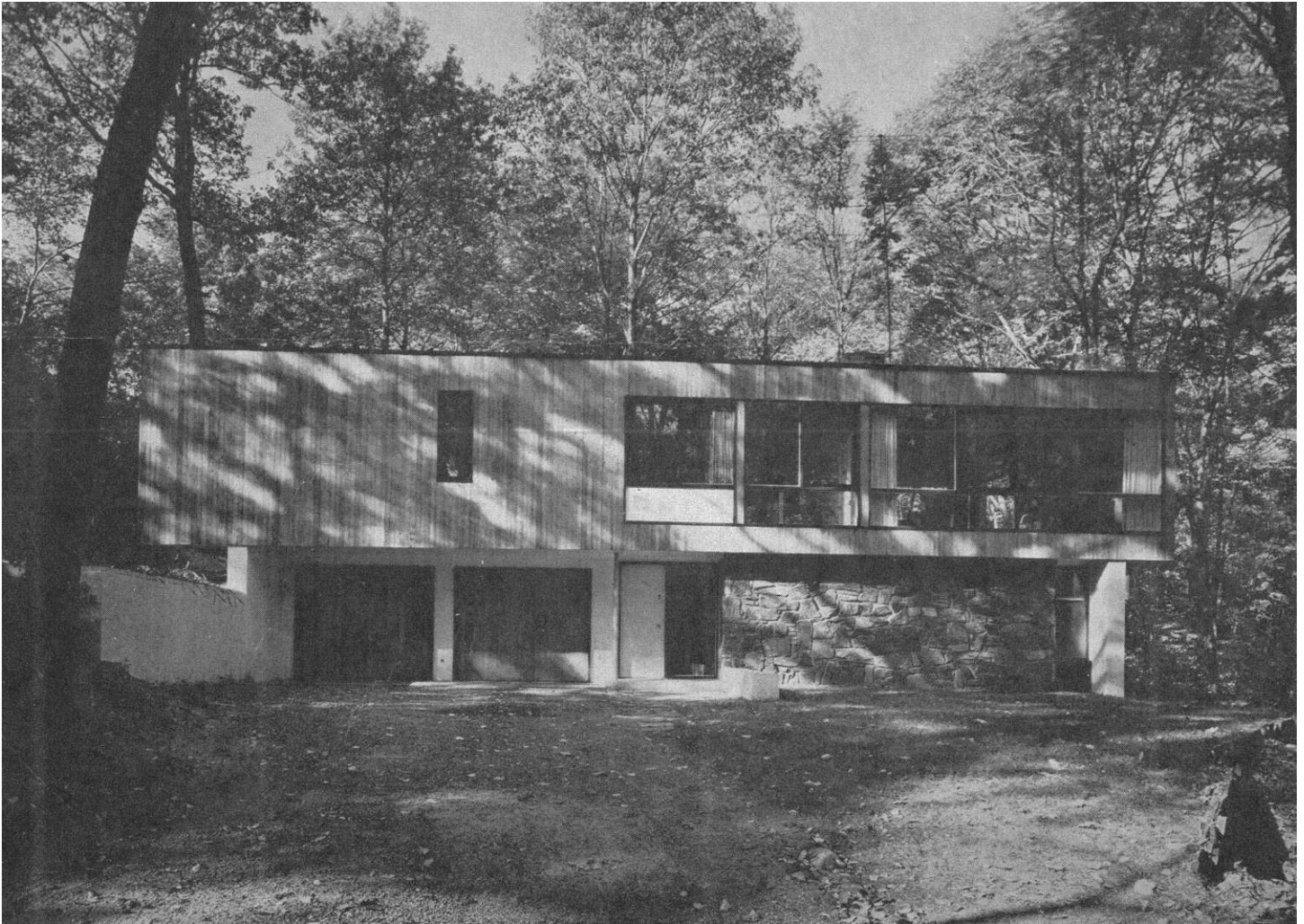
Façade, William Landsberg House, Architectural Record , 1953
