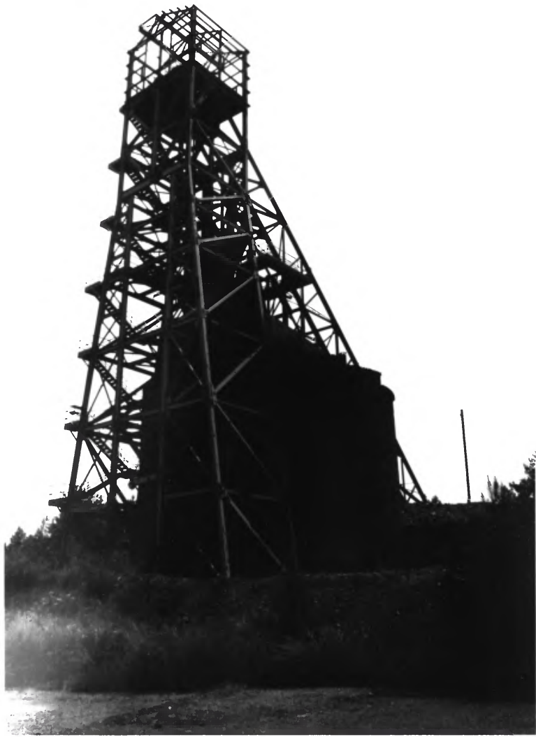
Central Headframe Polk County, TN
