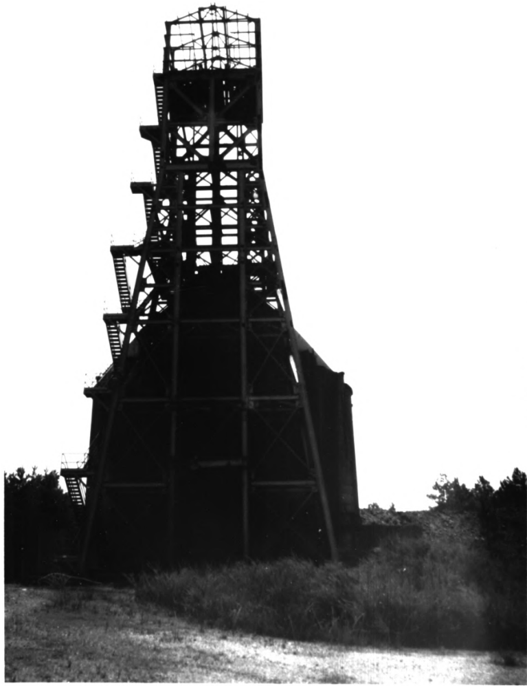
Central Headframe Polk County TN
