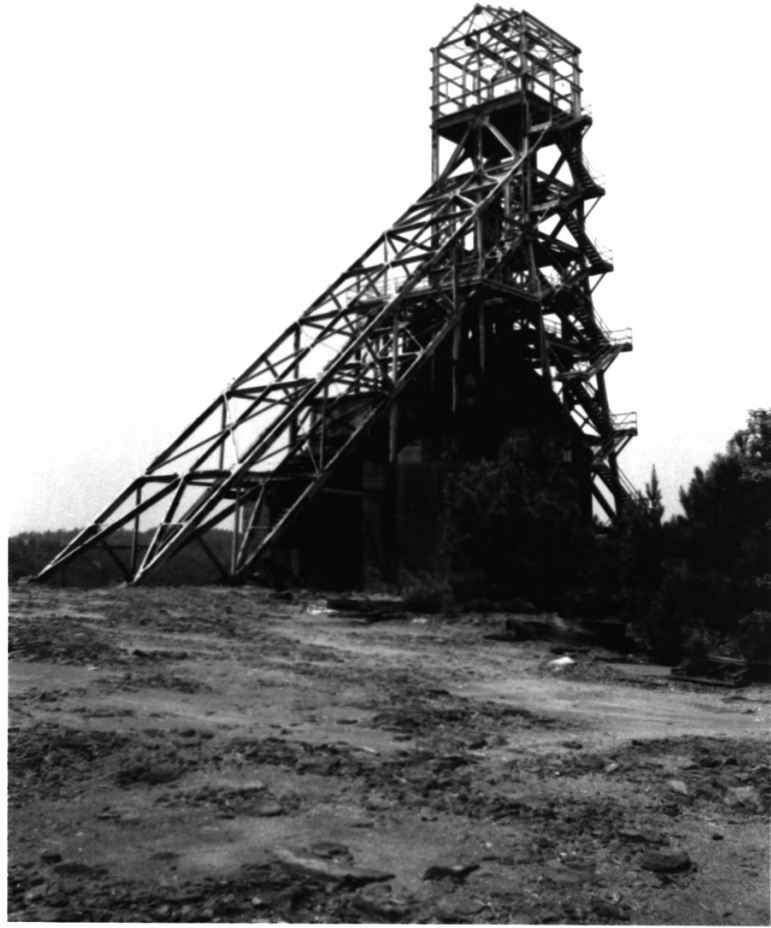
Central Headframe Polk County TN
