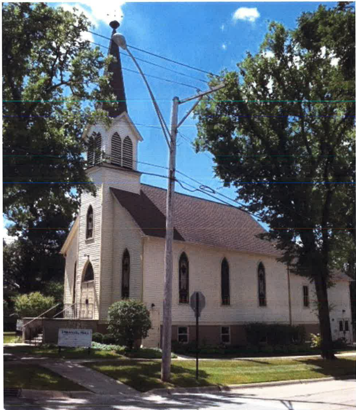
Figure 5: East (front) and north elevations
