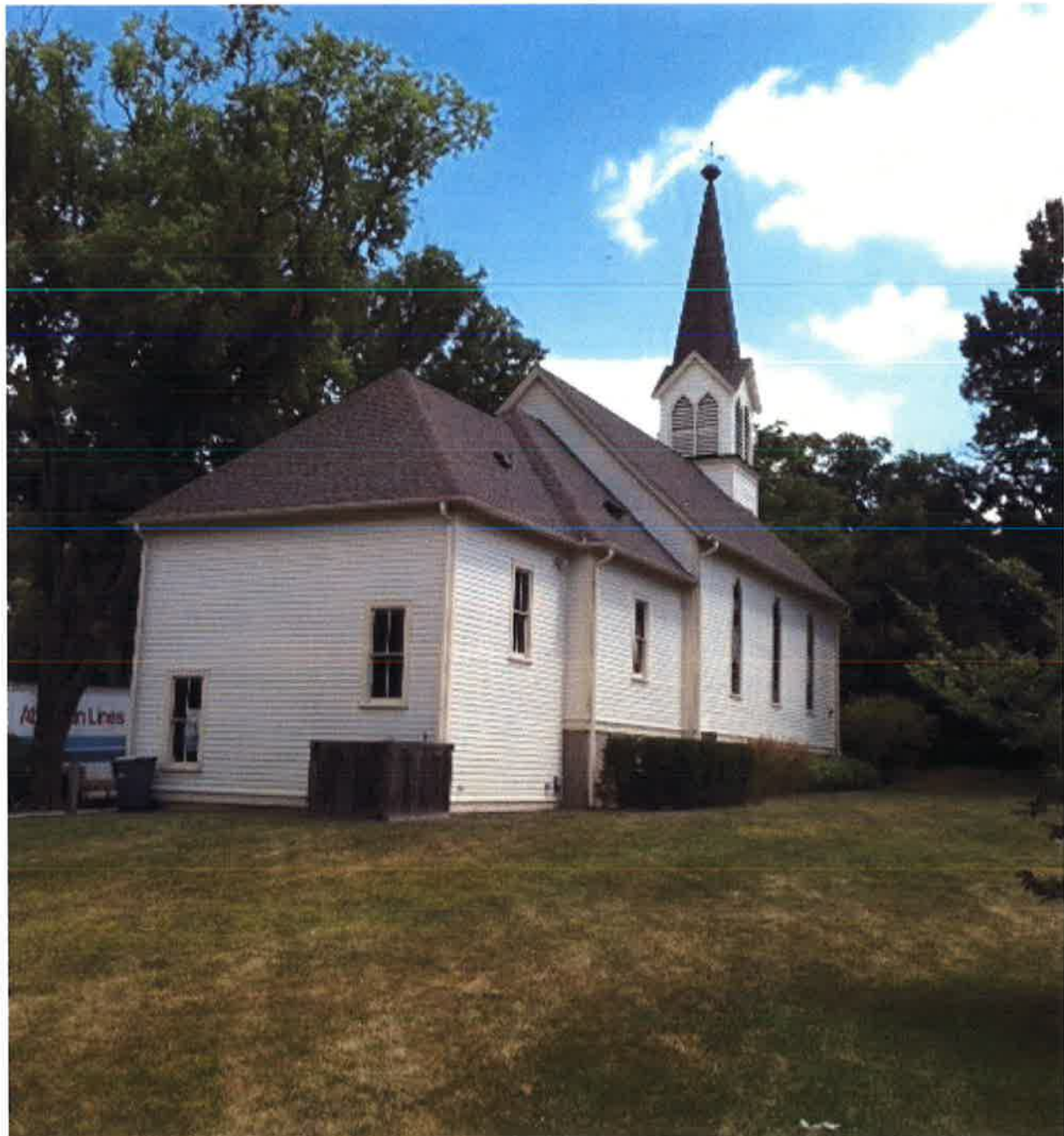
Figure 7: Rear addition on West elevation
