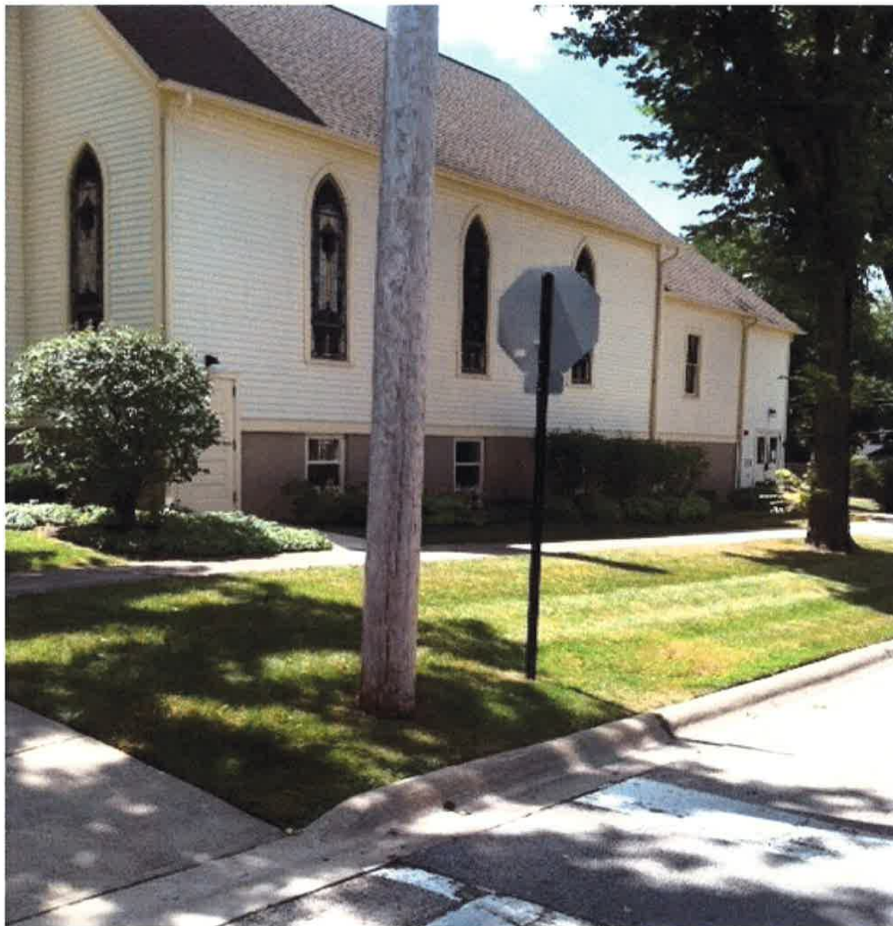
Figure 6: North elevation showing rear addition
