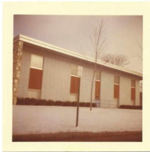
Figure 6: Franklin Park Medical Center in 1962 showing the original blue color of block walls (Photograph courtesy of Lenore Thomas)
