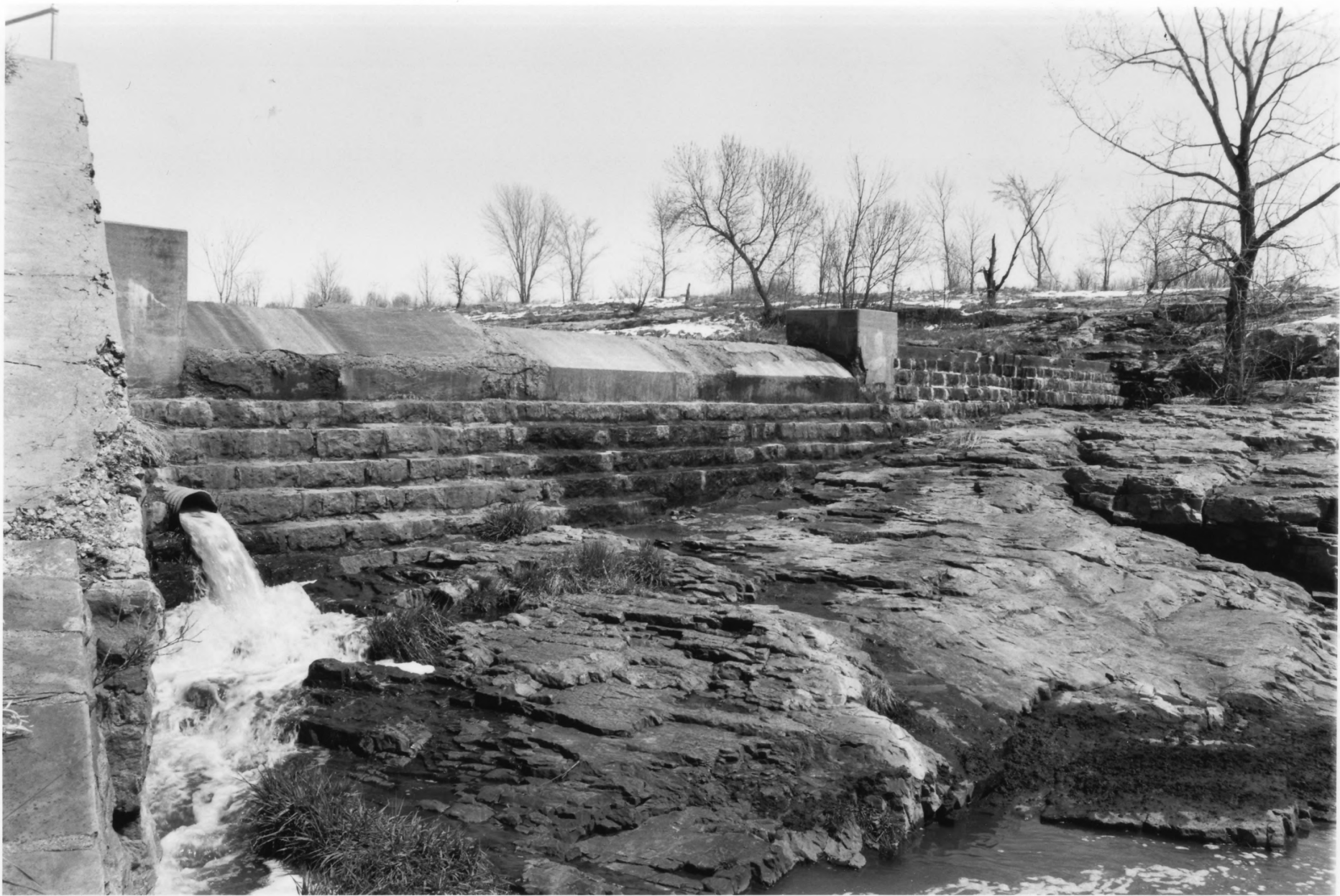
BLUE MOUNDS STATE PARK - UPPER DAM ROCK CO., MN STRUCTURE # 1 PHOTO I.D. 09724 # 9
