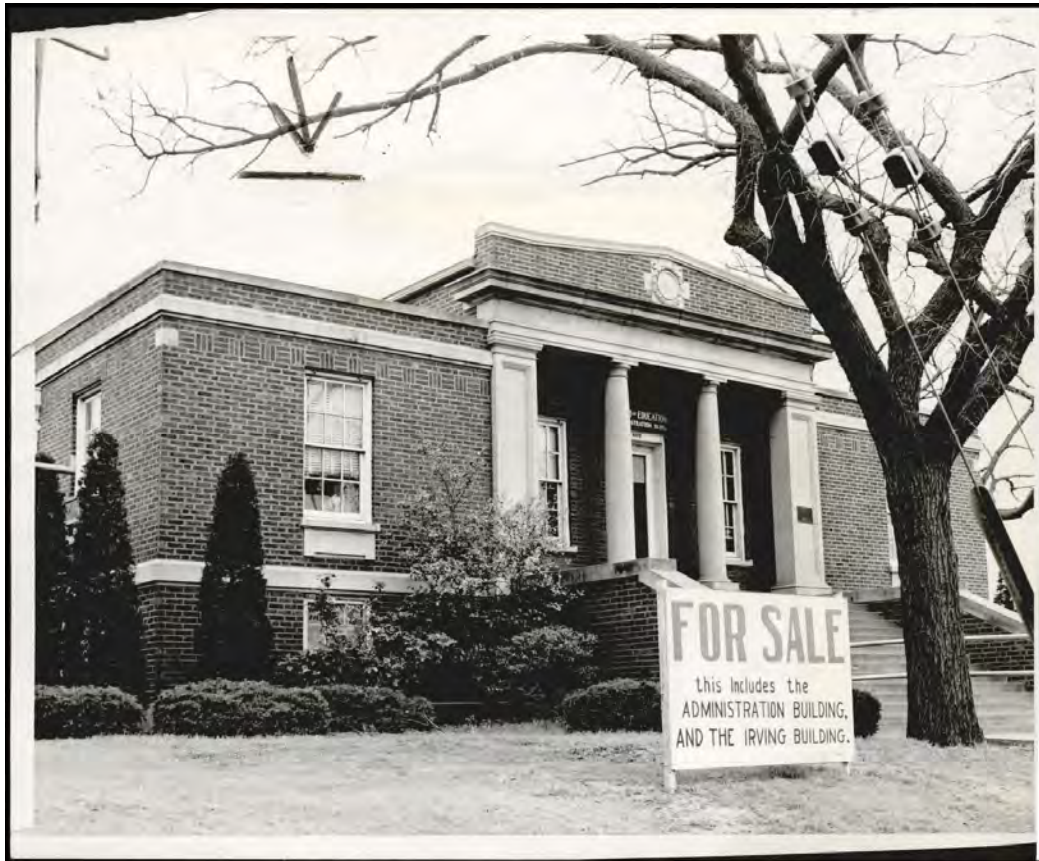
Photo #2: Oklahoma City Schools Administration Building
