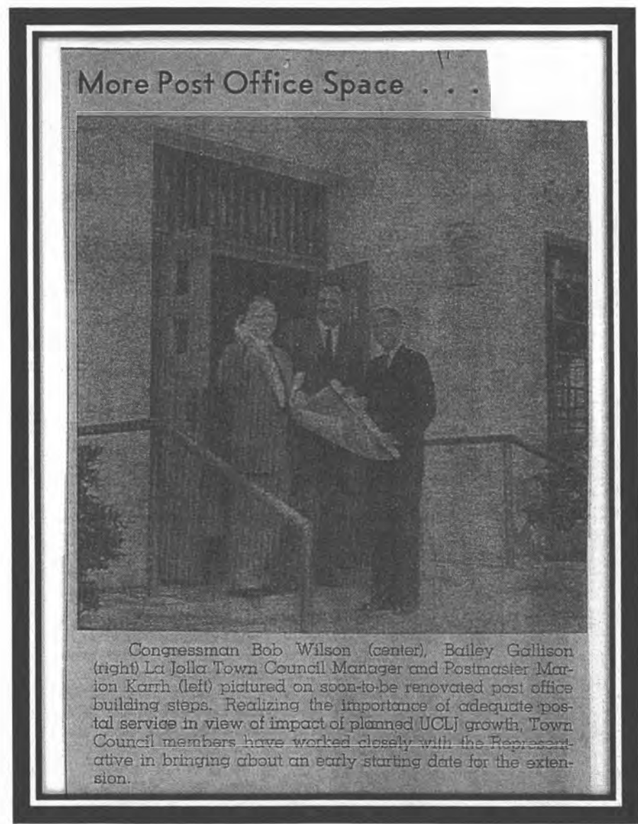
Figure 5. 1935 door and transom prior to remodel. Photo taken November 15, 1959.
