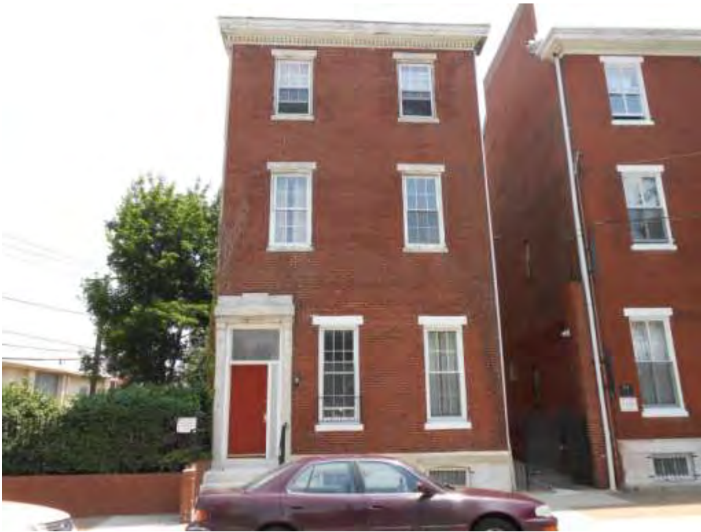
Photograph 23: 721 N. 8 th St. – Single Townhouse – Street Elevation – Facing W (PFA, 2014) PA_Philadelphia_Friends Housing Cooperative_0023
