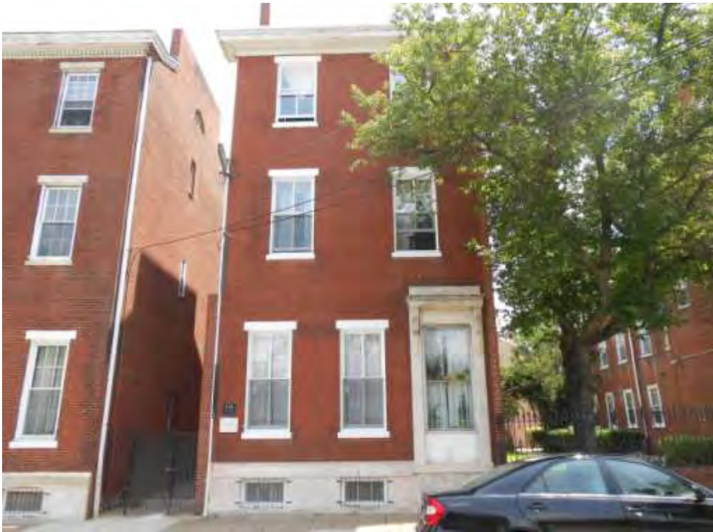
Photograph 19: 719 N. 8 th St. – Single Townhouse – Accessed from Side Alley - Facing E (PFA, 2014) PA_Philadelphia_Friends Housing Cooperative_0019
