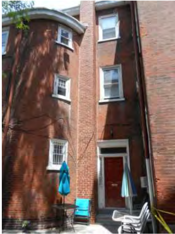
Photograph 29: 712 Franklin St – Access from Courtyard Facing NE (PFA, 2014) PA_Philadelphia_Friends Housing Cooperative_0029
