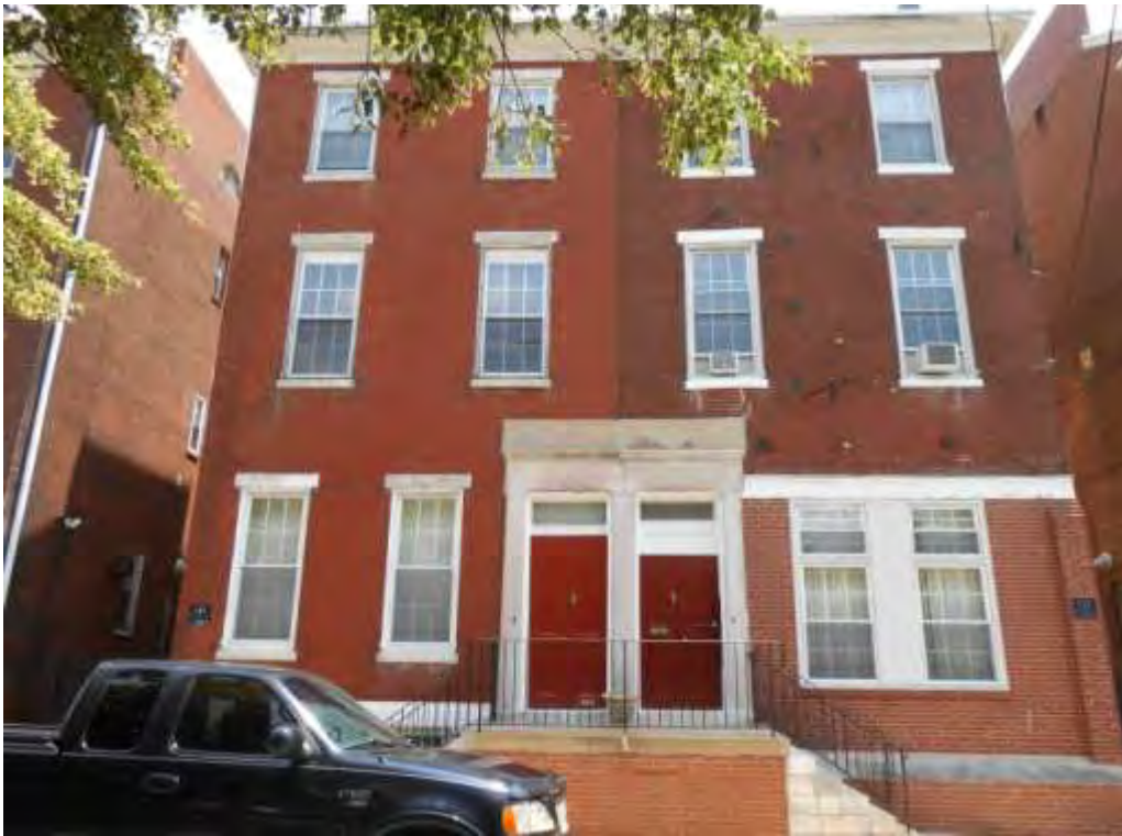
Photograph 15: 705-707 N. 8 th St – Street Elevation - Facing E (PFA, 2014) PA_Philadelphia_Friends Housing Cooperative_0015
