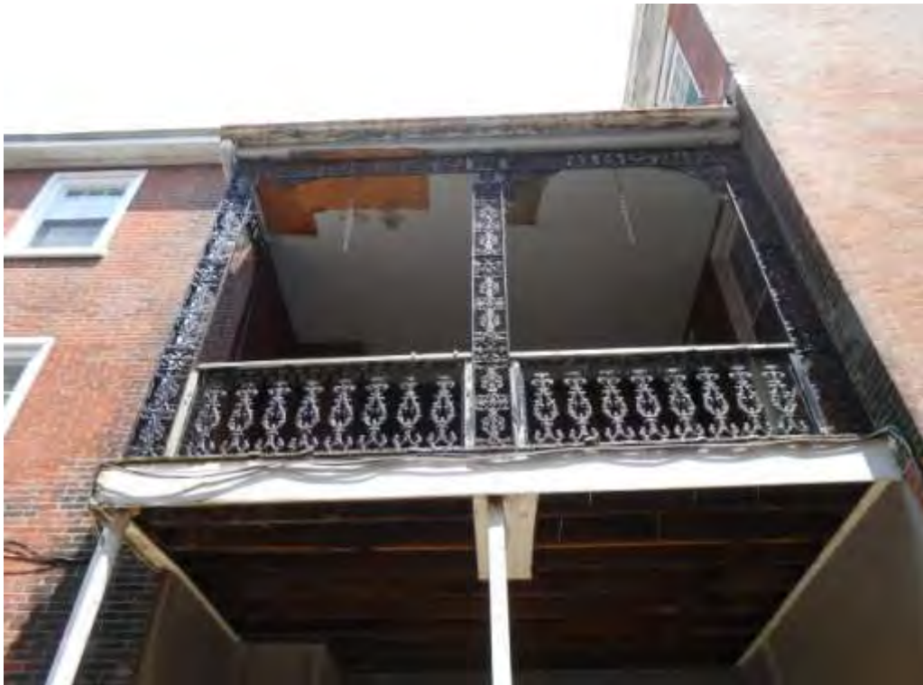
Photograph 31: 708 Franklin St – Balcony – South Elevation - Facing N (PFA, 2014) PA_Philadelphia_Friends Housing Cooperative_0031
