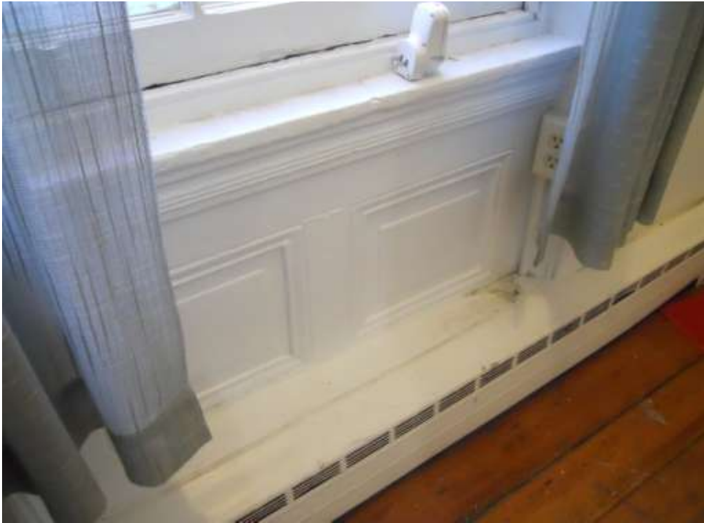
Photograph FHC 39: Apartment Unit – Extant 19 th Century Finishes, Typical (PFA, 2014) PA_Philadelphia_Friends Housing Cooperative_0039
