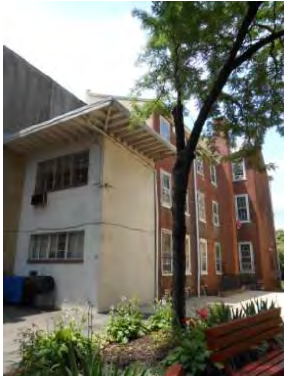
Photograph 34: Courtyard Elevations - 703 N. 8 th St. - Facing W (PFA, 2014) PA_Philadelphia_Friends Housing Cooperative_0034
