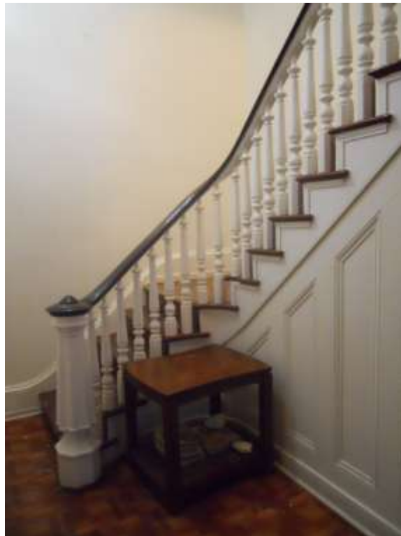
Photograph 40: “Piazza” Stair – 1 st Floor – Typical (PFA, 2014) PA_Philadelphia_Friends Housing Cooperative_0040
