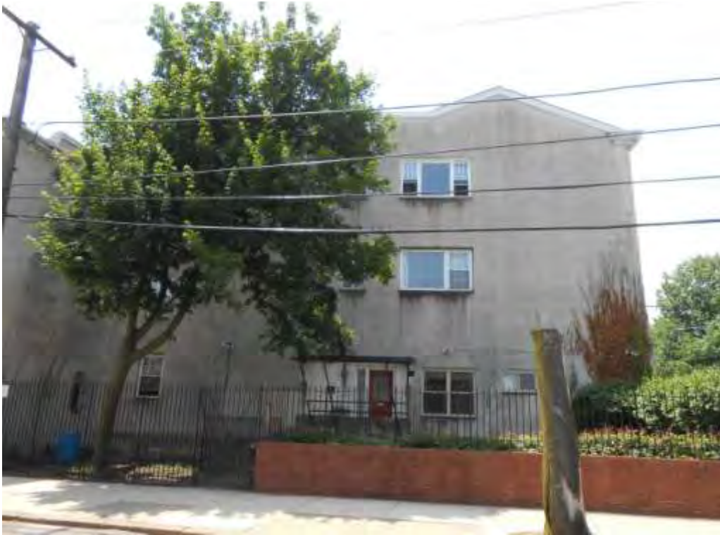
Photograph 25: 721 N. 8 th St. – Single Townhouse – Brown Street Elevation – Facing S (PFA, 2014) PA_Philadelphia_Friends Housing Cooperative_0025
