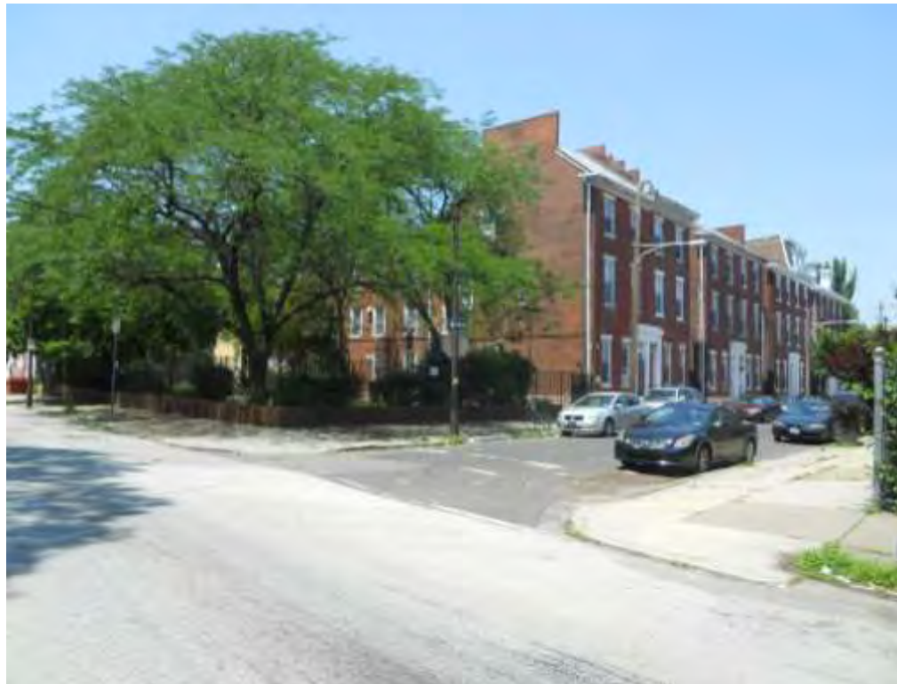
Photograph 04: FHC – Corner of Fairmount Avenue and Franklin Street – Facing NW (PFA, 2014) PA_Philadelphia_Friends Housing Cooperative_0004
