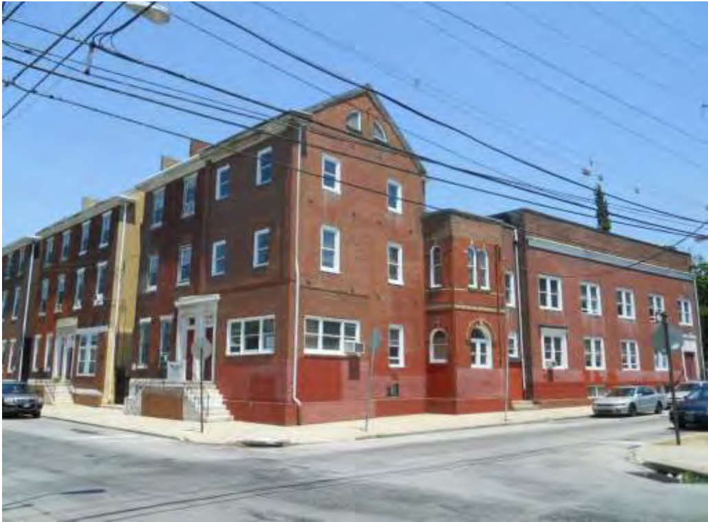
Photograph 01: Corner of Fairmount Avenue and N. 8 th Street – Facing NE (PFA, 2014) PA_Philadelphia_Friends Housing Cooperative_0001
