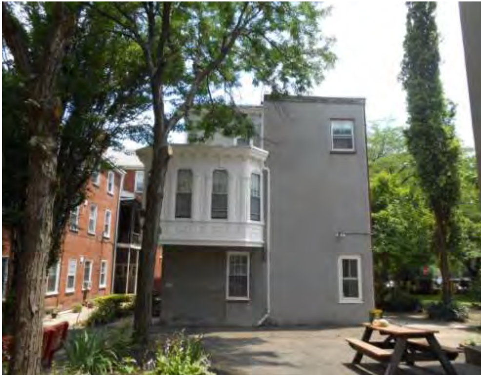
Photograph 12: 704-706 Franklin St – Courtyard Elevation - Facing E (PFA, 2014) PA_Philadelphia_Friends Housing Cooperative_0012
