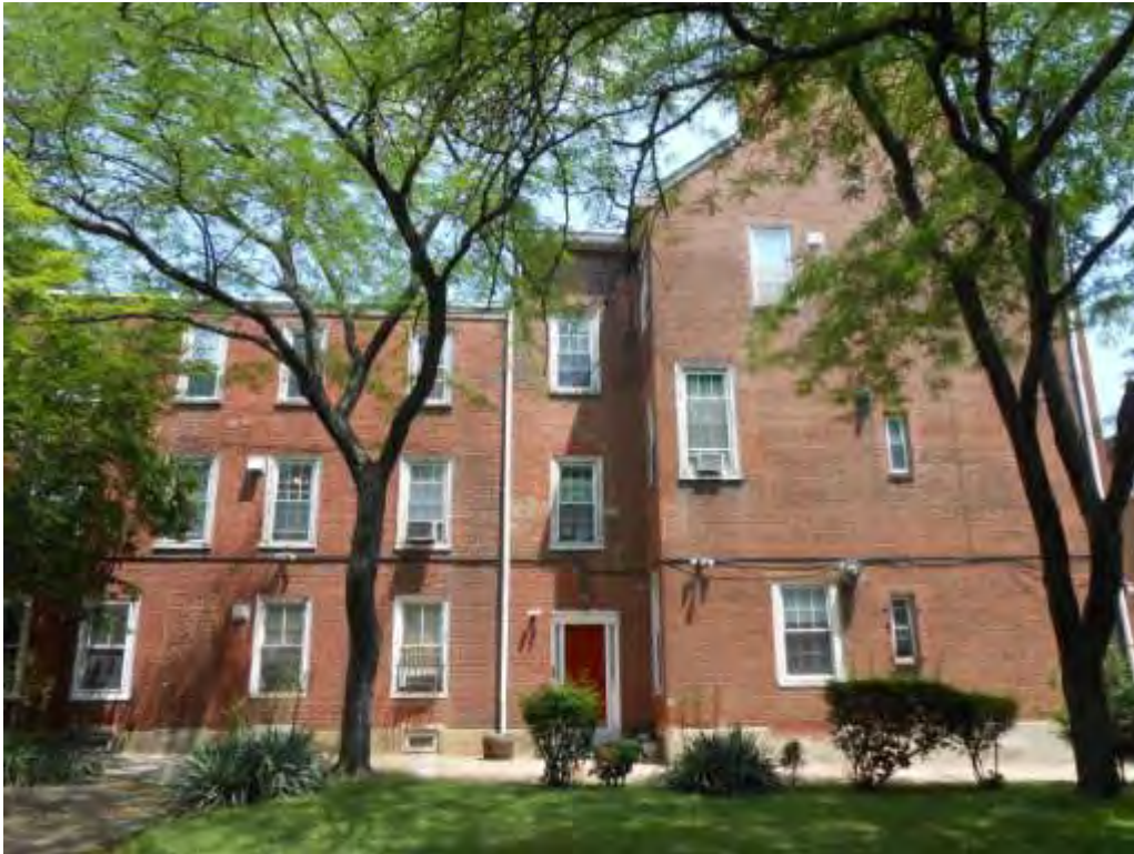
Photograph 13: 704-706 Franklin St – Side Elevation - Facing N (PFA, 2014) PA_Philadelphia_Friends Housing Cooperative_0013
