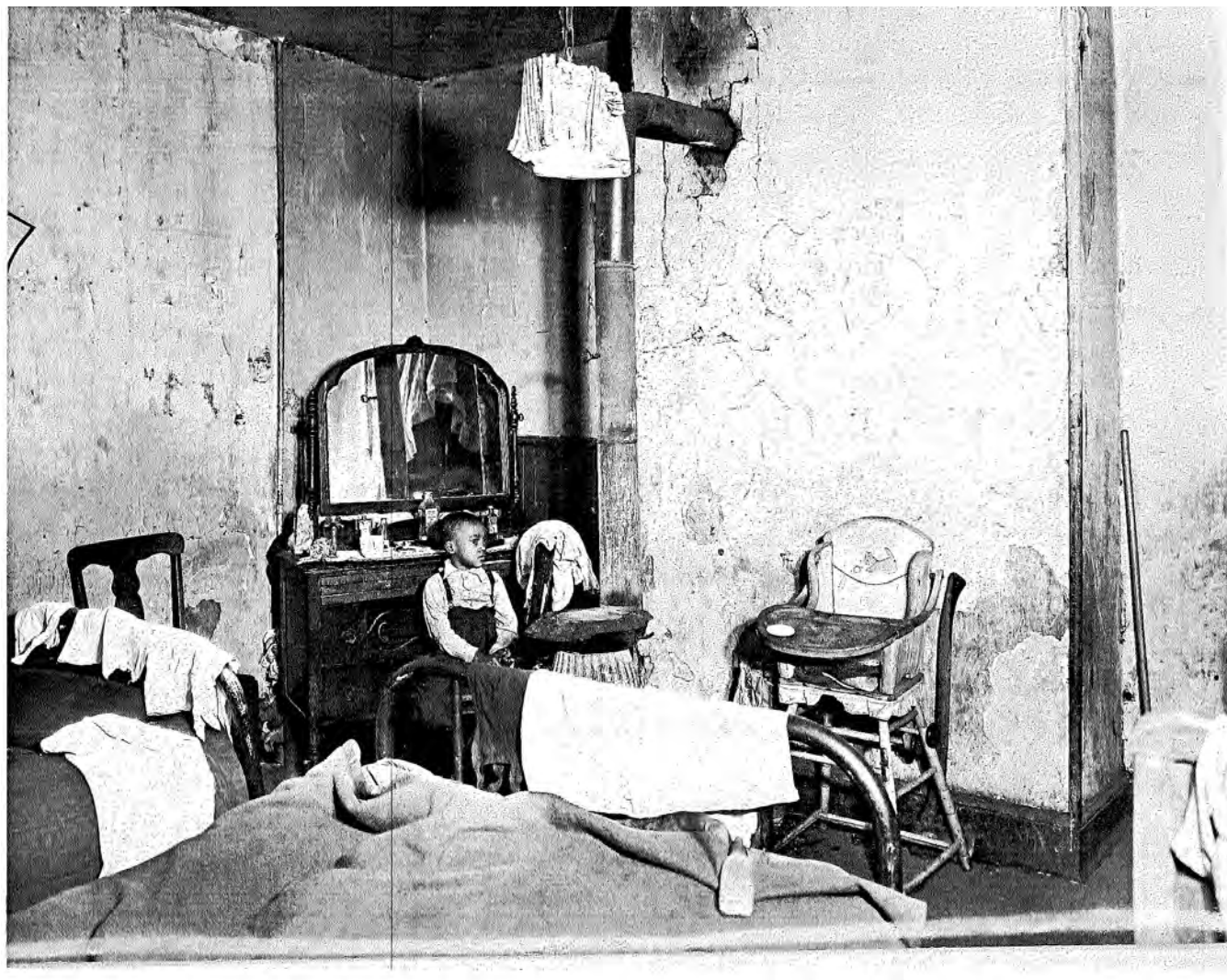
Figure 11: Existing Conditions Pre-Rehabilitation c. 1940s (AFSC Archives)
