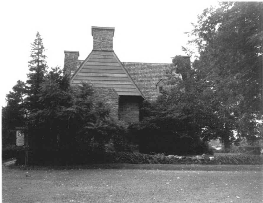
Henry Whitfield House, 1639 East end of rear wing (left), and east (rear) elevation of main house, right.
