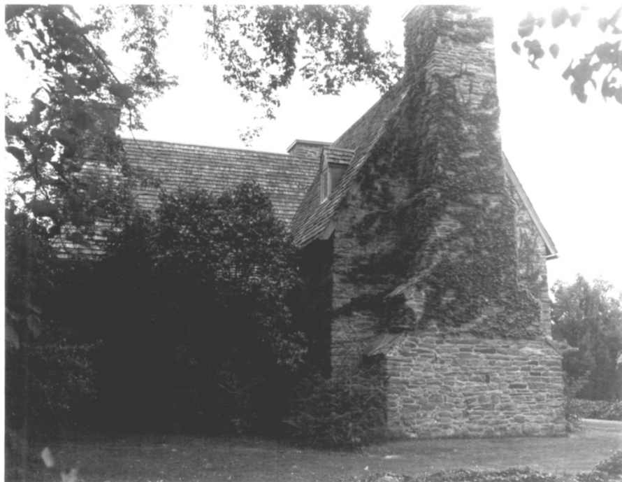
Henry Whitfield House, 1639 North end of main house, right and North side of rear wing, left
