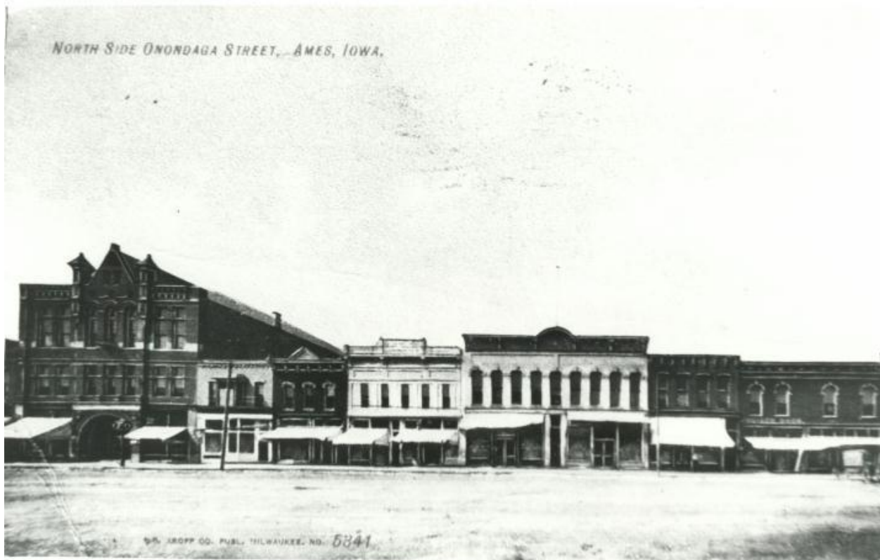
Figure 2. Showing the north side of Onondaga Street sometime before 1910. The Odd Fellows Building is the tall building on the very left. The Tilden Block buildings in right-center were built in 1883. (Farwell T. Brown Photographic Library 10.42.1-2)
