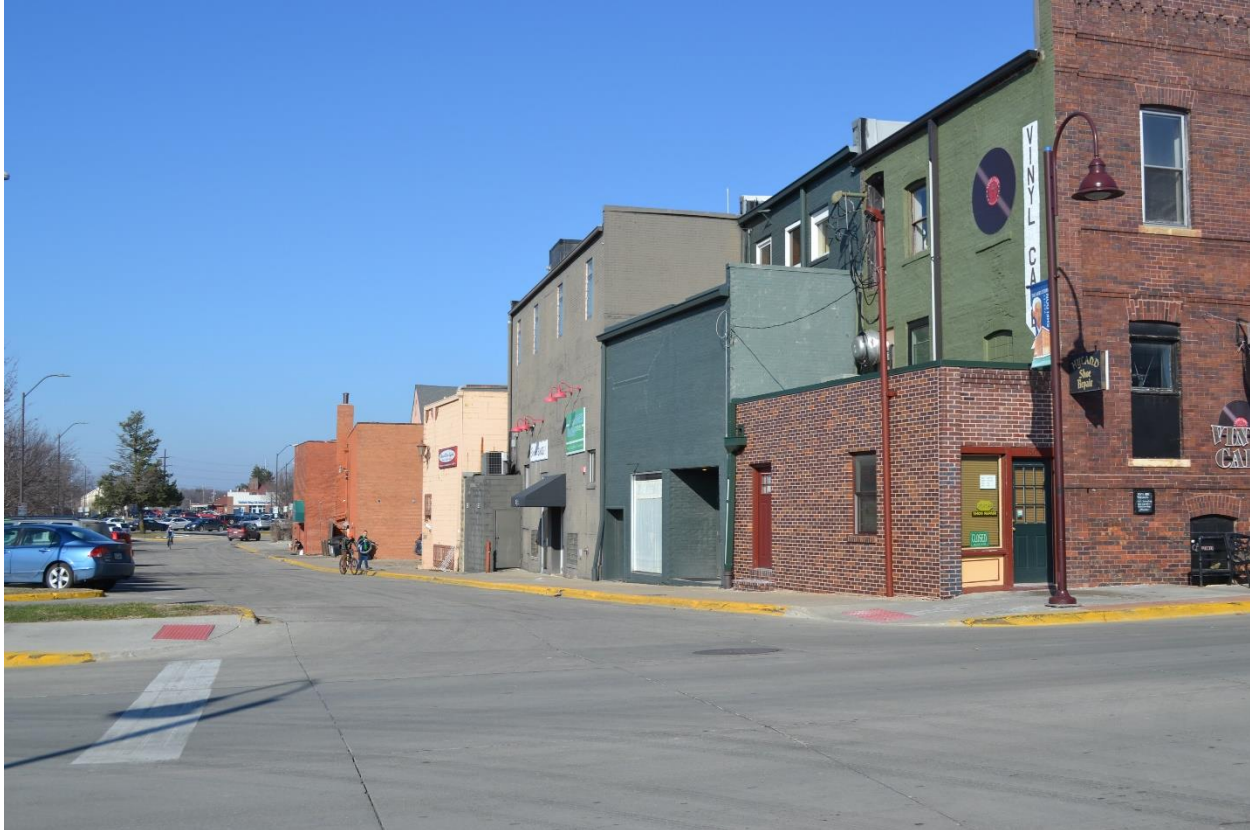
Figure S7. 2018 Photo looking northwest across Kellogg from the rear of south main street buildings. This view shows how removal of the railroad tracks allowed for a vital public parking lot which sparked an increase of commercial activity and modest rear “facelift” remodels on this side.
