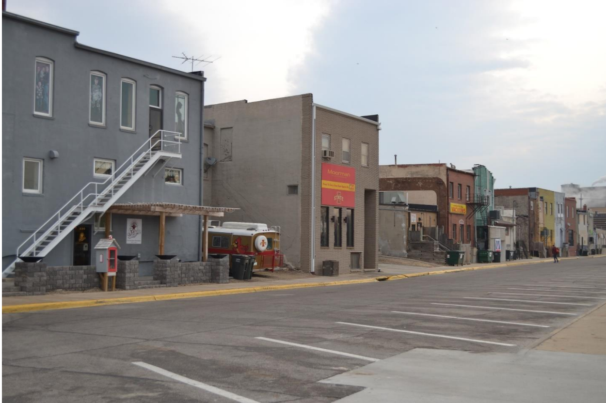
Figure S9. 2018 Photograph looking northeast on the rear of south Main St. buildings. This picture captures the adaptations which businesses have made to accommodate the rear traffic to their businesses (including entranceways and signage). Essentially, the 1960s change to move the rail tracks opened a second storefront for the businesses along the south of Main St.
