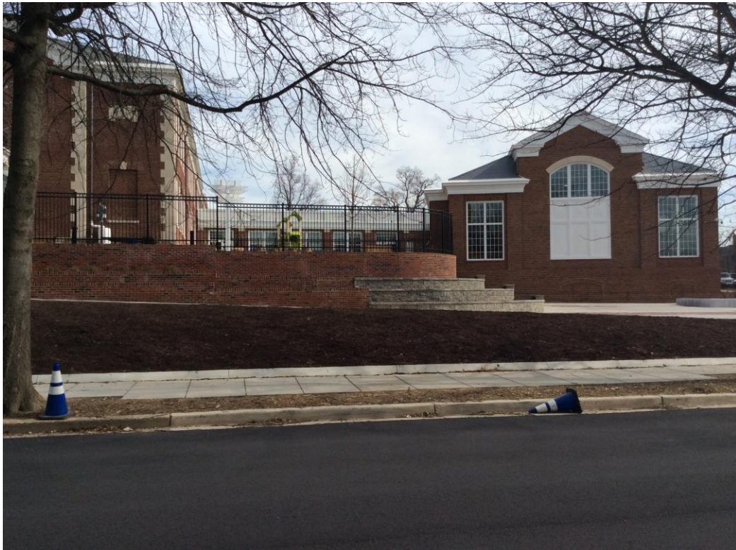
Photo 14: Gymnasium Wing (2016), Looking East Hartman-Cox, February 2013
