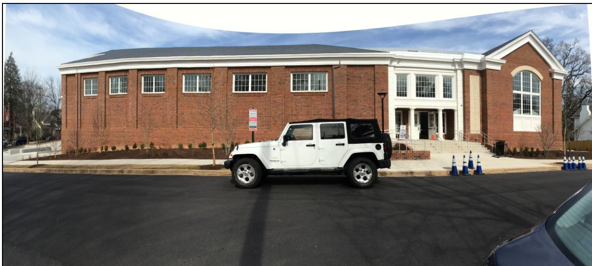
Photo 18: Gymnasium Wing (2016), Looking North Hartman-Cox, February 2017
