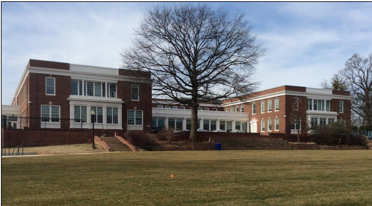
Photo 16: East Wing Additions with Central Pavilion, Looking Northwest Hartman-Cox, February 2017
