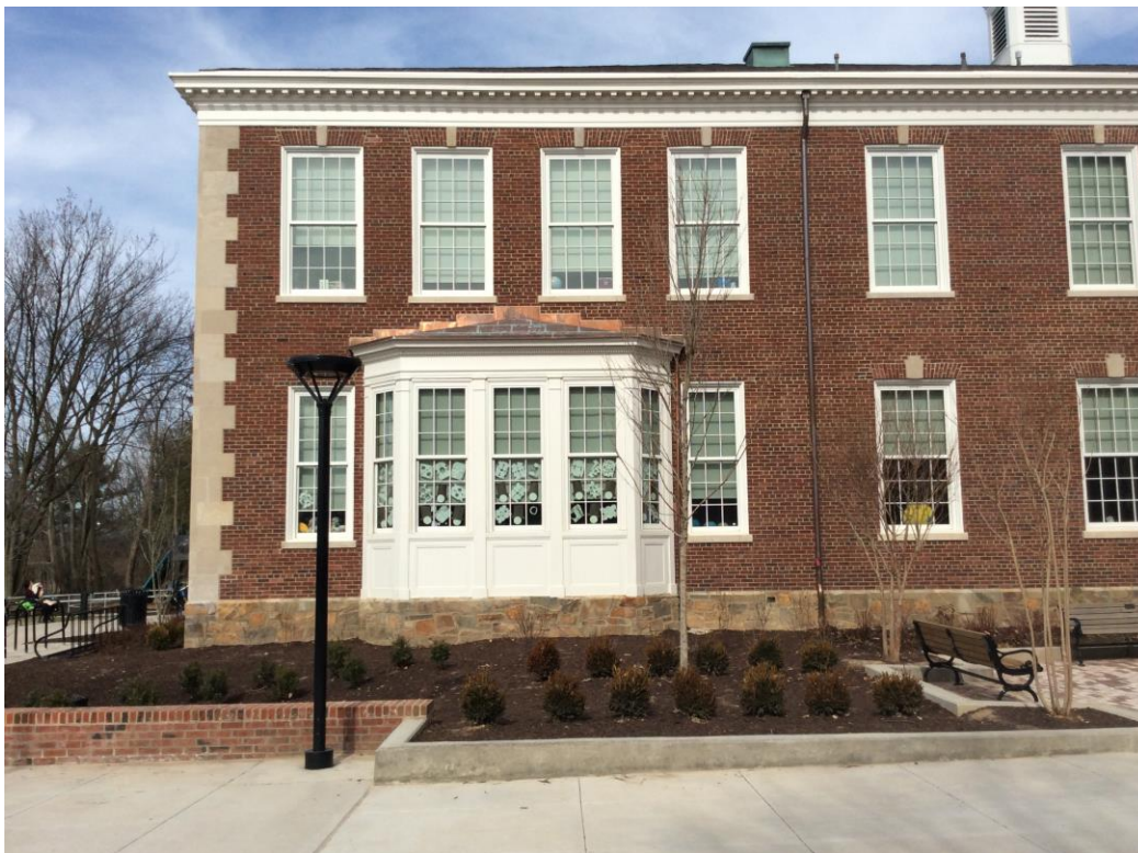
Photo 12: Bay Window on North Wing, Looking South Hartman-Cox, February 2017
