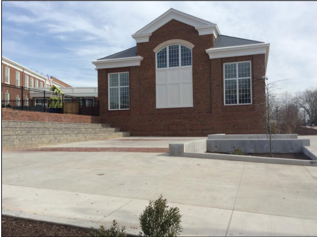
Photo 17: Gymnasium Wing (2016), Looking East Hartman-Cox, February 2017
