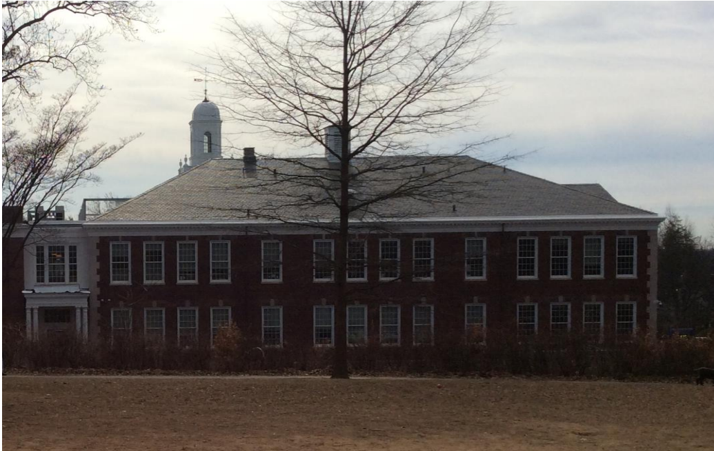
Photo 11: North Wing, North Elevation, Looking Southeast Hartman-Cox, February 2017
