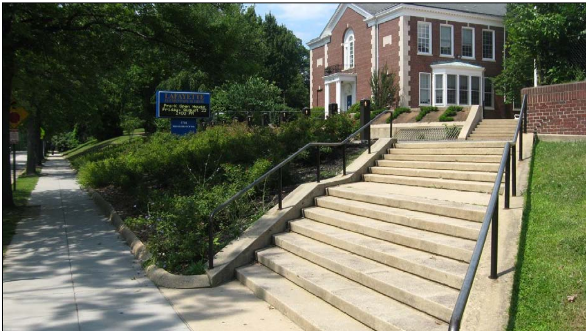
Photo 2: Front Access along Broad Branch Road, Looking North EHT Traceries, July 2014
