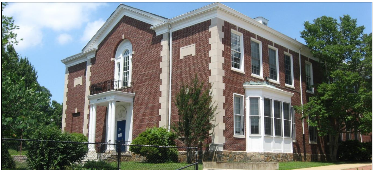
Photo 8: North Wing, West and South Elevations, Looking Northeast EHT Tracerics, Inc., June 2014
