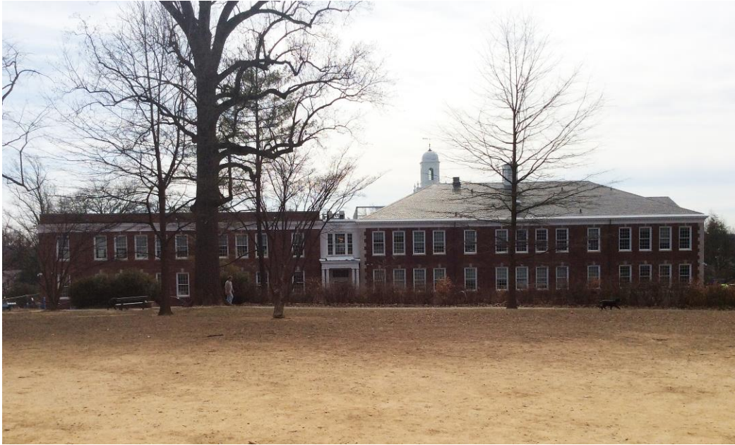
Photo 13: West Wing and Addition, Looking South Hartman-Cox, February 2017
