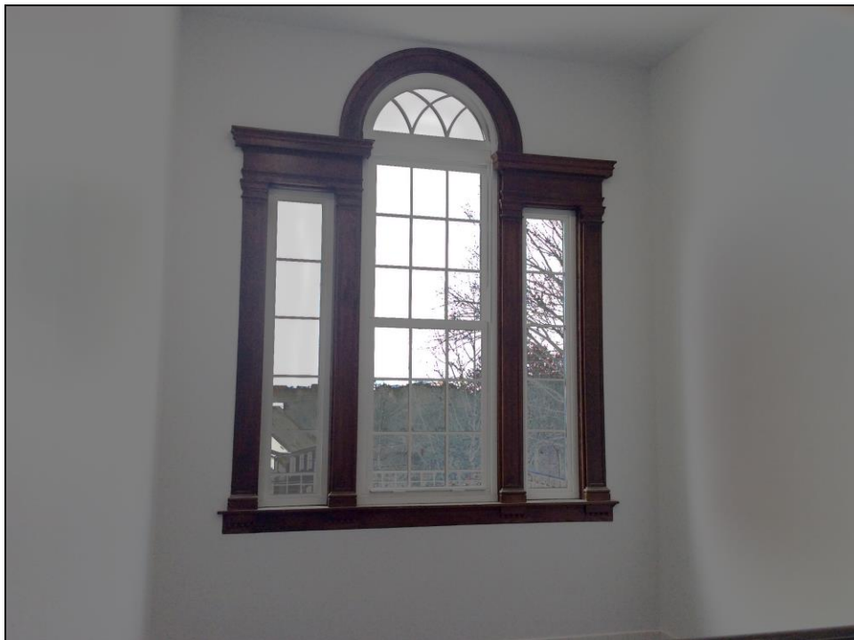
Photo 20: Interior of Palladian Window, Looking West Hartman-Cox, February 2017
