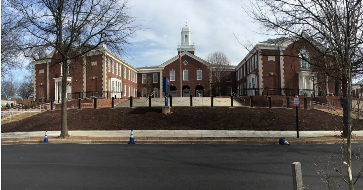
Photo 1: Lafayette Elementary School, West Elevation, Looking East Hartman-Cox, February 2017
