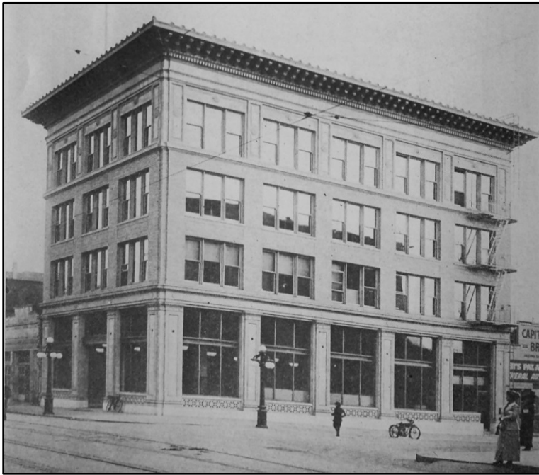
Figure 3, Great Western Power/ PG&E Building, Sacramento, E.C. Hemmings
