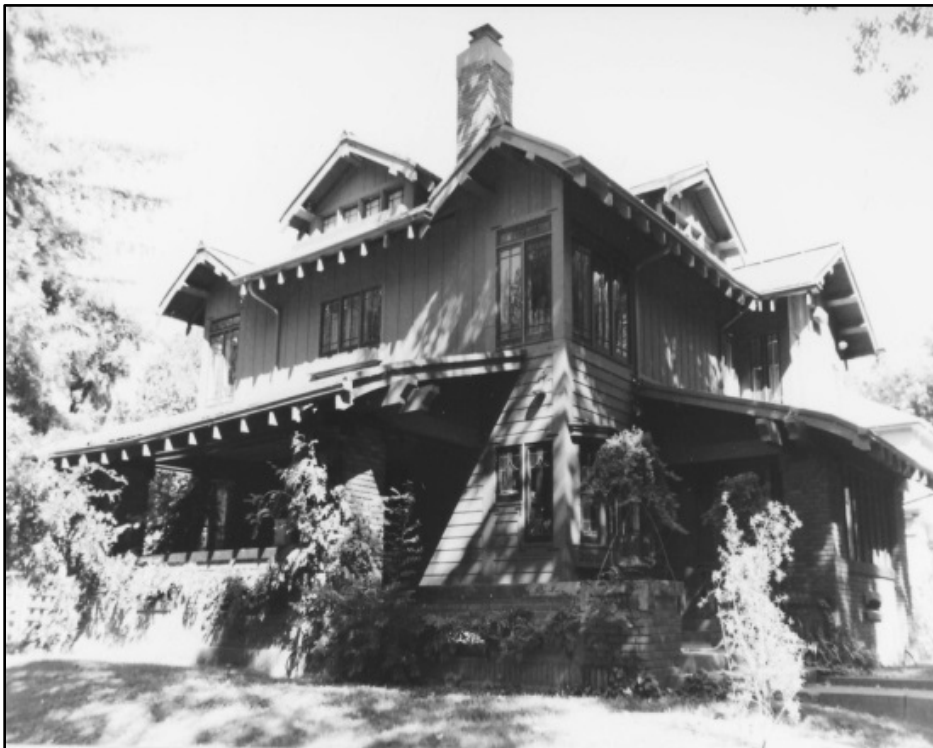
Figure 9 The Cranston-Geary House, Sacramento, listed in the National Register of Historic Places
