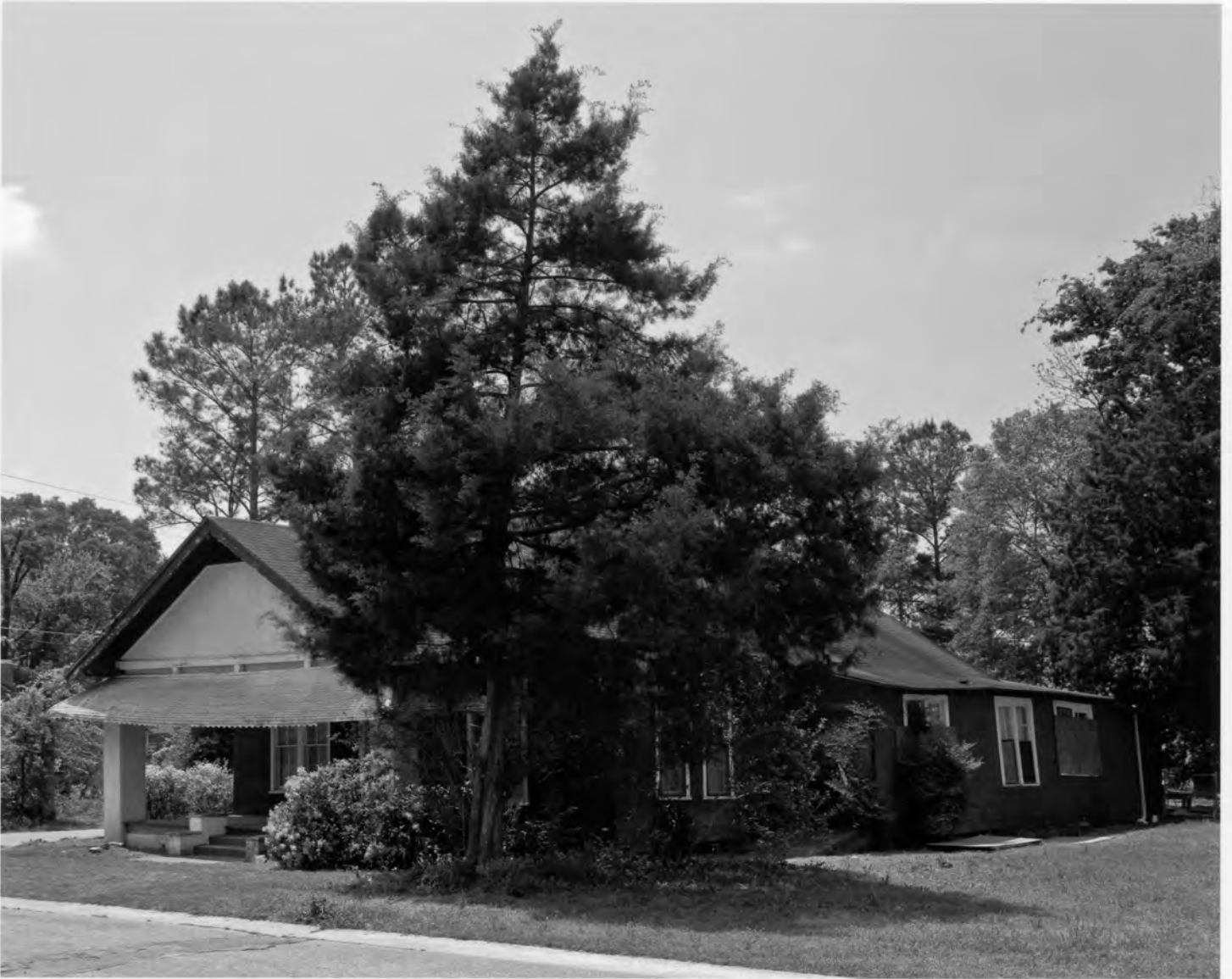
Georgia Williams Nursing Home Mitchell County, Georgia Photograph 6 of 22
