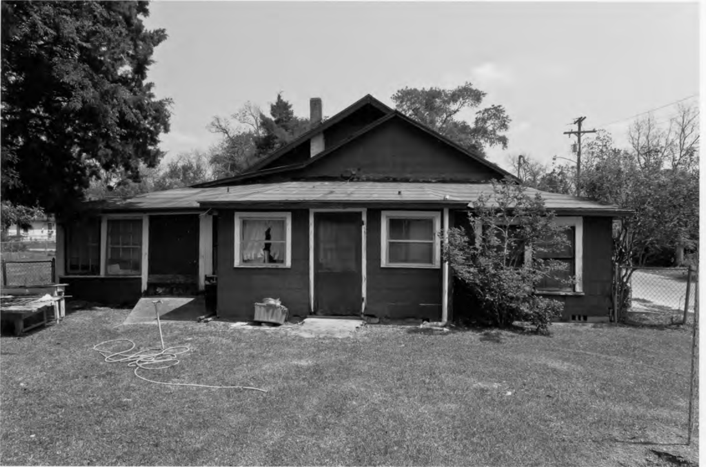
Georgia Williams Nursing Home Mitchell County, Georgia Photograph 4 of 22
