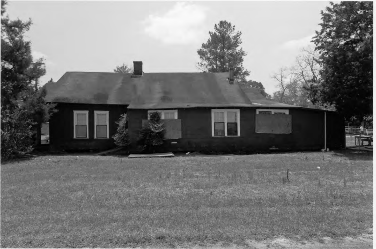
Georgia Williams Nursing Home Mitchell County, Georgia Photograph 7 of 22
