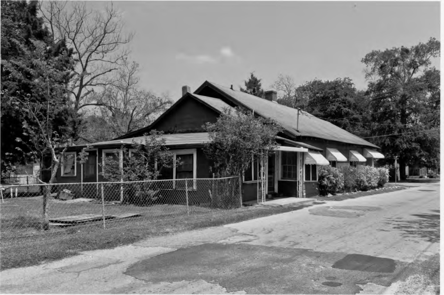
Georgia Williams Nursing Home Mitchell County, Georgia Photograph 3 of 22
