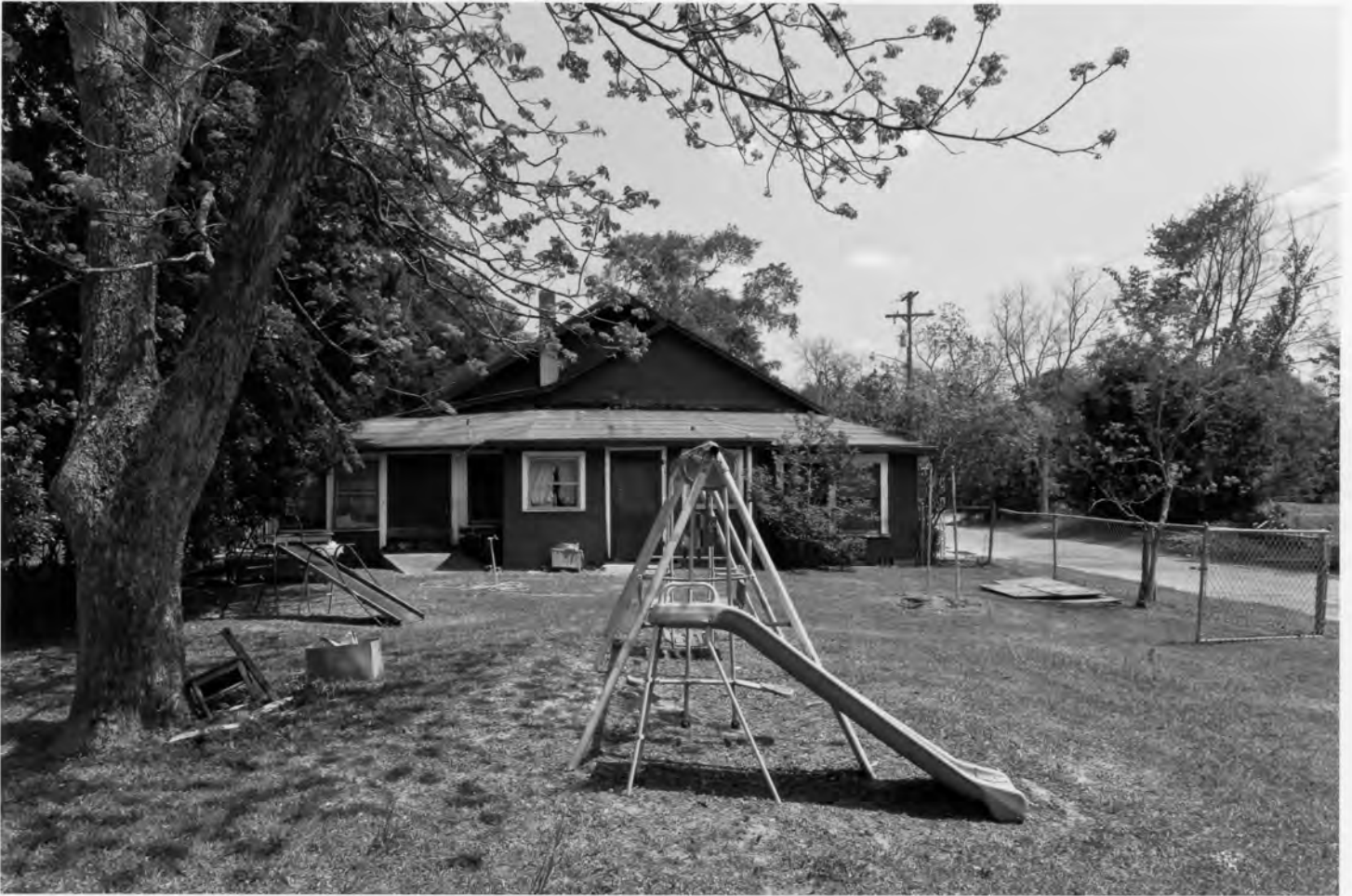
Georgia Williams Nursing Home Mitchell County, Georgia Photograph 5 of 22
