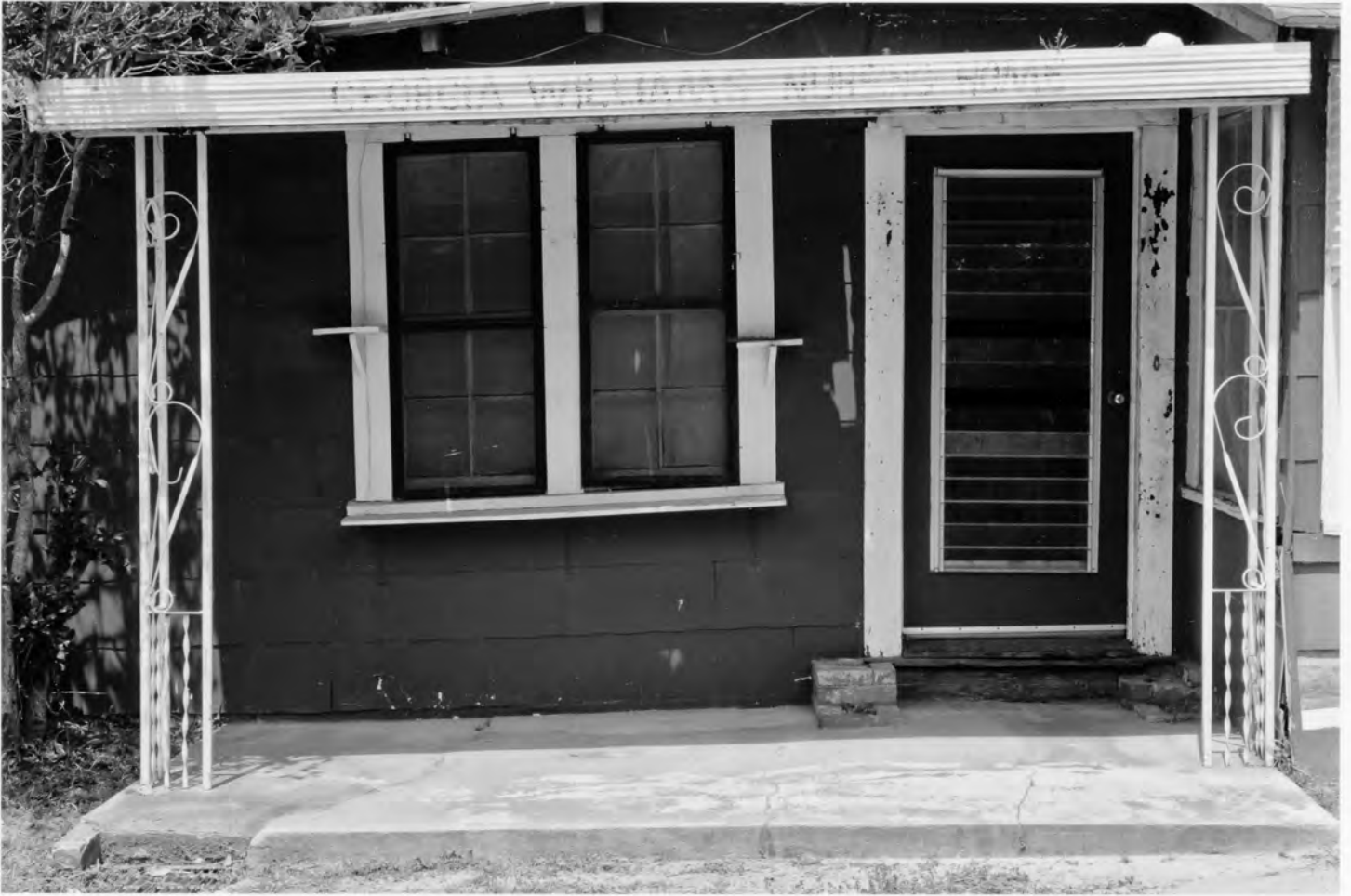
Georgia Williams Nursing Home Mitchell County, Georgia Photograph 9 of 22
