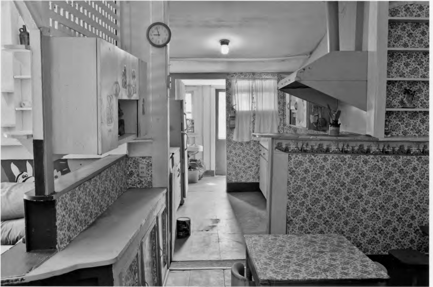
Georgia Williams Nursing Home Mitchell County, Georgia Photograph 20 of 22
