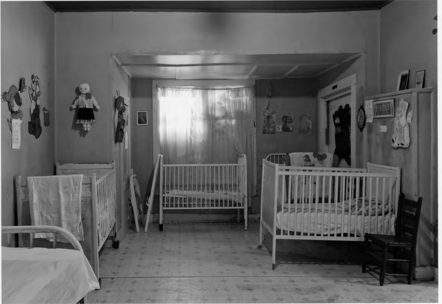
Georgia Williams Nursing Home Mitchell County, Georgia Photograph 14 of 22
