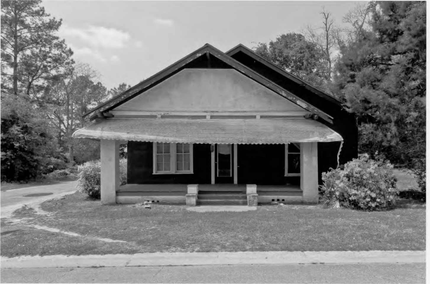
Georgia Williams Nursing Home Mitchell County, Georgia Photograph 1 of 22
