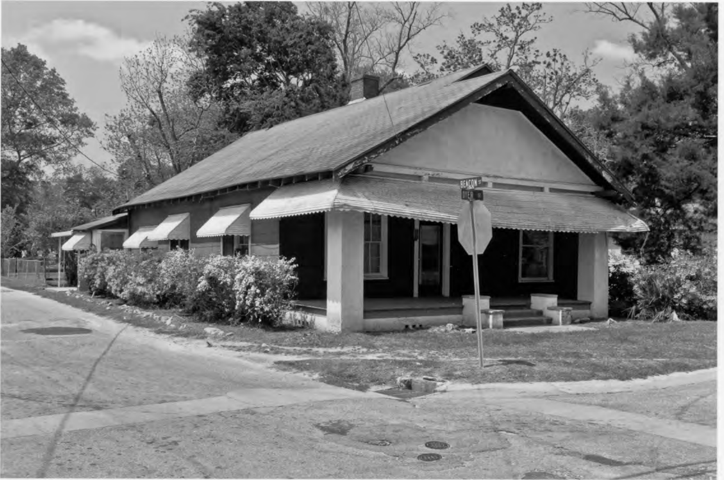
Georgia Williams Nursing Home Mitchell County, Georgia Photograph 2 of 22
