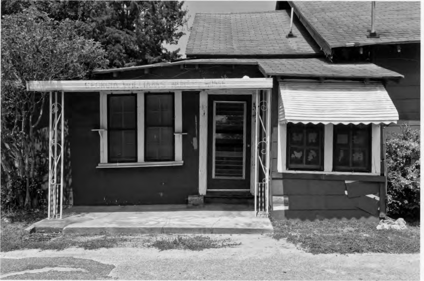
Georgia Williams Nursing Home Mitchell County, Georgia Photograph 8 of 22
