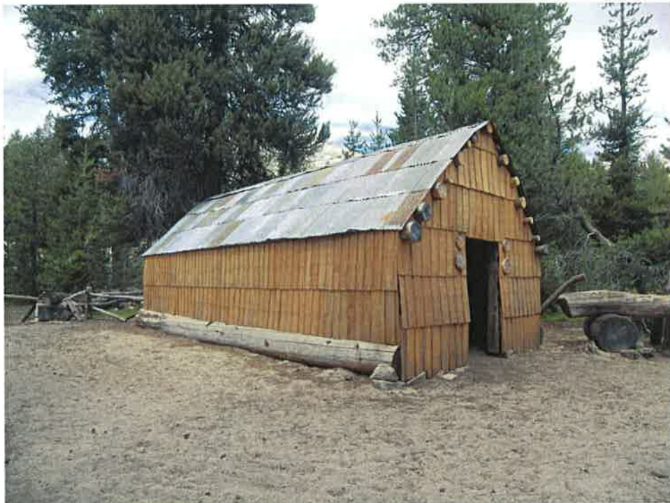
8 of 20. Barn; Contributing. Southeastern elevation.
