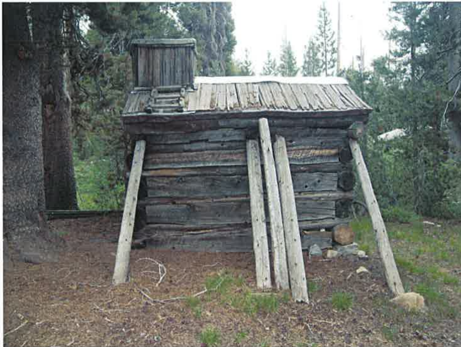
14 of 20. Ranger Showerhouse; Contributing. Eastern elevation.
