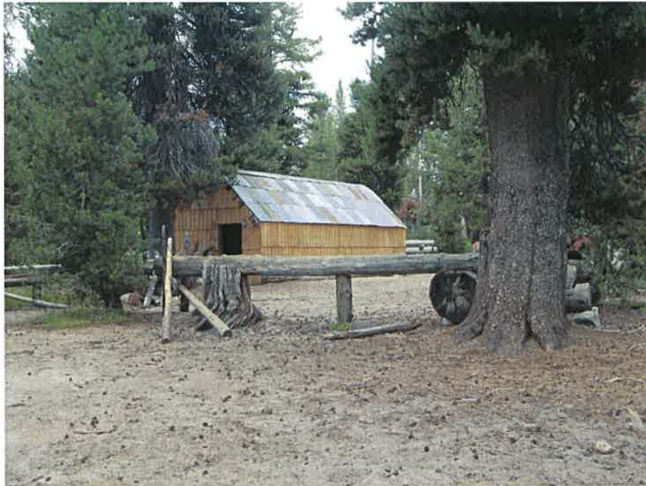
15 of 20. Barn and Corral; Contributing. Eastern elevation.
