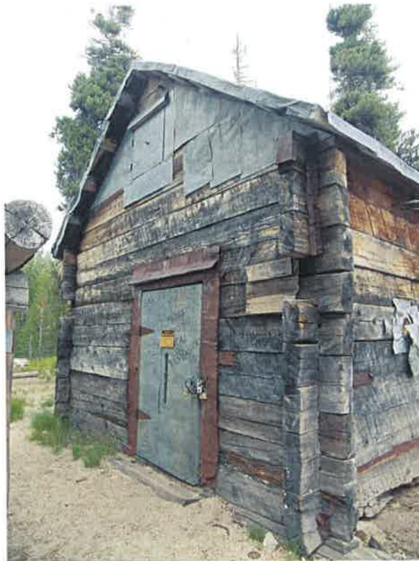
4 of 20. New Cabin; Contributing. Southeastern elevation.
