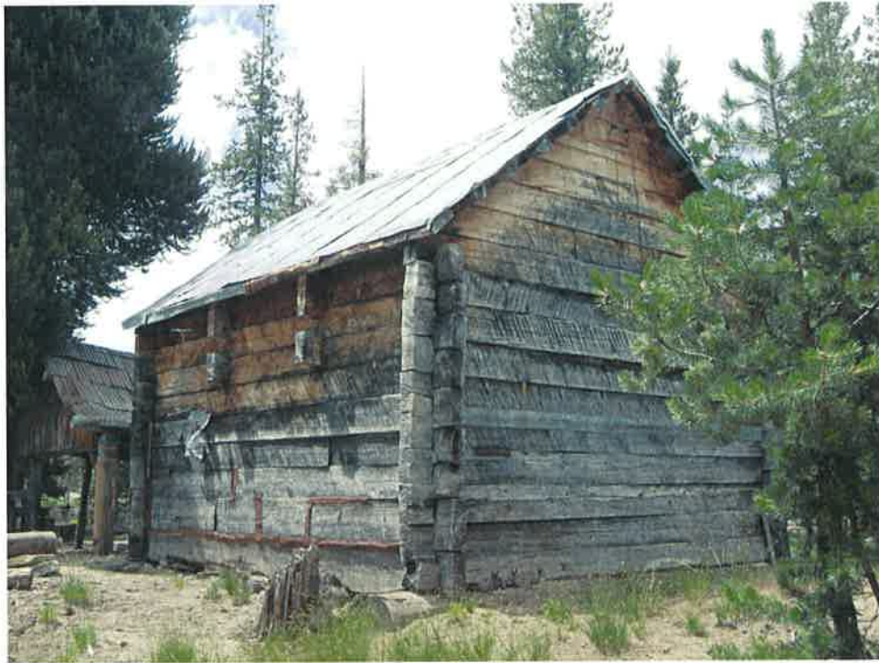
5 of 20. New Cabin; Contributing. Northeastern elevation.
