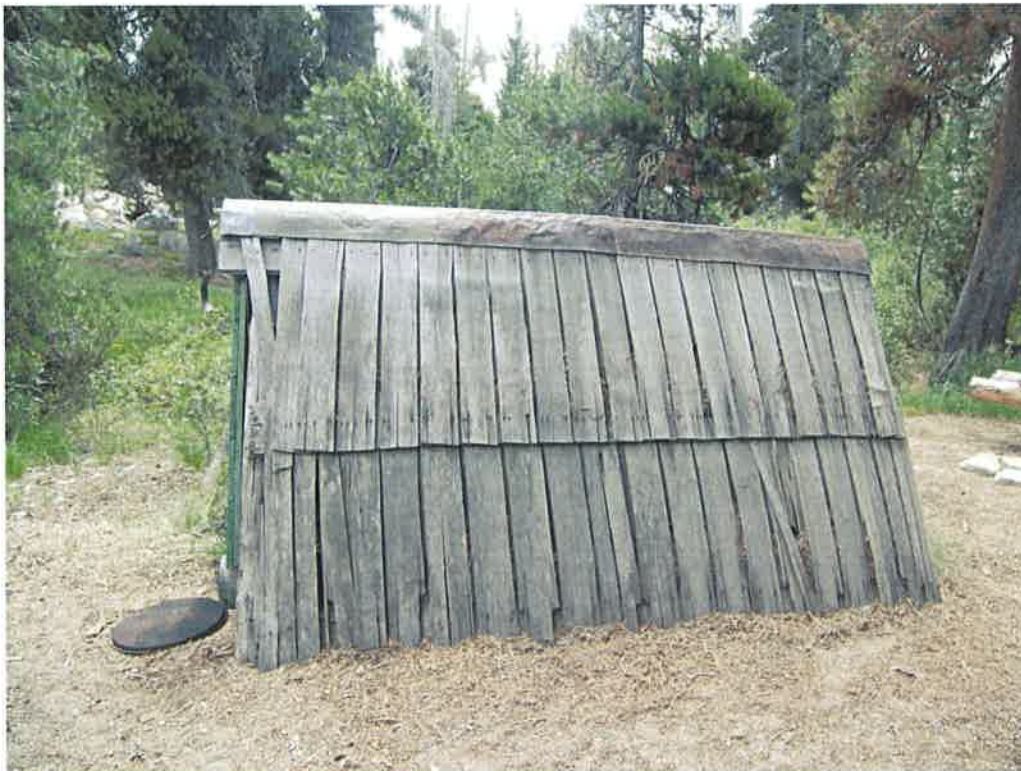
20 of 20. Bunkhouse roof; Non-contributing. Eastern elevation.
