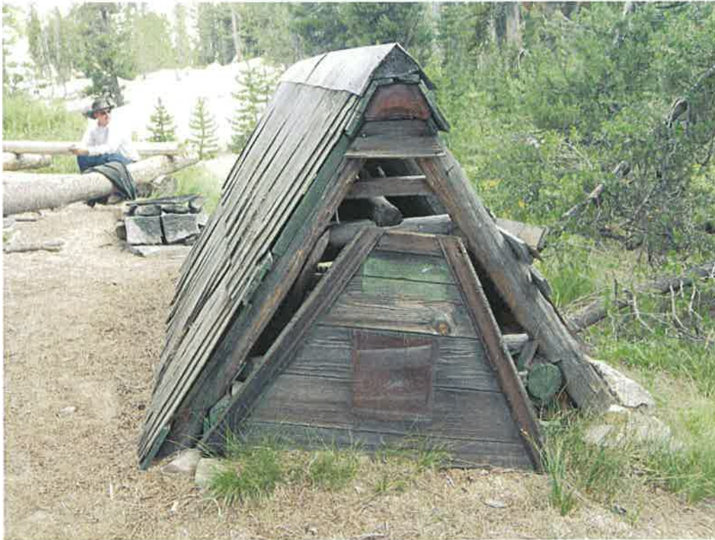
19 of 22. Bunkhouse roof; Non-contributing. Southern elevation.
