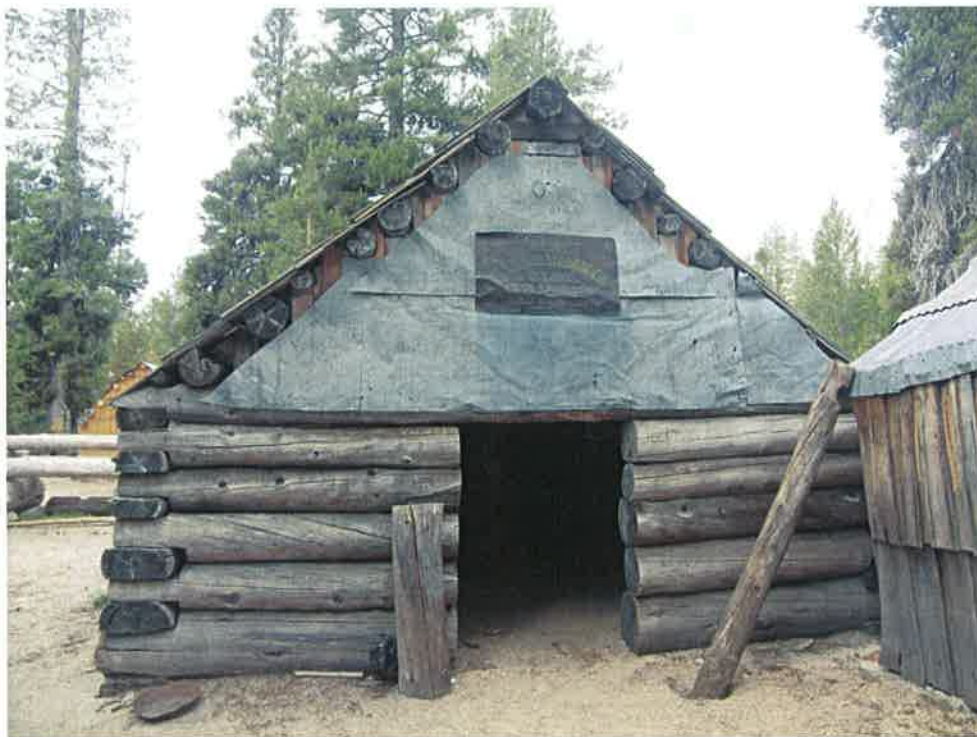
2 of 20. Old Cabin; Contributing. Northeastern elevation.
