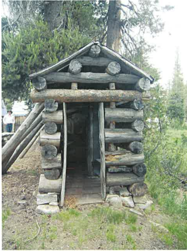
13 of 20. Showerhouse; Contributing. Southern elevation.
