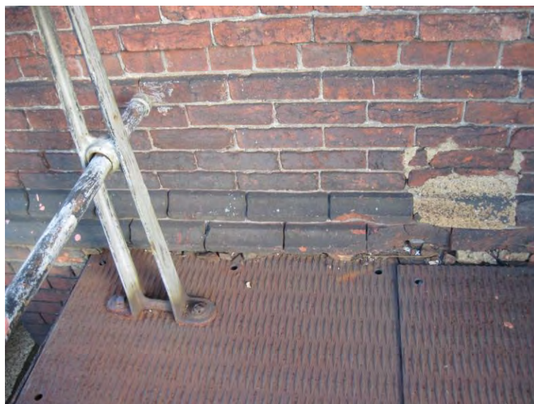
Figure 4. Water table consisting of two rows of red concave plinth bricks
