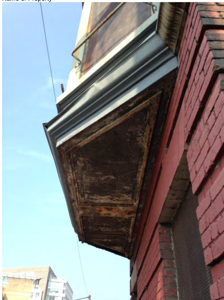
Figure 7. Bay Window Soffit, South Elevation
