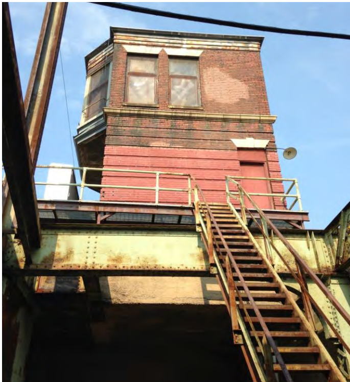
Figure 3. Steel staircase attached to steel platform on the East Elevation
